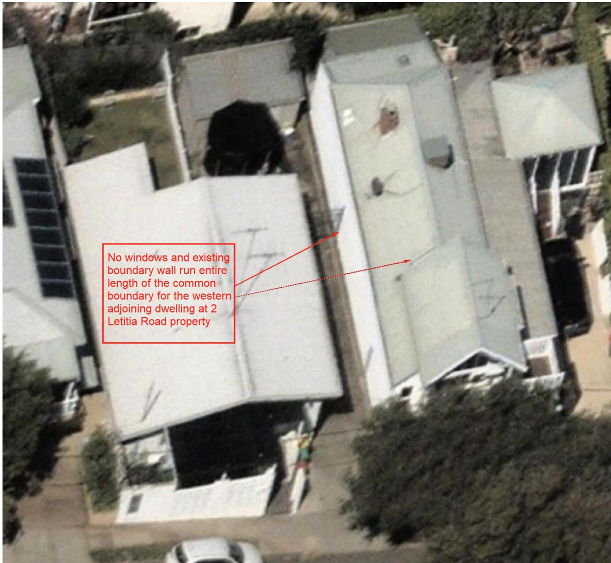
Figure 6 - Showing subject site to the left and western adjoining property (No.2 Letitia Road) and its existing eastern elevation
