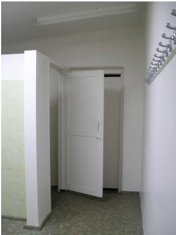
Figure 64 View of toilet and shower rooms. Hocking Planning and Architecture, August 2009.
