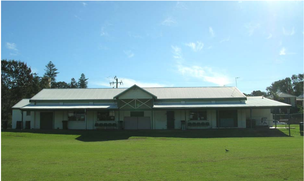
Figure 68 View of the single storey hall –‘Stan Whipp Hall’ - from the oval. Hocking Planning and Architecture, August 2009.
