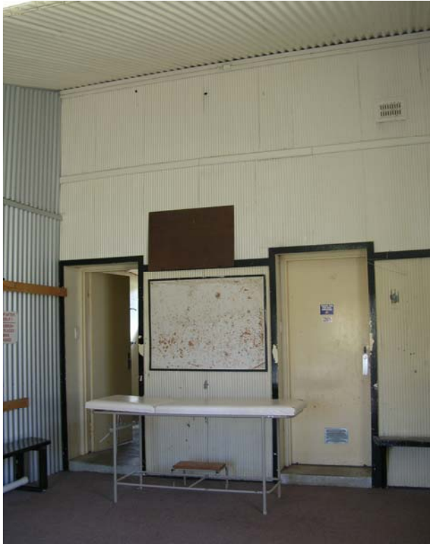
Figure 63 Interior view of the northern end change room. All original wall lining on three elevations, apart from the western wall (as seen in image), have been replaced with 'Zincalume Custom Orb' wall lining. Hocking Planning and Architecture, August 2009.
