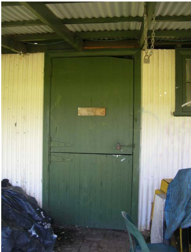
Figure 90 Extant timber matchboard door and signage identifying the former stables. Hocking Planning and Architecture, August 2009
