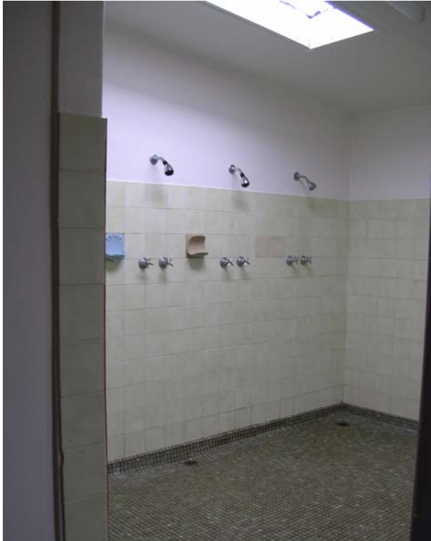
Figure 65 View of shower area. Hocking Planning and Architecture, August 2009.
