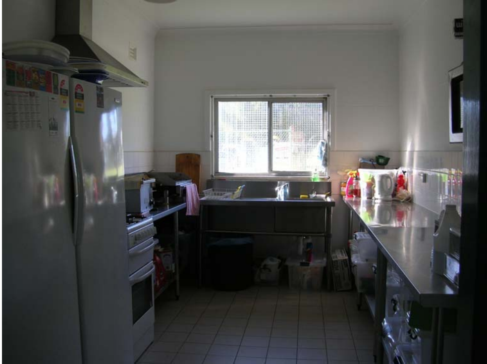
Figure 84 View of kitchen. Hocking Planning and Architecture, August 2009
