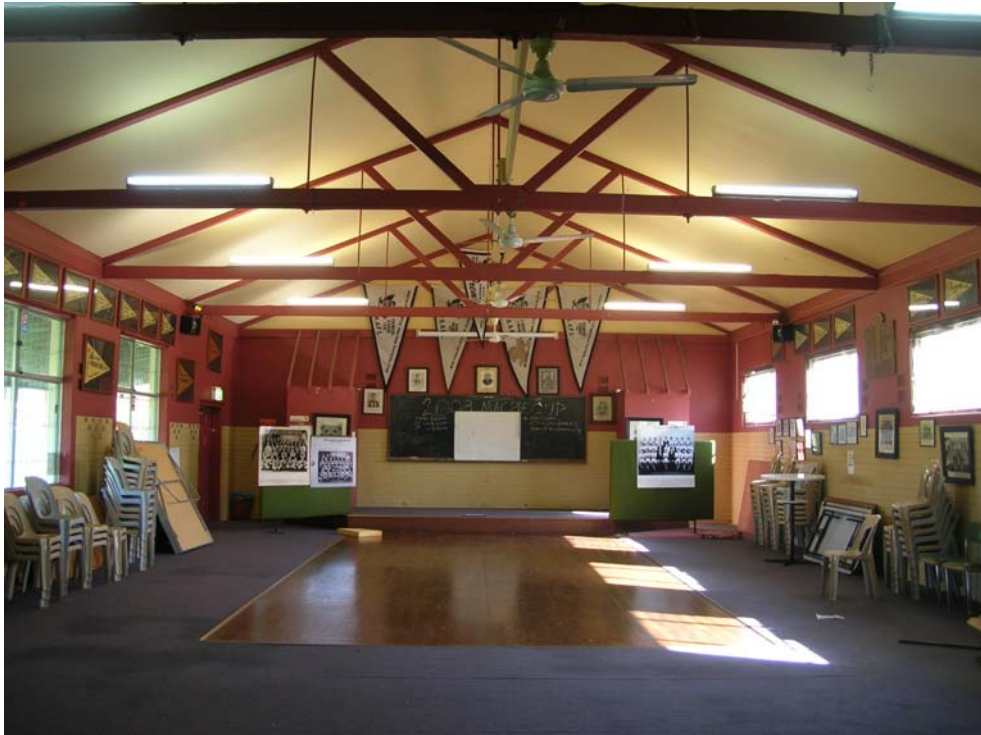
Figure 78 Interior view of the hall, looking west. The toilet annexe is located beyond the stage. Hocking Planning and Architecture, August 2009.
