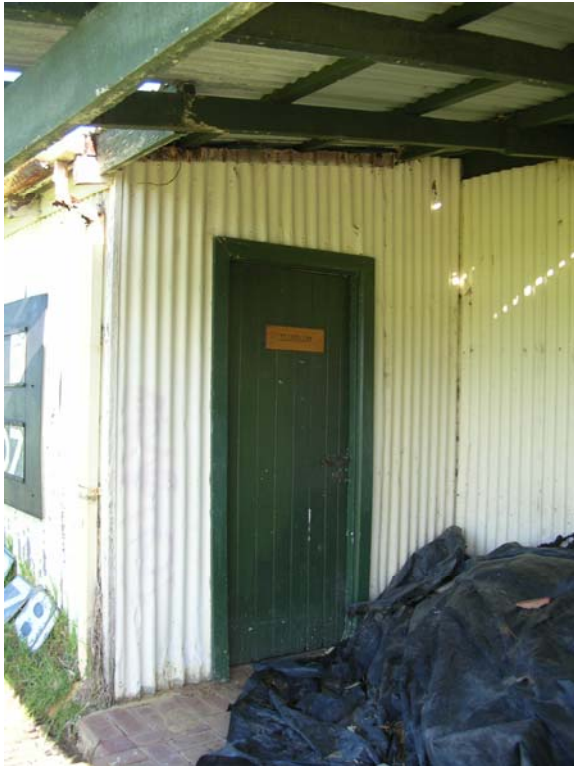
Figure 91 Extant timber matchboard door. Hocking Planning and Architecture, August 2009
