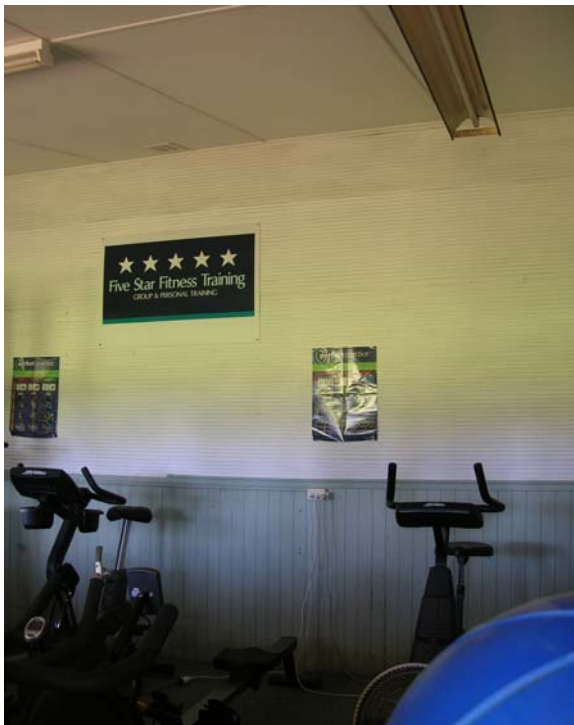
Figure 92 Interior view of the south-western room, with timber wainscoting and corrugated sheet metal cladding above dado. Hocking Planning and Architecture, August 2009
