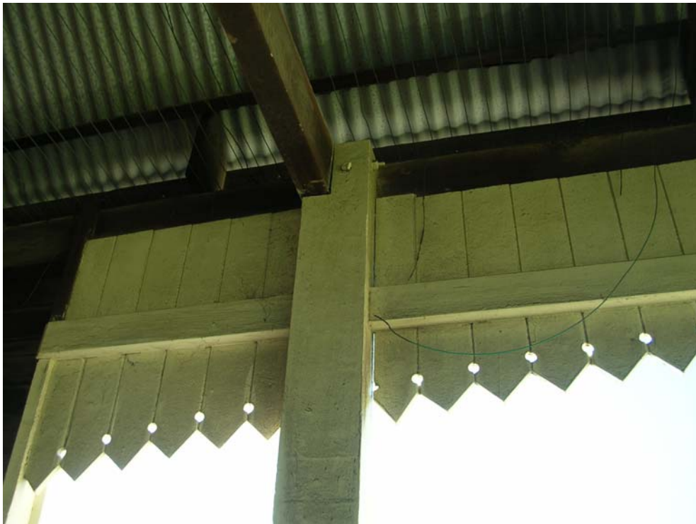
Figure 53 View detail of timber fascia boards with simple chevron and circle cut-out pattern on the, evident on the north and south elevations of the pavilion. Hocking Planning and Architecture, August 2009.
