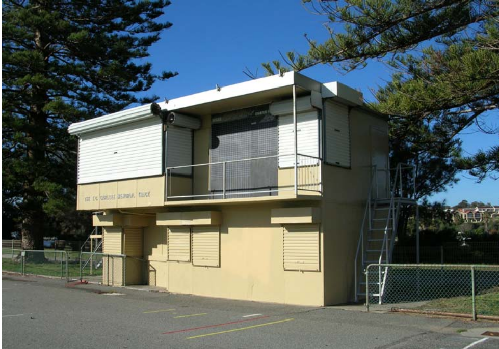
Figure 93 Exterior view of the W.A.F.B. timing stand. Hocking Planning and Architecture, August 2009
