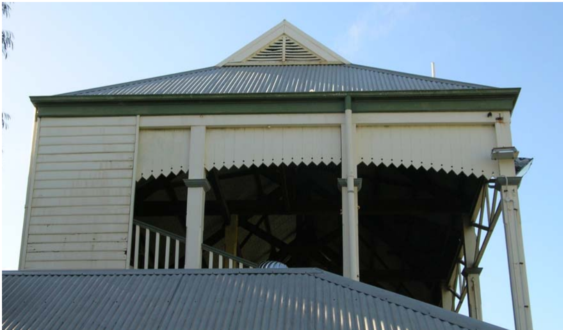
Figure 51 Timber detailing on the east elevation of the grandstand structure. Corrugated sheet metal roof seen below the pavilion is the southern addition, accommodating an office and storage room. Hocking Planning and Architecture, August 2009.
