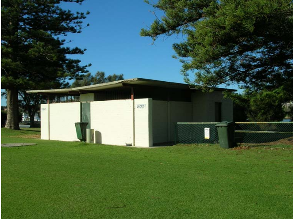
Figure 99 View of the northeastern toilet block. Hocking Planning and Architecture, August 2009
