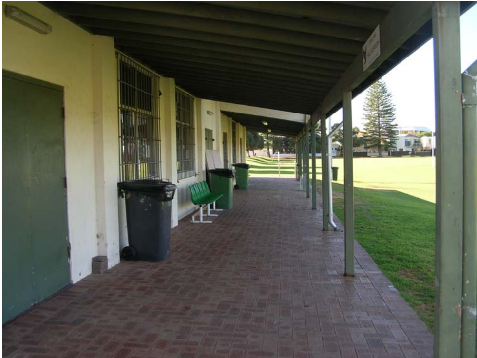
Figure 72 Verandah, looking east. Hocking Planning and Architecture, August 2009.
