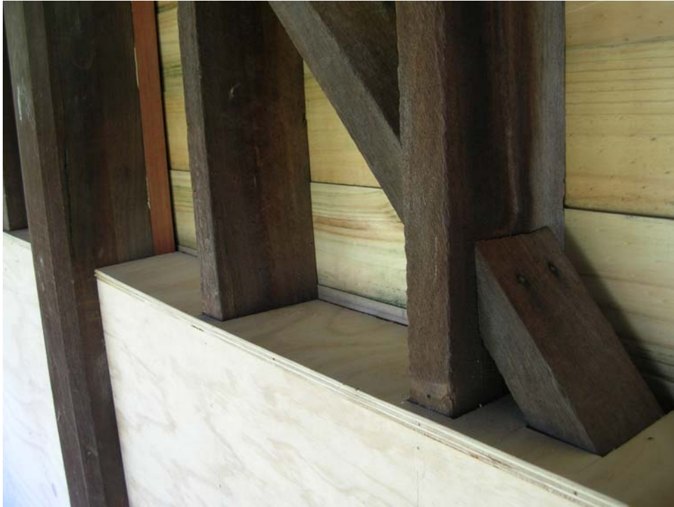
Figure 55 Detail of plywood lining (during conservation work; unpainted) on the internal face of the west wall. This recent addition created a small 'ledge' along the length of the west wall which may pose future maintenance issues as nesting areas for bird pests. Hocking Planning and Architecture, August 2009.
