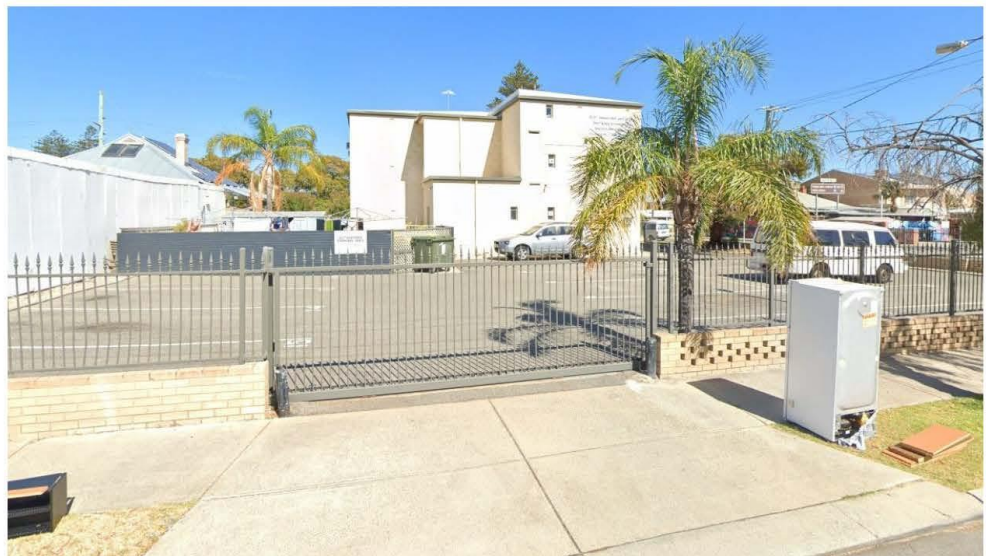
1 Douro road (view from Hickory street)
