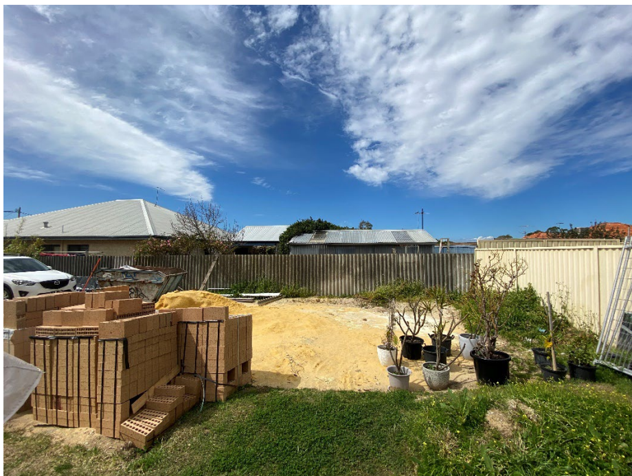
Photo 3: view of eastern boundary of subject site looking towards No. 31 Simper Crescent (eastern neighbour).
