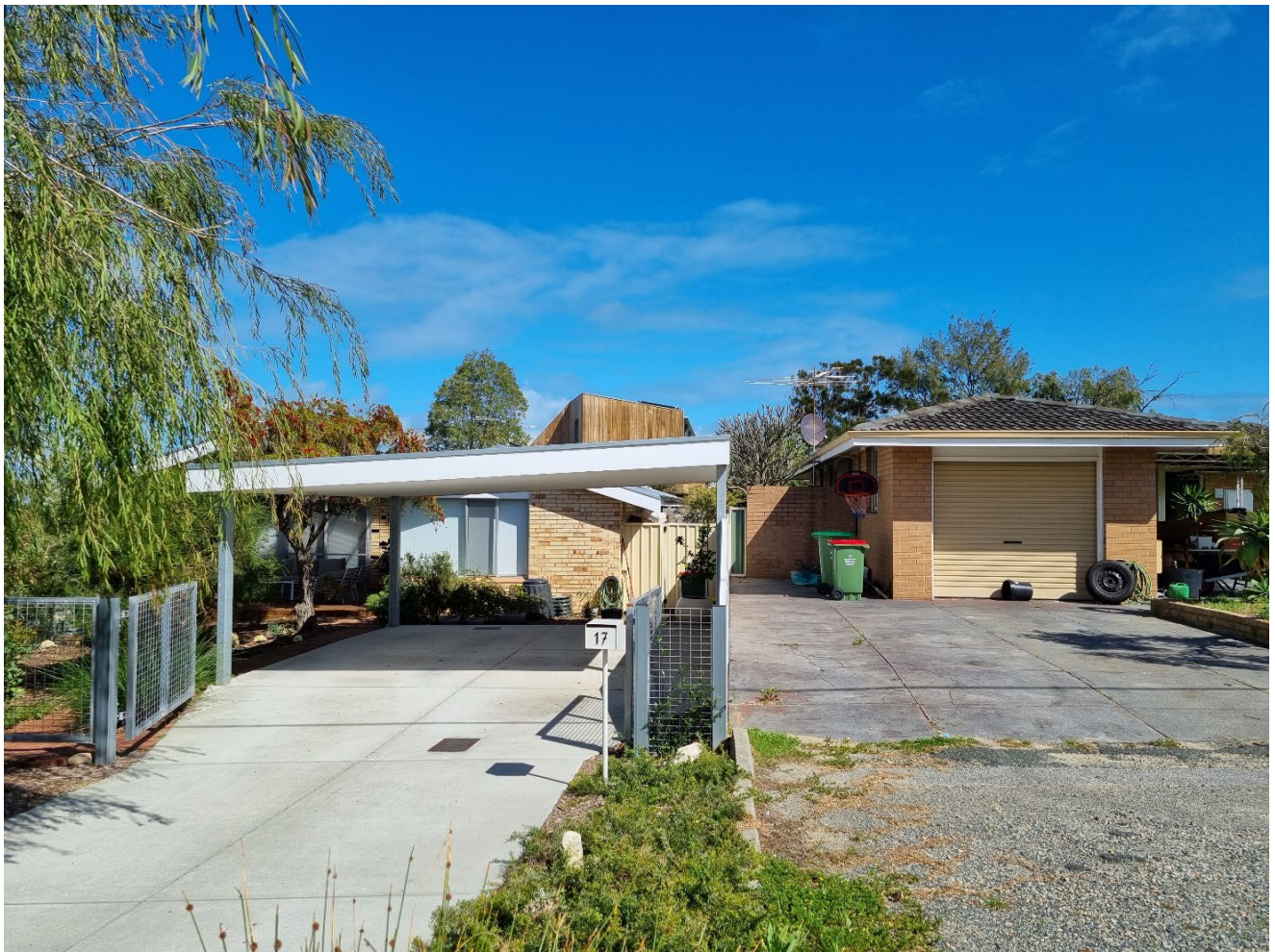
Photo 2: Photo showing existing level difference between Nos. 15 (subject site) & 17 Prowse Street.
