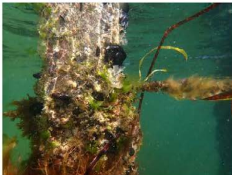
Jetty Ladder missing rung
