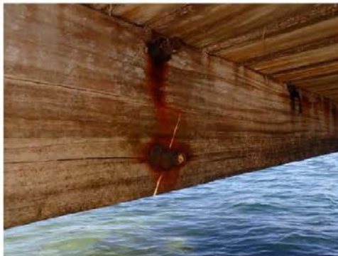
Typical internal face condition
