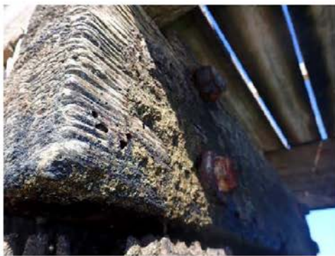
Bent two headstock condition
