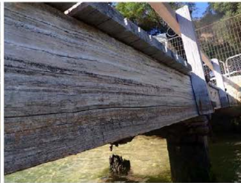
Typical external face condition
