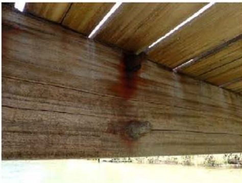
Typical internal face condition
