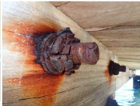
Typical fixing condition
