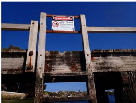
Jetty Ladder above waterline
