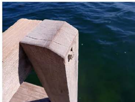
Handrail in good condition (1)
