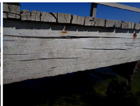
Stress cracking external face
