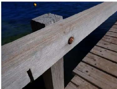
Handrail in good condition
