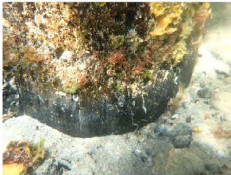
Pile 1A seabed condition (1)
