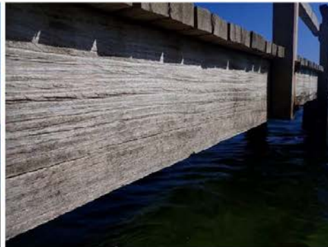
Typical external face condition
