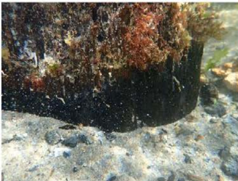
Pile 1A seabed condition
