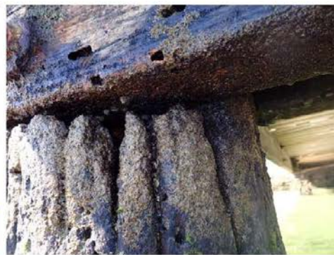
Bent two headstock condition (1)
