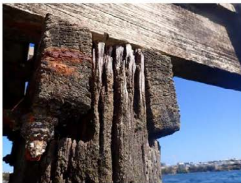
Bent two headstock condition (2)
