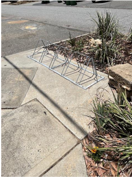
Figure 10: Bike rack on footpath is a trip hazard
