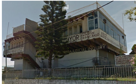
2015 Street View of 20 Moran Street, Google Maps.
