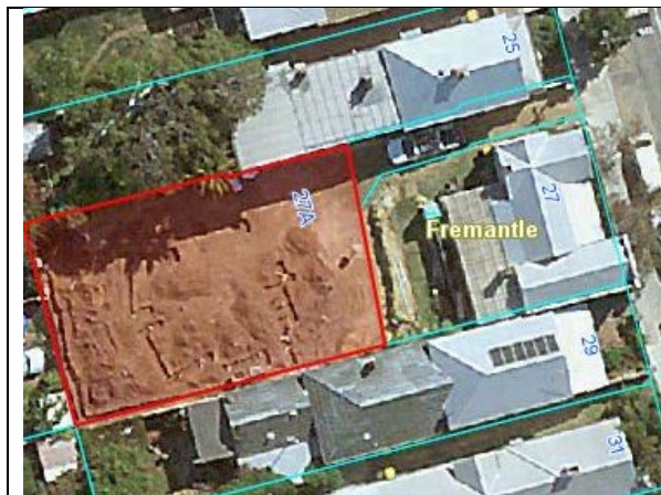
April 2017 aerial view of site, CoF Intramaps.
