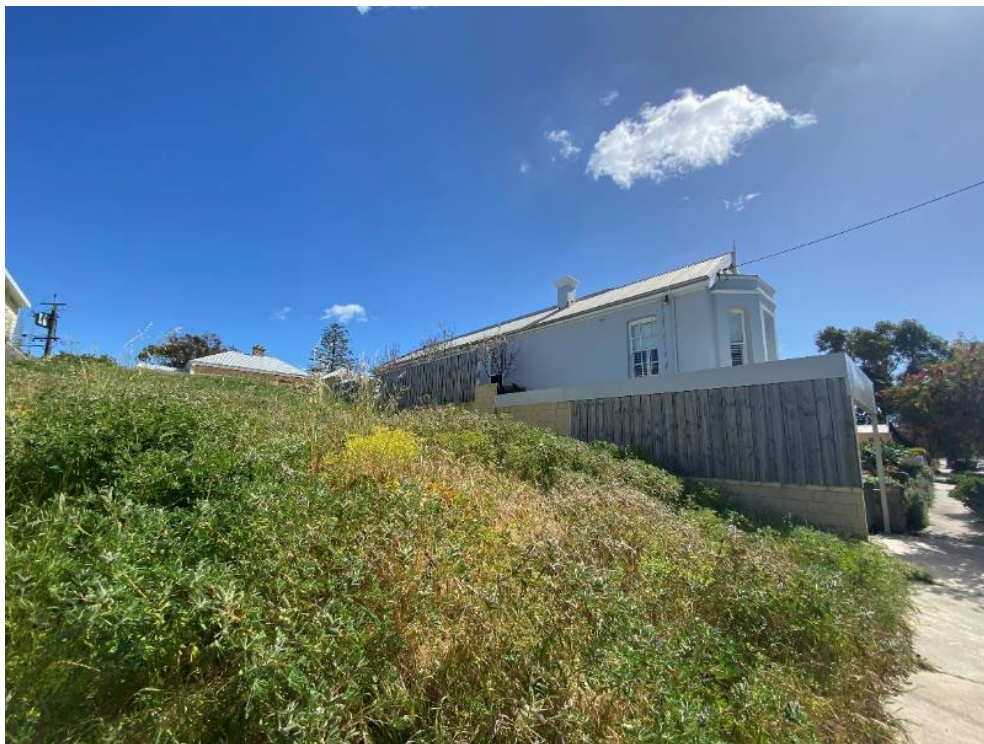
Photo 4: View of south-western elevation of subject site
