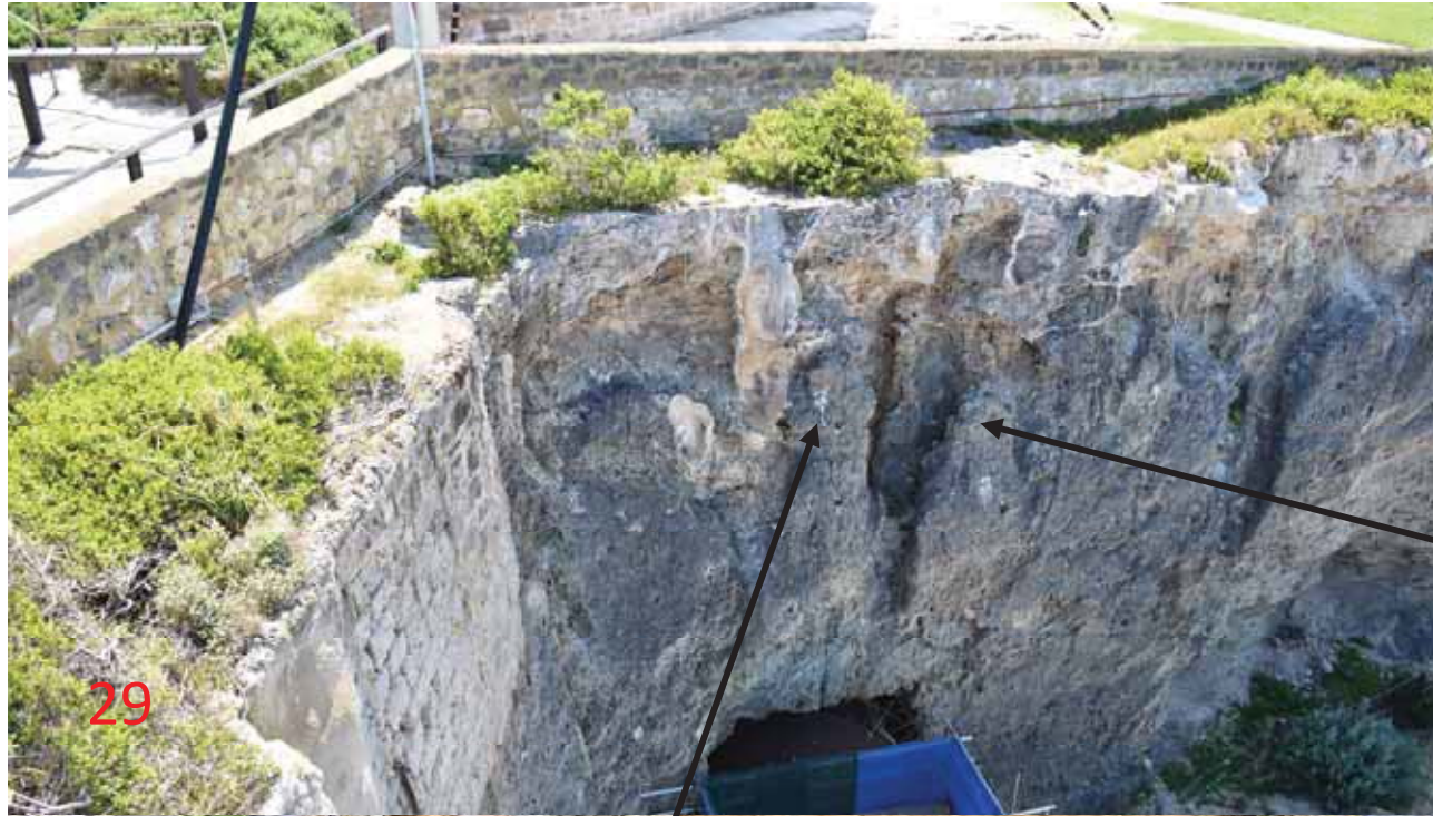
Area 7 – Vertical Face over western tunnel portal
