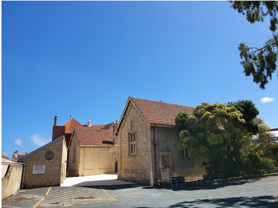
Photo 2 – Site from entry on Norfolk Street
