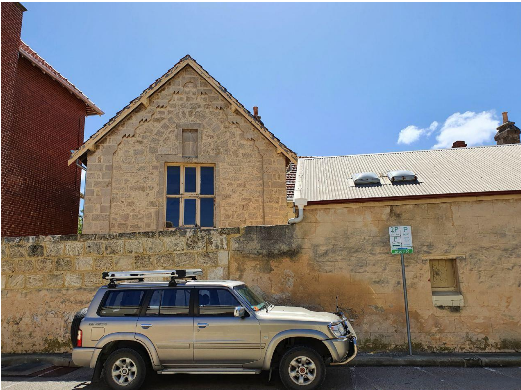
Photo 6 – Existing buildings from Norfolk Lane
