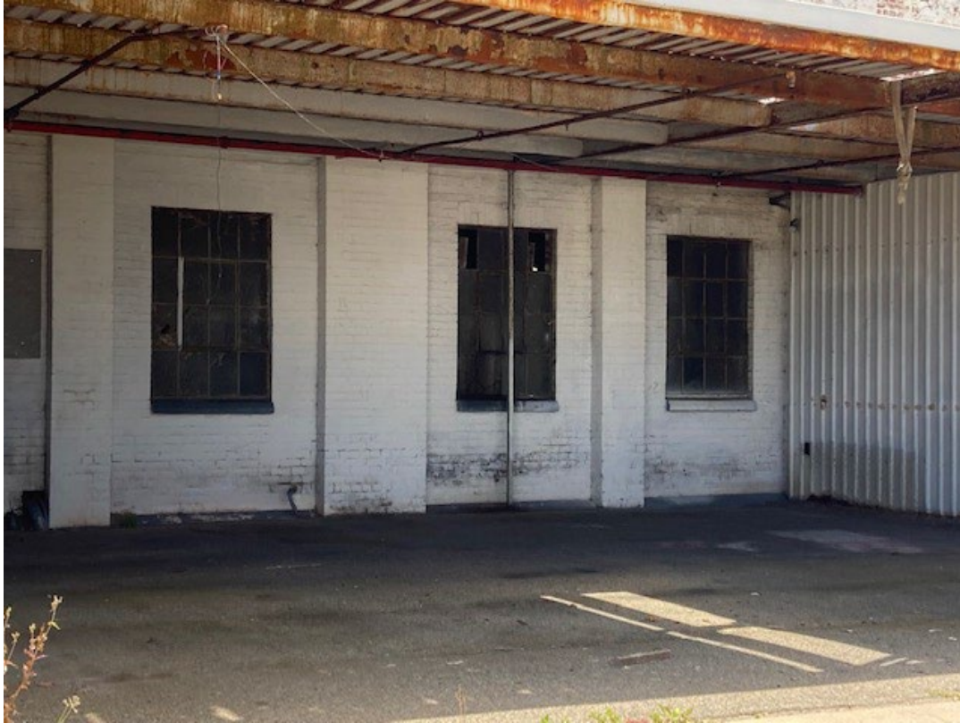
Detail of the steel framed windows to the J. Gadsden Pty Ltd Building (1937 – 1939).
