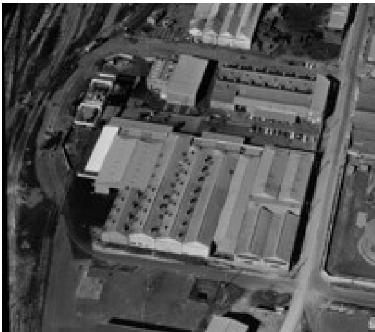
Detail of 1964 aerial photograph
