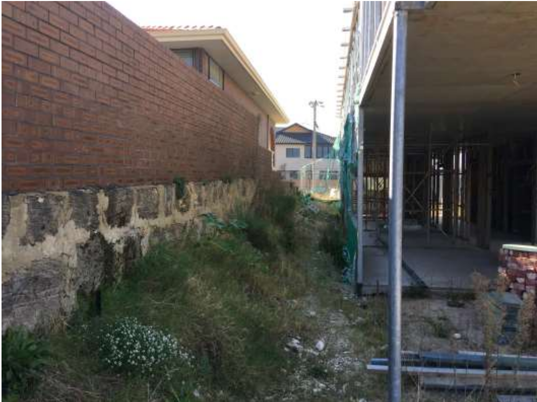
Photo 3: View from adjoining southern lot to existing dividing fence and retaining wall
