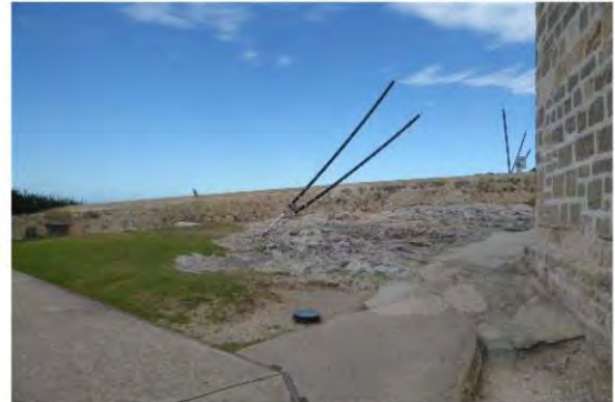
Figure 94: Capstone to the south west of the Round House and mast ties
