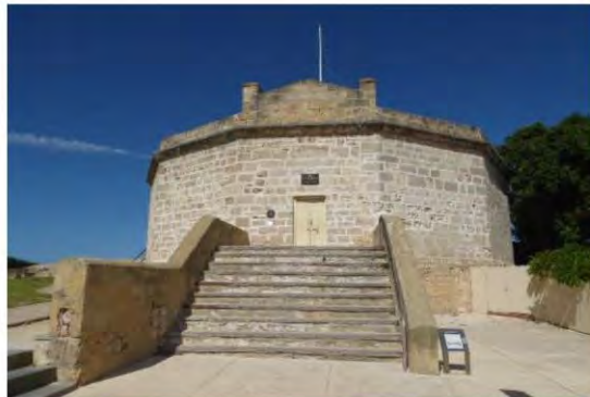
Figure 55: The Round House viewed from the top of the steps
