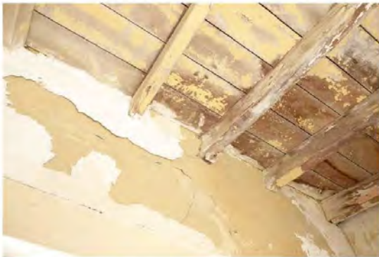
Figure 143: Drummy and patched render
