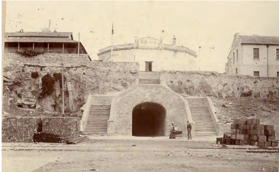
Figure 17: View of Round House from High Street, 1890s. Courtesy City of Fremantle Local History Collection, image 650.
