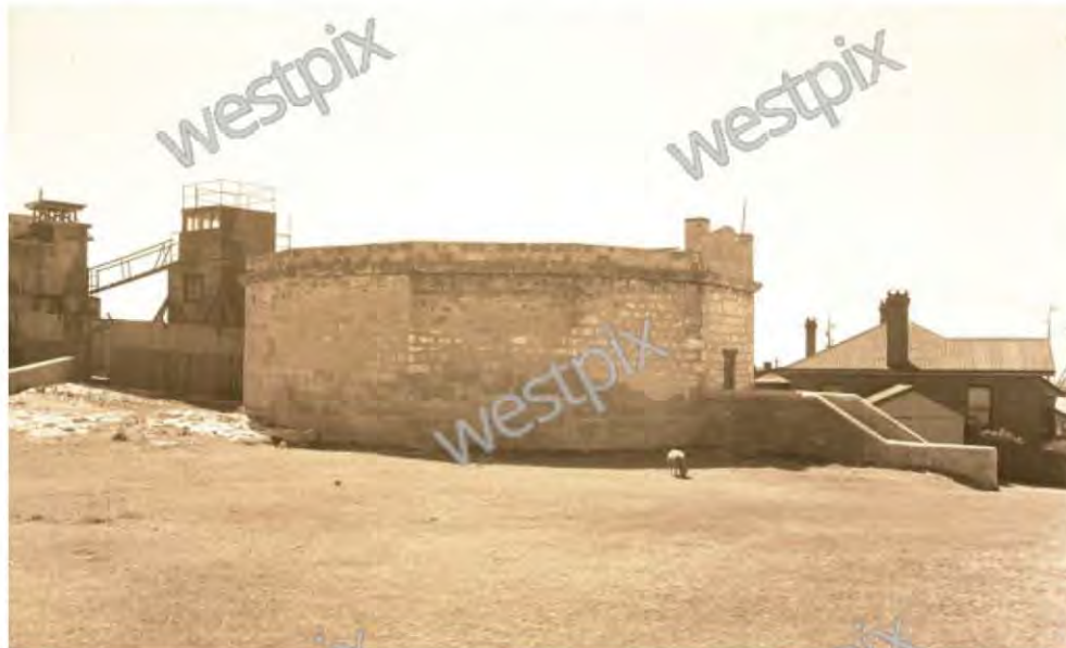
Figure 37: View of the south side of the Round House. 1951. Courtesy Westpix image 35529.
