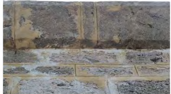
Figure 48: Previous repairs
