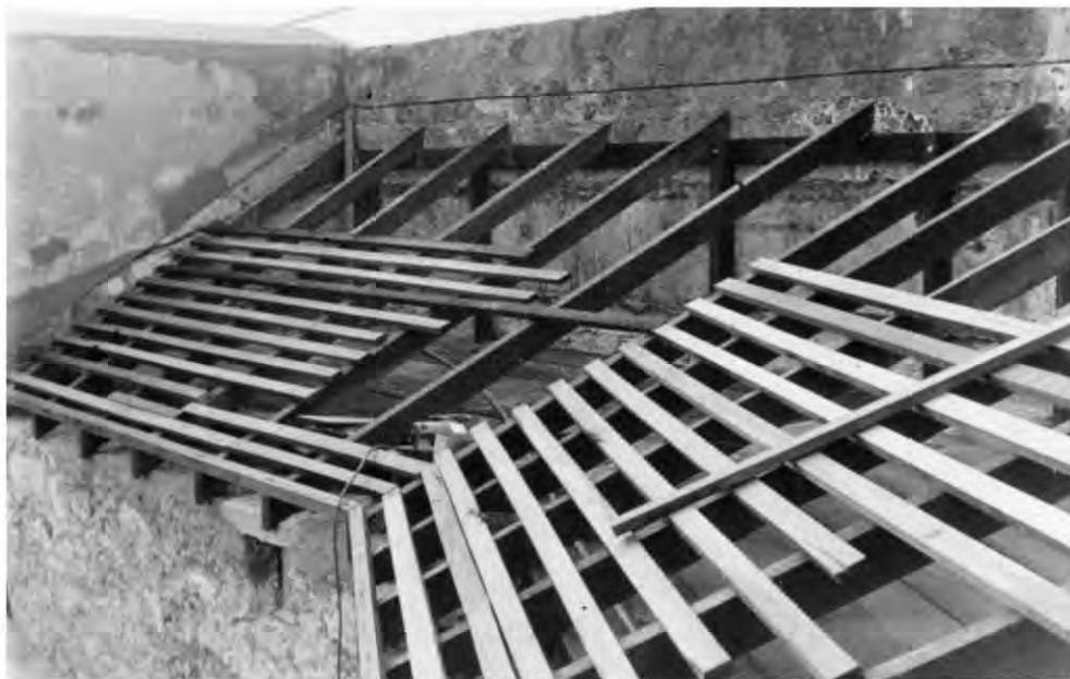
Figure 46: Detail of Roof works, 1975.
