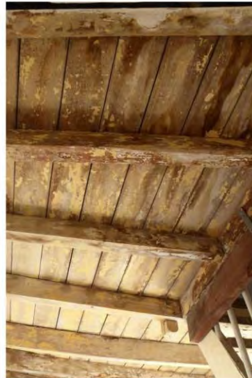
Figure 159: Ceiling to Room 1, underside of floor to Room 14
