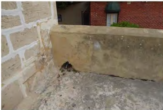
Figure 15: Drainage channel and discharge point
