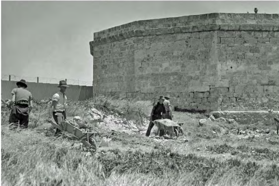
Figure 31: Creation of the grassed area alongside the Round House, 1937 Courtesy Fremantle Port Authority
