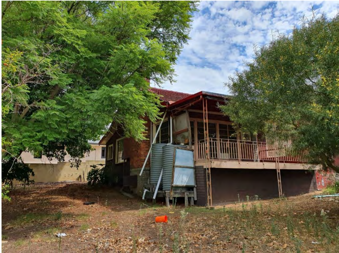
Photo 7 – South east corner of original portion of dwelling
