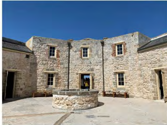
Figure 117: View east across courtyard to main entrance
