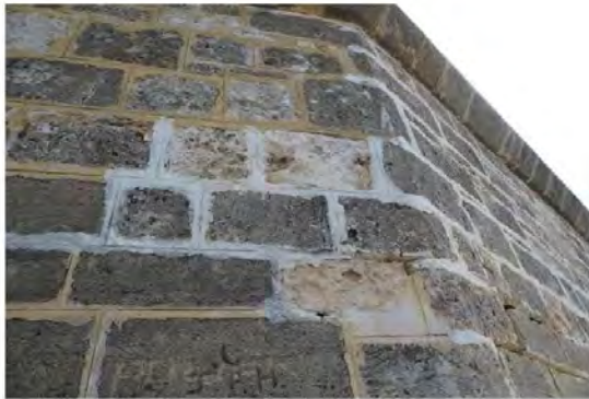
Figure 49: Mix of mortars in repairs
