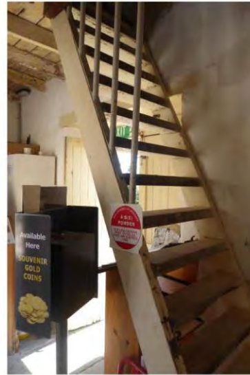
Figure 156: Steep timber stair (ladder stair) from Room 1 to Room 14
