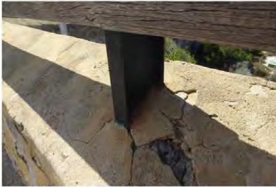
Figure 89: Cracked render
