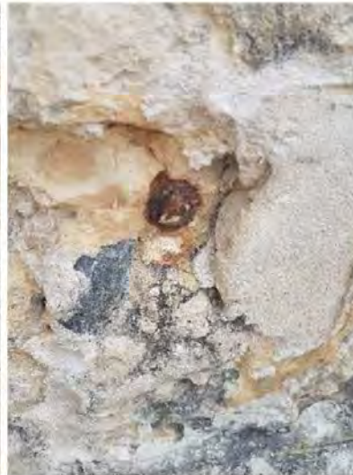
Figure 41: Pins from old sign (removed)
