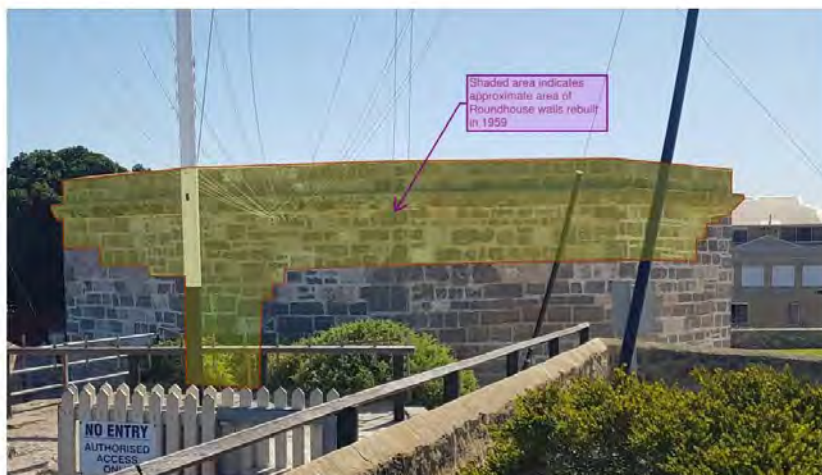
Figure 35: Approx area of Roundhouse walls rebuilt in 1929 / 1959 conservation and restoration works
