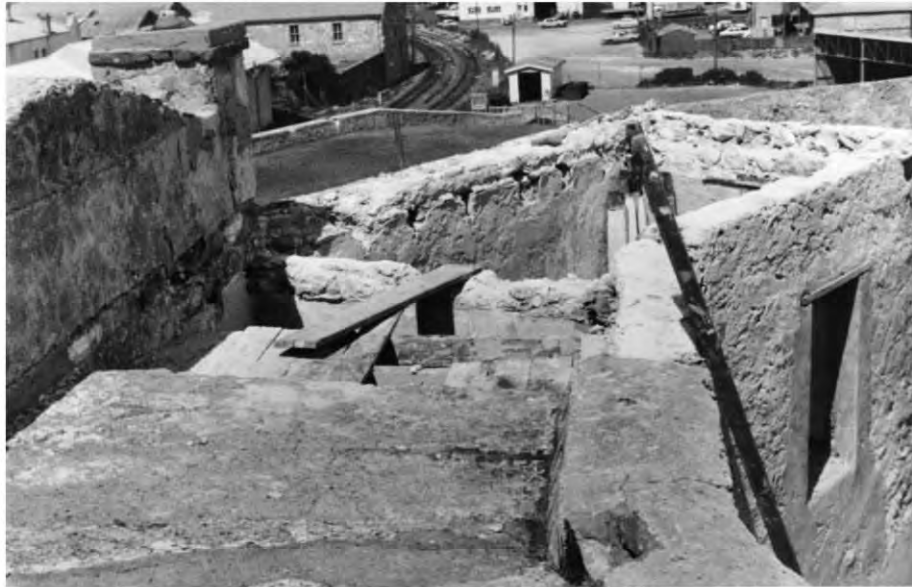
Figure 47: Flat roof on upper level prior to works, 1975. Courtesy City of Fremantle
