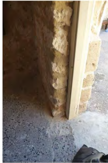
Figure 179: Illustrative thickness of cell walls
