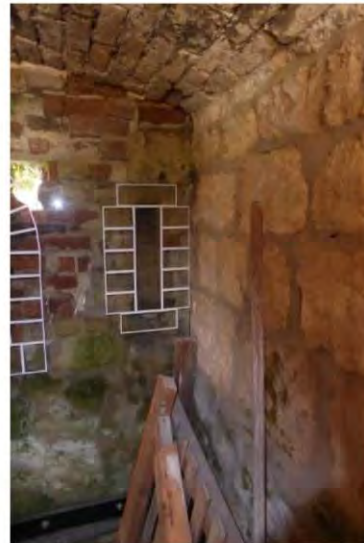
Figure 112: Inside the Bakehouse with interpretation showing where the oven originally was located
