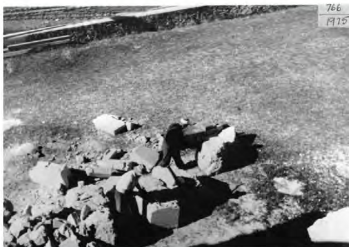
Figure 33: 1975 limestone blocks being cut by hand on site
