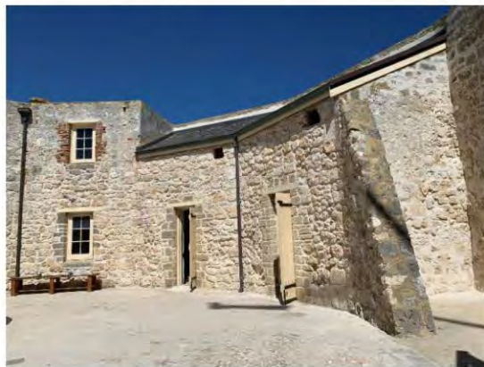
Figure 118: View east across the front of Cells 1 and 2
