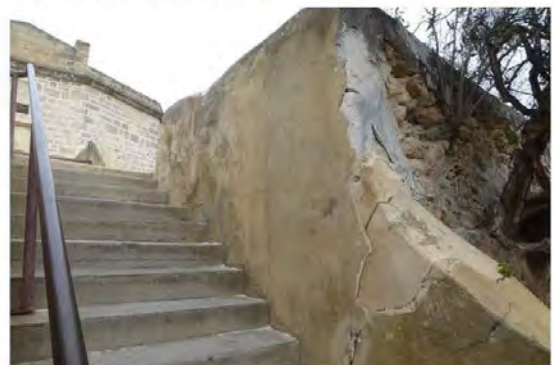
Figure 6: Failing render to steps from High Street
