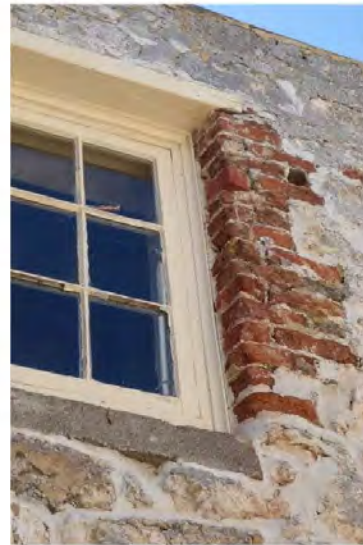
Figure 96: Brick infill around window
