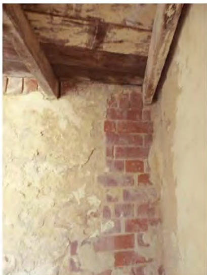
Figure 171: Room 1 brick infill c.1975
