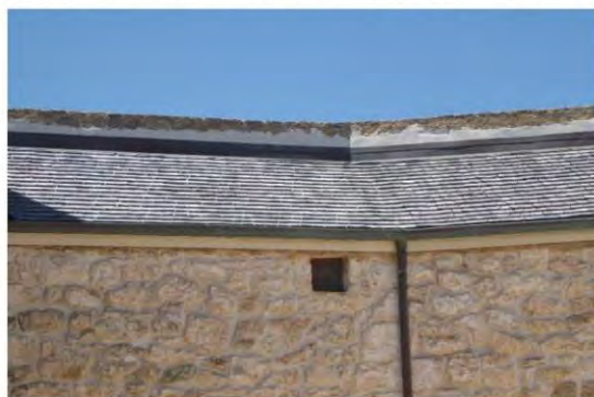
Figure 129: Shingle roof over cells 1 and 2
