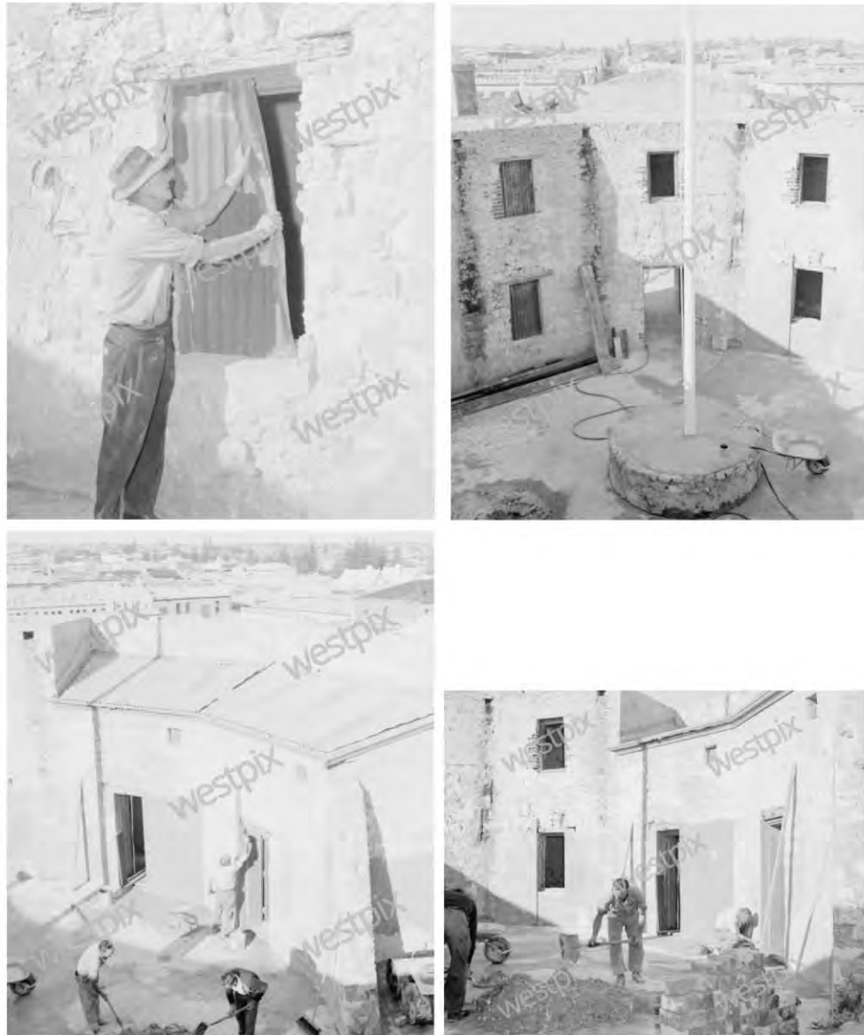
Figure 39: Repairs to the Round House, May 1959, note the render on the walls Courtesy Westpix images 35483, 35484, 35485, 35486
