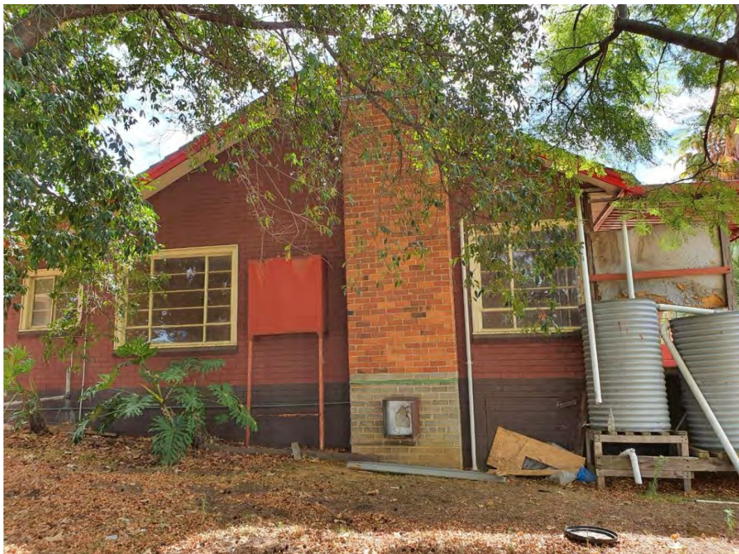
Photo 2 – Southern façade of dwelling (facing Winterfold Road)
