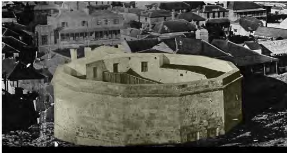
Figure 16: View of the Round House from the Lighthouse, 1879 showing the timber dividing wall and casement windows and flat roof over the cells. Courtesy Curtin University Historical Panoramas.
