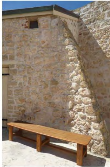
Figure 136: Buttress wall containing remnant fabric from demolished cells
