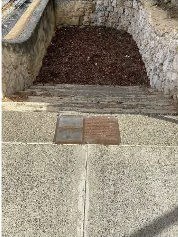
Plate 10. View of truncated northern staircase (note jarrah lined steps)
