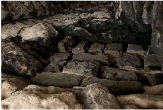
Figure 151: Brick infill in stone chimney
