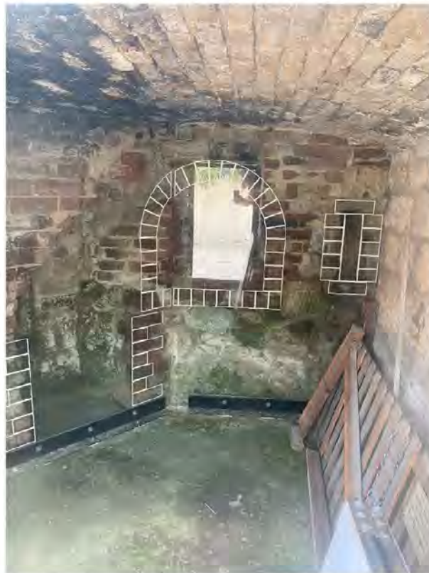
Plate 7. View into the Bakery showing current interpretative glass installations (2019)
