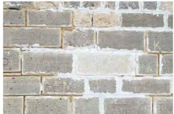
Figure 42: Bad repairs
