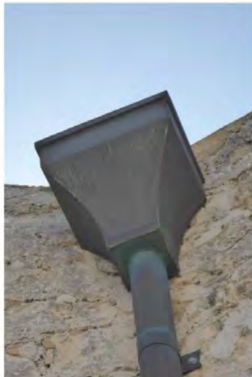
Figure 101: Copper rainwater head
