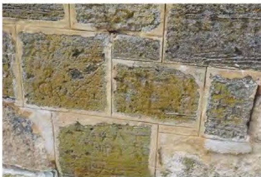
Figure 53: Lichen growth on stones face 7
