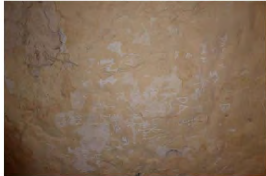
Figure 173: Partially rendered wall in Cell 4
