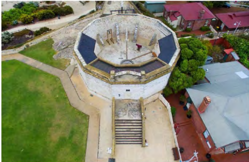
Figure 46: Roundhouse roof from NE
