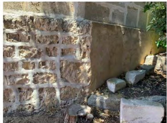
Figure 103: Rendered and un-rendered sections of plinths to faces 12 and 11
