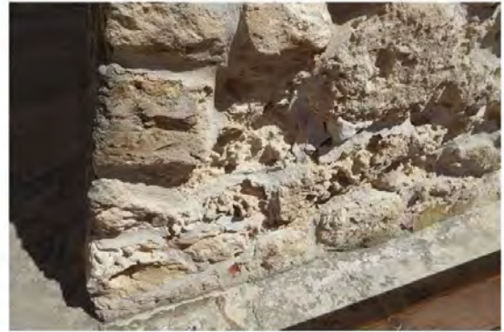
Figure 114: Stone erosion
