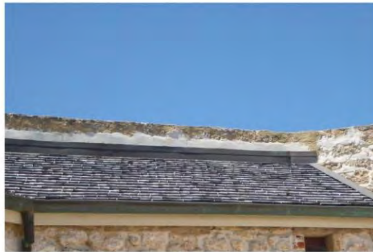
Figure 124: Shingle roof over Cell 4
