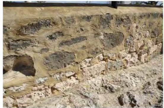
Figure 84: Previous repairs to boundary wall
