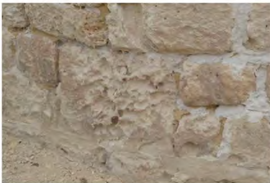
Figure 25: Missing mortar
