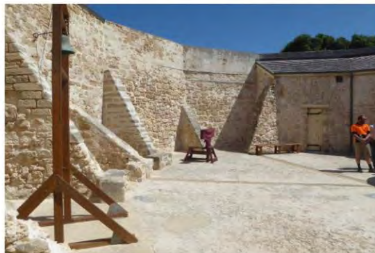
Figure 135: View north across rear (west) wall towards Cell 3
