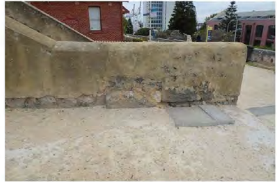
Figure 28: Southern side of balustrade
