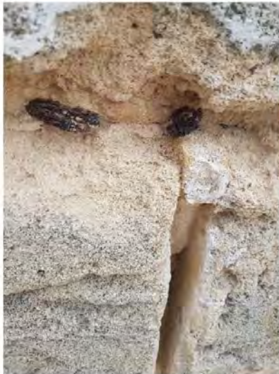
Figure 42: Steel embedments West side
