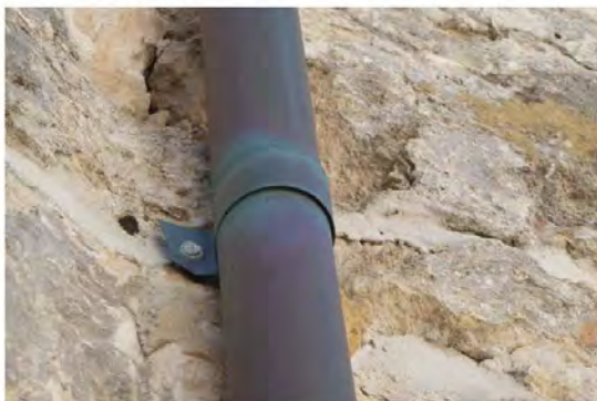
Figure 103: Copper downpipes
