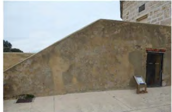
Figure 88: Rendered limestone balustrade and wall to Round House steps, incorporating former Bakehouse
