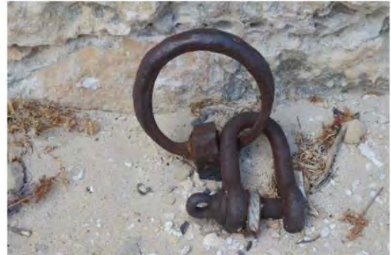
Figure 98: Remnant rope fixings from earlier Signal Mast
