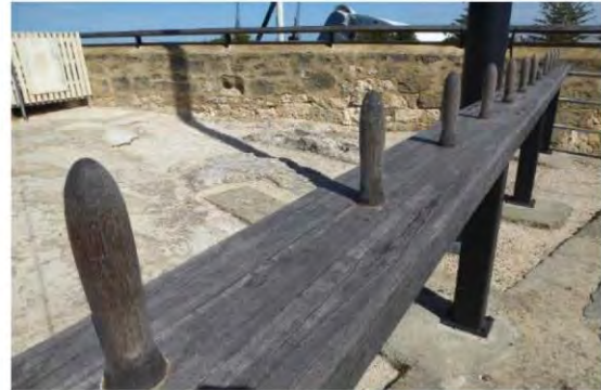
Figure 111: Timber belaying pins at base of signal mast
