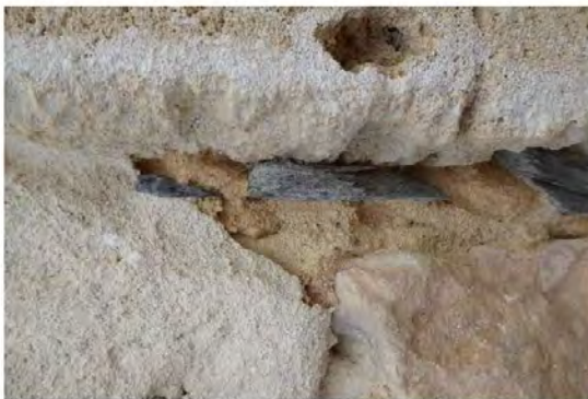
Figure 31: Joint packers
