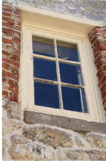
Figure 138: Typical replacement timber framed casement window
