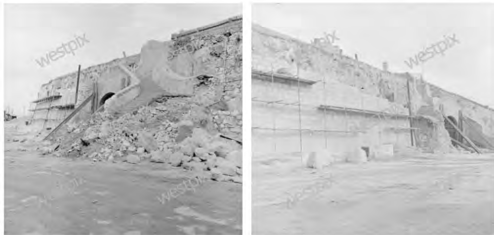
Figure 43: Stabilisation of the cliff face, March 1966 Courtesy Westpix, images 107771 and 107772
