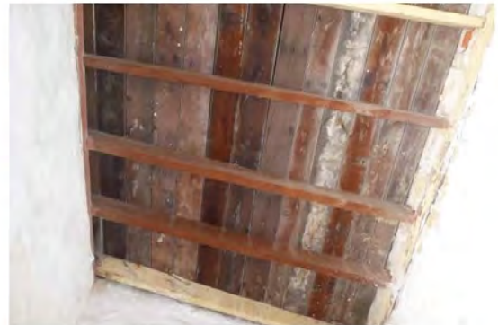
Figure 194: Underside to ceiling in Cell 2
