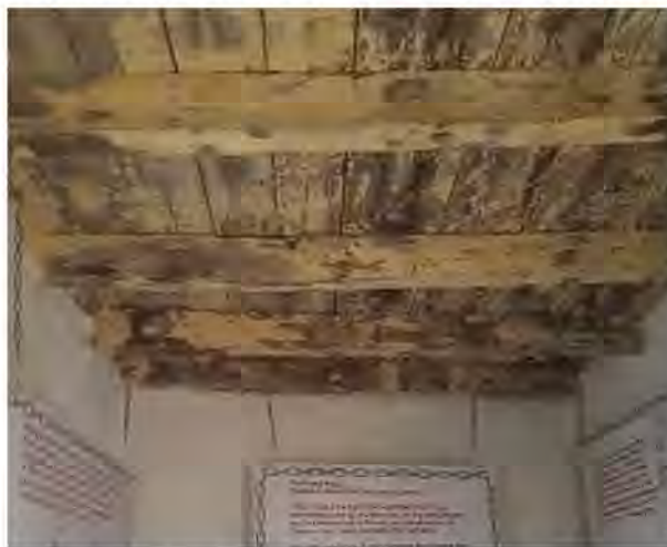
Figure 45: 1st floor joists
