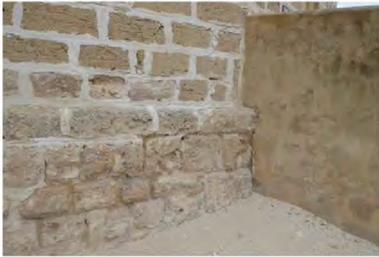
Figure 27: Plinth abutting steps balustrade
