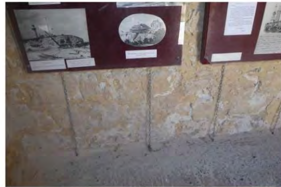
Figure 177: Connection of existing interpretation into concrete floor, Cell 3
