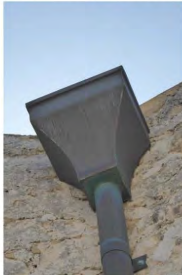
Figure 139: Copper rainwater head
