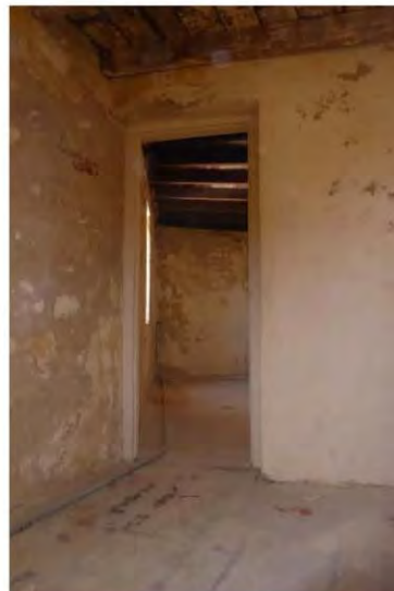
Figure 146: View north through Room 14 looking into Room 13
