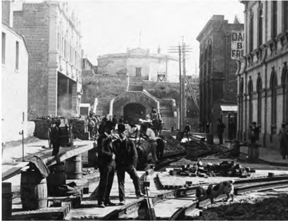
Figure 21: Laying tram tracks in High Street in 1905, Round House in Background. Courtesy City of Fremantle Local History Collection, image LH1892
