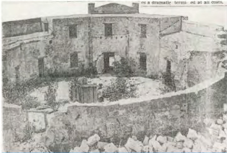
Figure 34: Collapsed wall sections 1929
