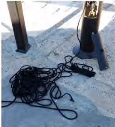
Figure 61: Access hatch and rope stored in the mast
