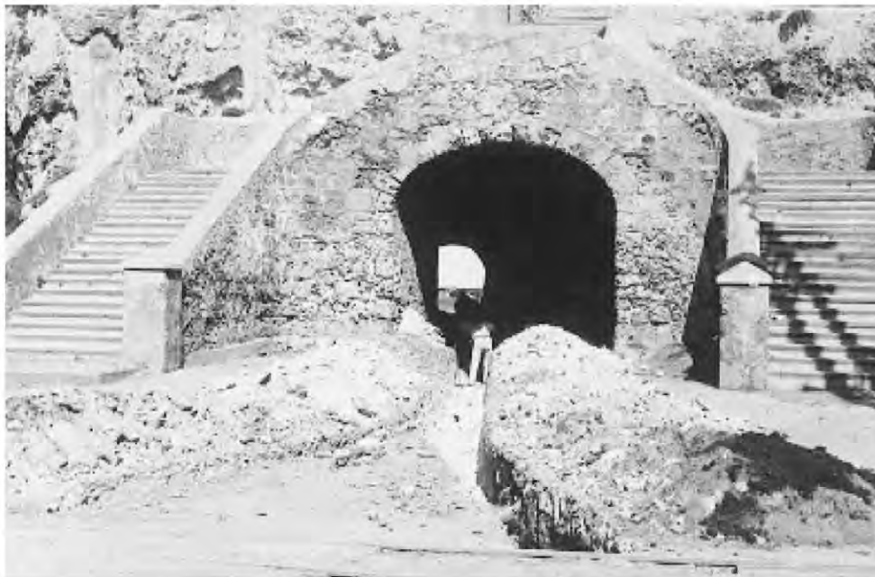
Figure 20: Laying cable through the tunnel from the Powerhouse to the Car Barn in High Street. Courtesy City of Fremantle Local History Collection, image 650
