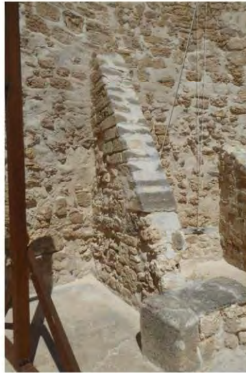
Figure 133: Non-original buttress walls constructed to stabilise the Round House following the collapse of the cells
