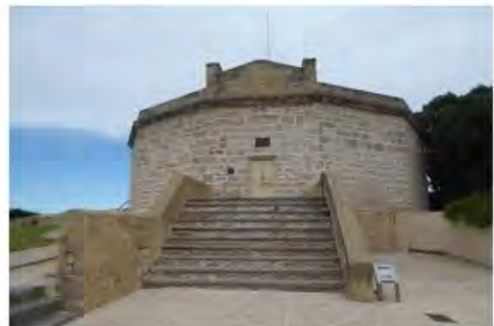
Figure 76: Timber and stone steps leading to the entrance
