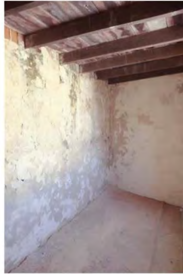
Figure 152: View south through Room 15
