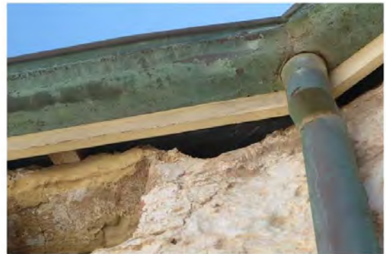
Figure 106: Copper gutters
