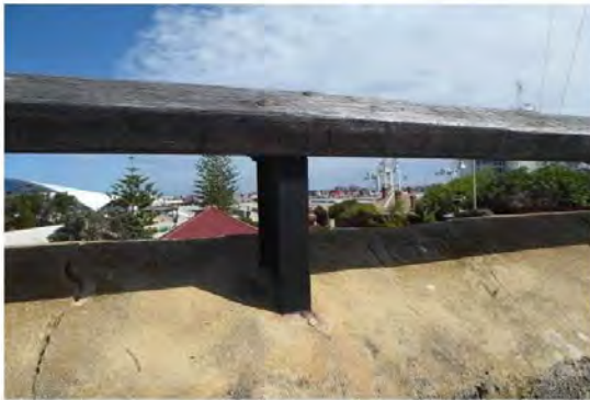
Figure 83: Timber security balustrade to boundary wall
