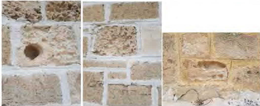
Figure 30: Weathered original limestone block faces
