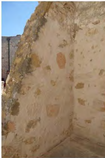
Figure 125: Previous repairs
