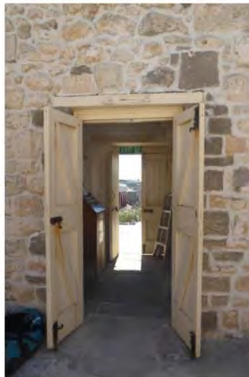
Figure 122: Internal doors looking towards external doors
