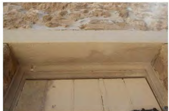
Figure 112: Replacement lintel
