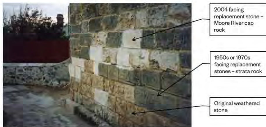
Figure 189: Stone replacements
