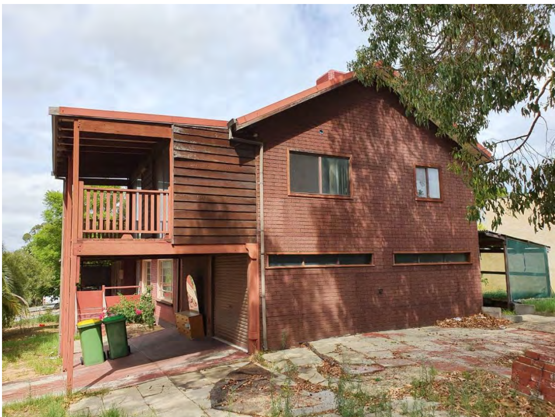
Photo 4 – northern façade of dwelling showing later addition
