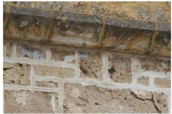
Figure 22: Eroding limestone, traces of white wash
