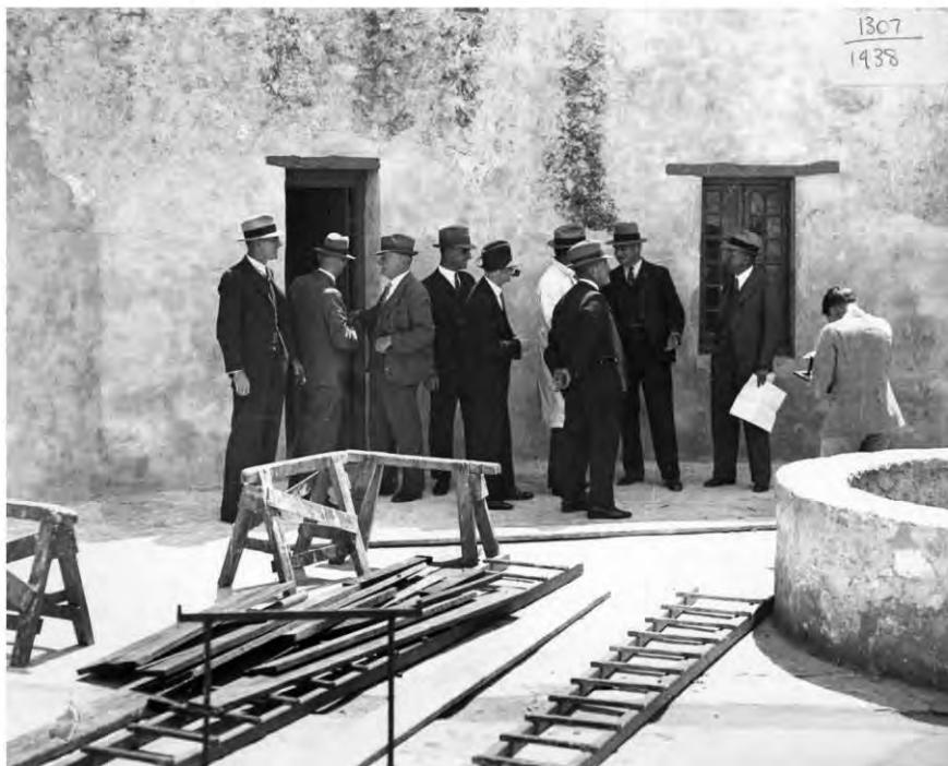
Figure 33: Site Visit, 1938 showing casement windows at Ground Level Courtesy Fremantle Library, Arthur Head Collection, AH 1307.
