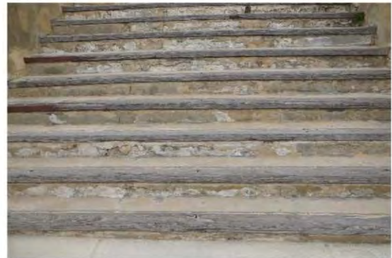
Figure 86: Timber steps leading up to entrance doors
