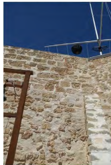
Figure 124: Previous mortar repairs
