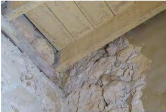
Figure 191: Eroding joints
