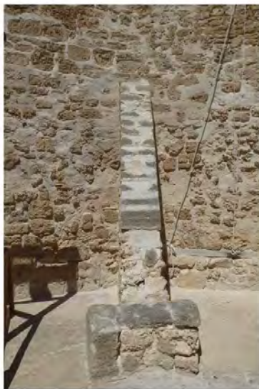
Figure 123: Buttress
