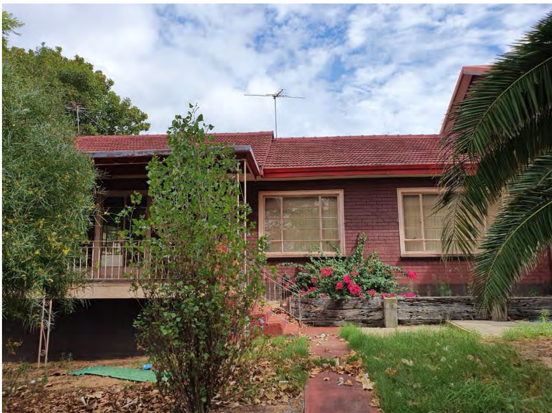
Photo 5 – original portion of dwelling from Paget Street
