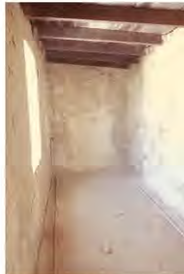
Figure 143: View north through Room 13
