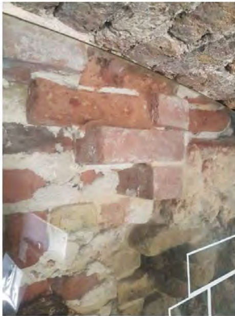
Figure 56: Fretting brickwork
