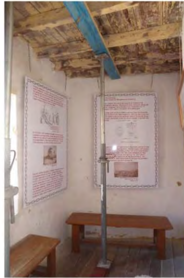
Figure 168: View south through Room 12
