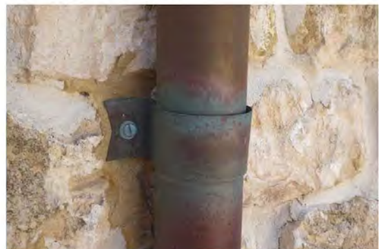
Figure 104: Fixings to copper downpipes
