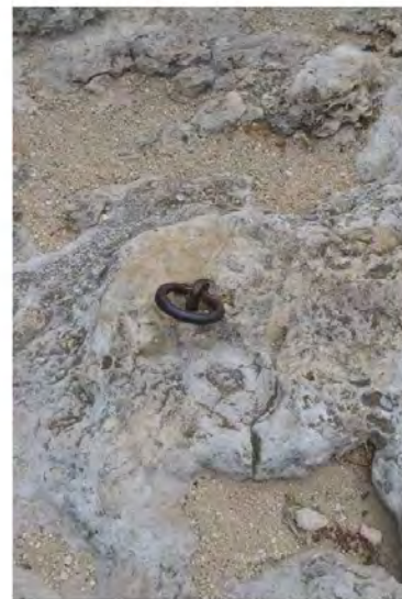
Figure 46: Rope hook in capstone
