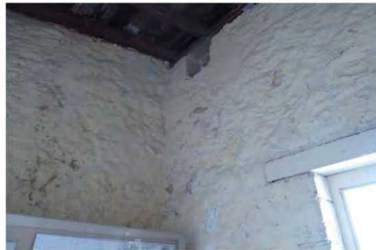
Figure 172: White washed walls in Cell 4
