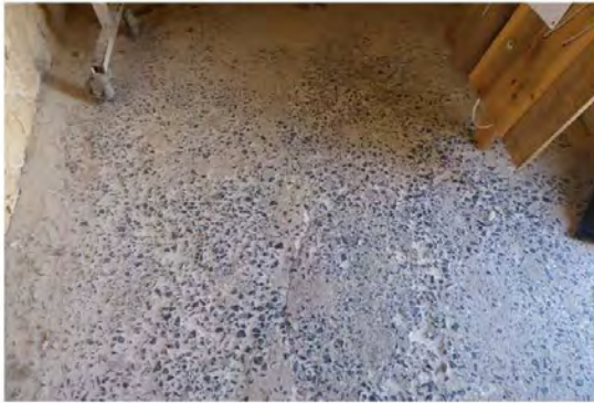
Figure 179: Concrete floor to cells
