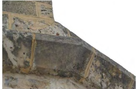
Figure 81: Stone string course below parapet
