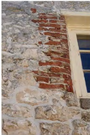
Figure 97: Brick infill around window
