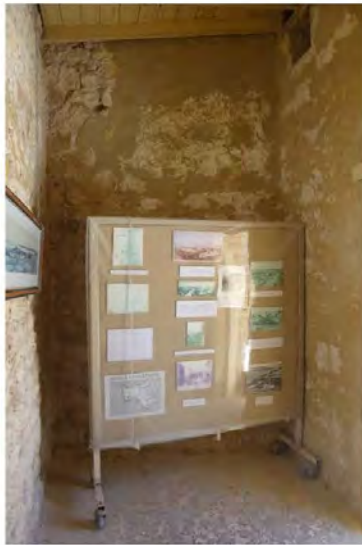
Figure 187: Wearing paint finish to cells and cement repairs
