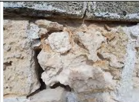
Early yellow/orange mortar (assumed to have used sand from a limestone root pocket on site)
