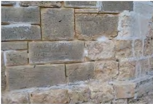
Figure 63: Eroded joints
