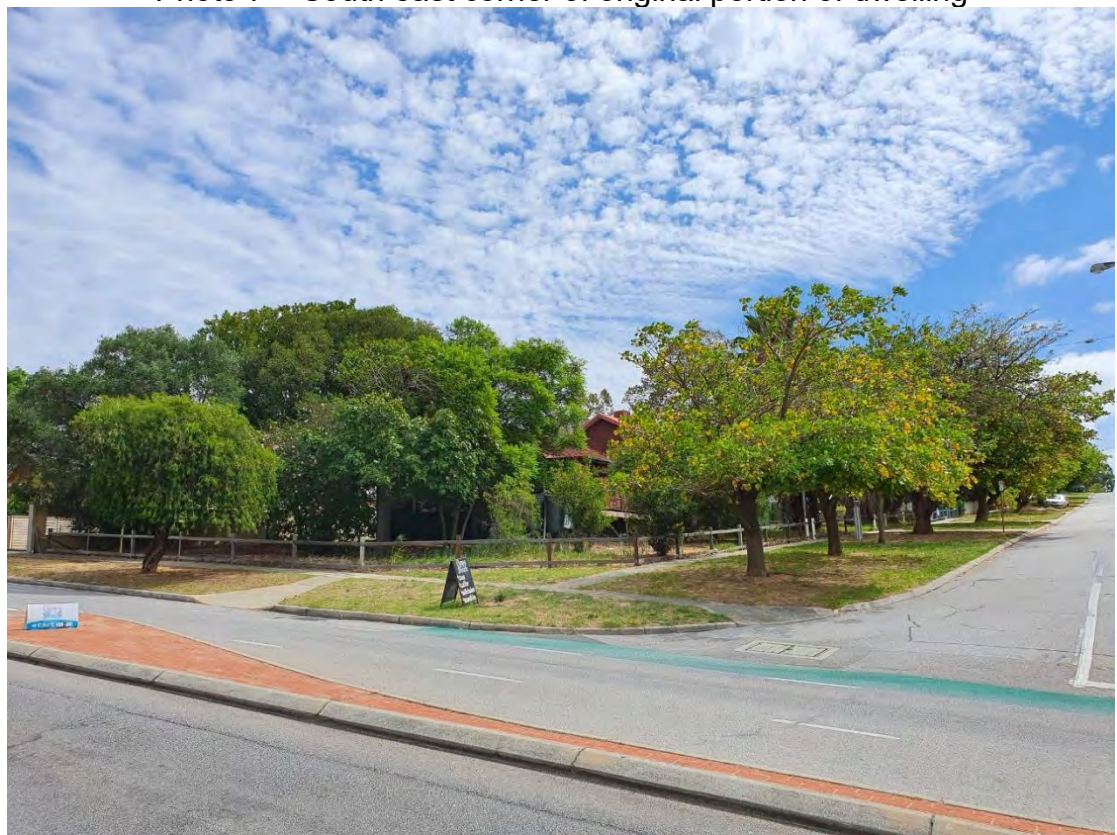
Photo 8 – Subject dwelling from across Winferfold road
