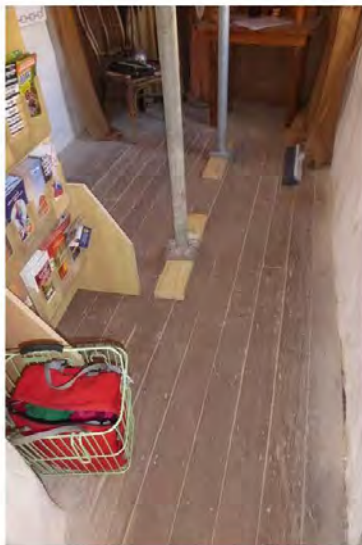
Figure 145: Timber boards to Room 2
