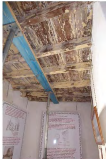
Figure 169: Timber ceiling in Room 12, underside of floor to Room 13 above
