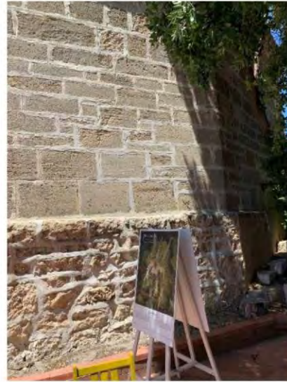
Figure 101: Part of face 12 looking towards face 11
