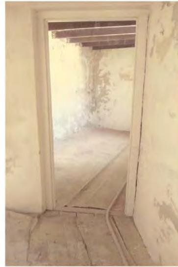
Figure 147: View south through Room 14 looking into Room 15
