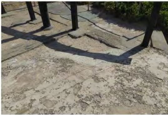
Figure 81: Concrete and capstone surface to look out
