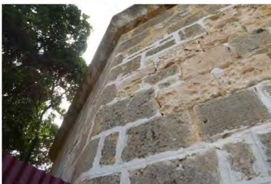
Figure 65: Repairs to face 10
