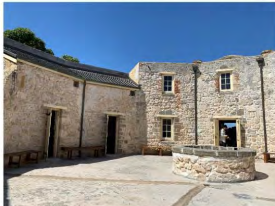
Figure 119: View east across the front of Cells 3 and 4
