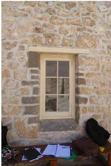
Figure 99: Replacement stones, window and lintels
