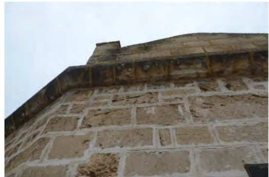
Figure 83: Underside of string course with angled stones
