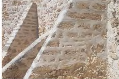
2004 lime mortar surface finish
