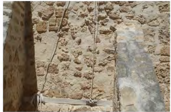
Figure 122: Previous repairs using mortar for stone repairs
