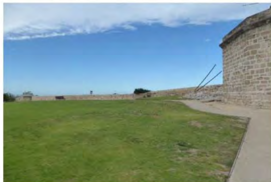
Figure 62: Grassed area to south of the Round House
