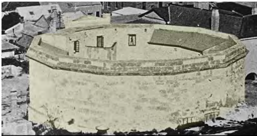
Figure 19: View of the Round House from the Lighthouse, 1902 showing the remnant of the timber-dividing wall.
