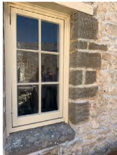
Figure 94: Replacement limestone and windows
