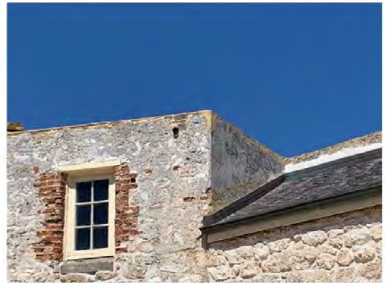
Figure 92: Various treatments to elevations
