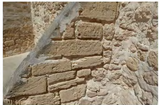
Figure 118: Eroding joints
