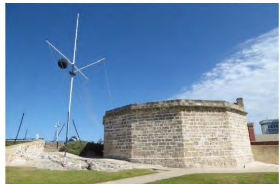
Figure 93: South view of Round House with Signal mast to the west
