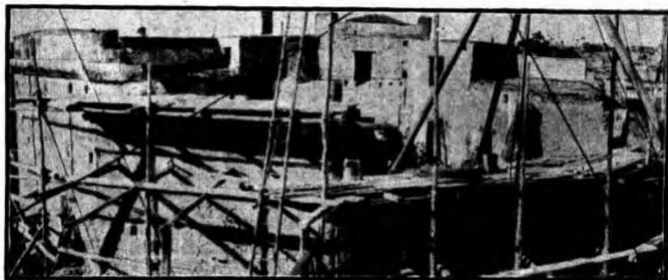
Figure 29: During repairs May 1929.
