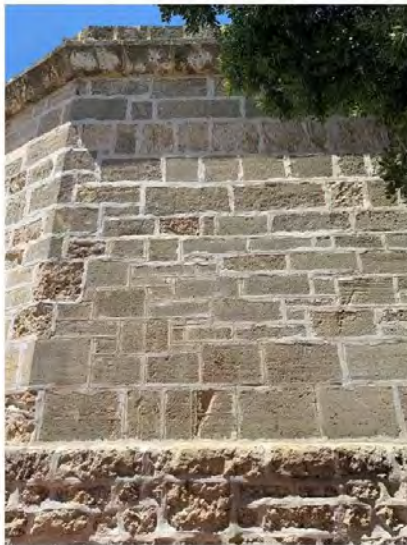
Figure 75: Differences in stone quality face 11
