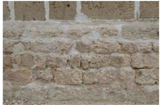
Figure 30: Missing mortar
