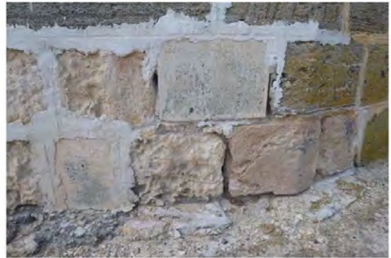
Figure 58: Eroded joints
