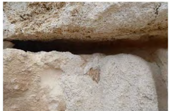
Figure 32: Eroded joint
