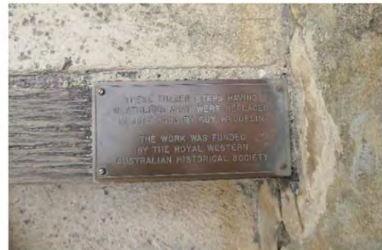
Figure 77: Plaque on steps commemorating the replacement of the timber stapes in 1983
