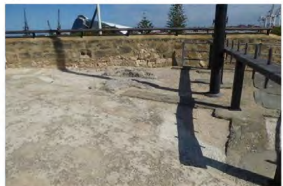
Figure 80: Concrete and capstone surface to look out
