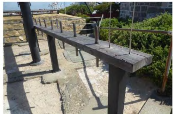
Figure 110: Timber belaying at base of signal mast
