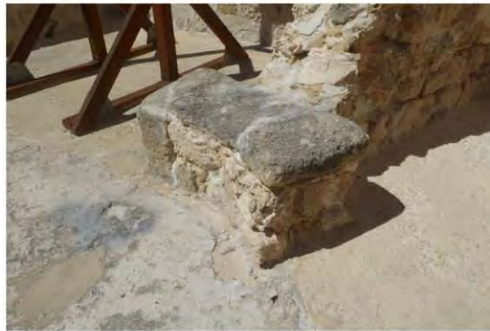
Figure 134: Termination of buttress wall and interpretation of where the original cell wall terminated
