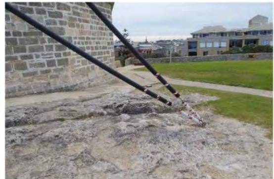
Figure 95: Mast ties connected into the cap stone
