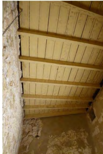
Figure 182: Painted timber ceiling in Cell 1
