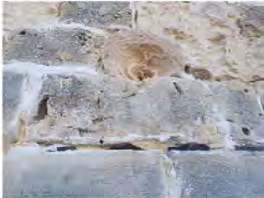
Figure 38: Slate setting blocks for stones
