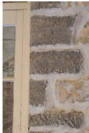
Figure 98: replacement stone around window
