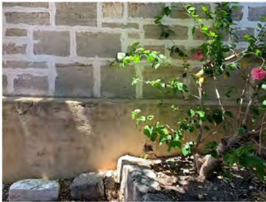
Figure 69: Rendered plinth to face 10
