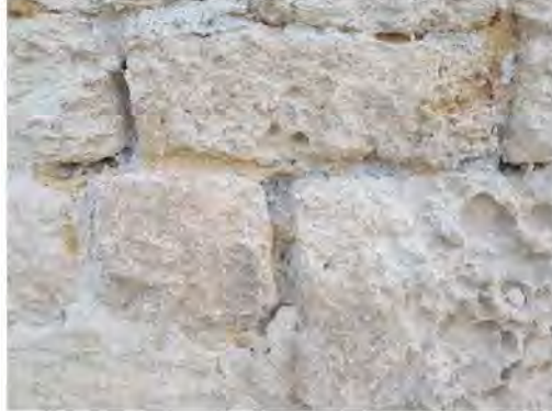
Early mortar – grey with shells, stones and possible inclusion of pozzolans
