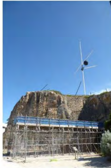
Figure 68: View from Bathers Beach to the Signal Station. Tunnel entrance canopy in the foreground.
