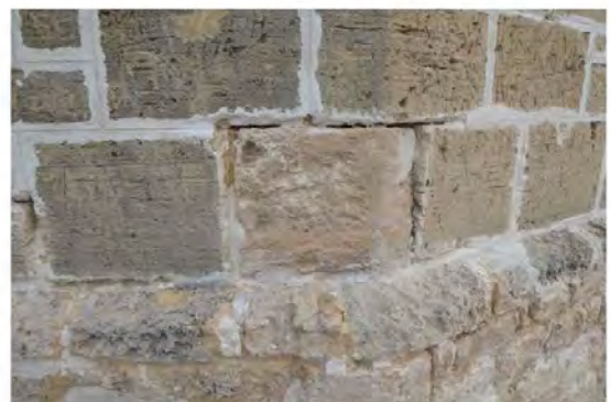
Figure 38: Eroded joints
