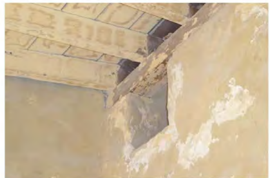
Figure 190: Cement render repairs
