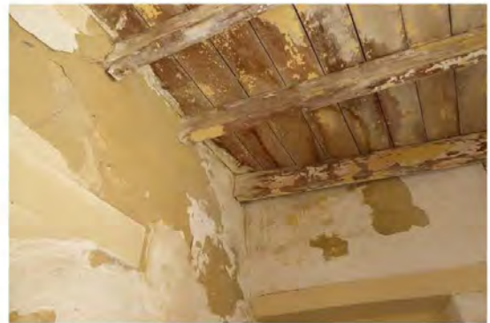
Figure 144: Drummy and patched render
