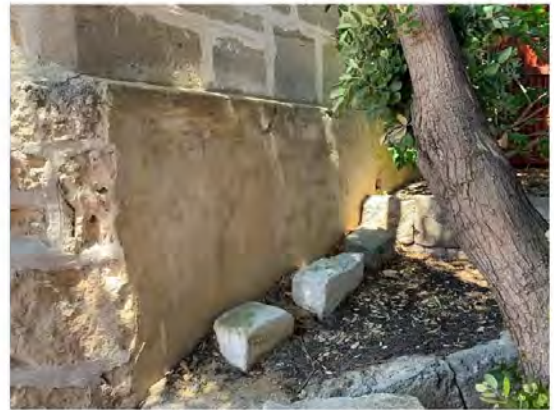
Figure 70: rendered plinth to face 10
