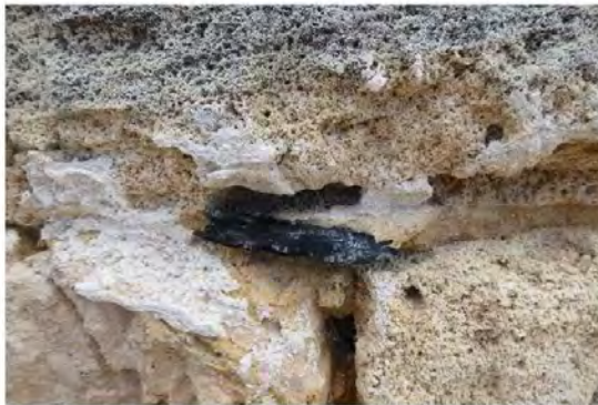
Figure 47: Packers in joints
