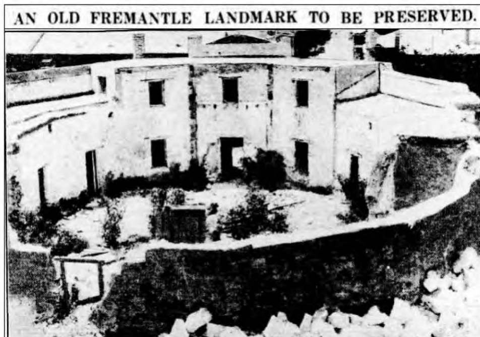
Figure 28: Prior to the repairs April 1929 showing the collapsed wall and loose stones. Courtesy The West Australian , 18 April 1929, p. 22.
