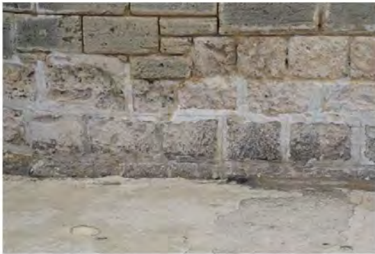
Figure 43: Eroded joints
