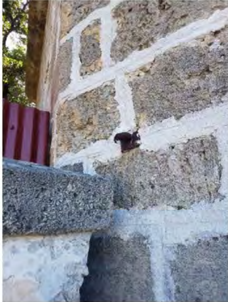
Figure 40: Steel embedment for removal - NW side
