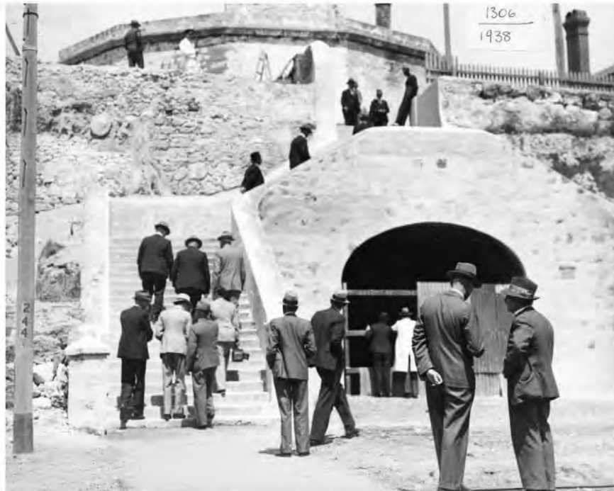
Figure 34: Site Visit, 1938 showing repairs to the steps. Courtesy Fremantle Library, Arthur Head Collection, AH 1306.
