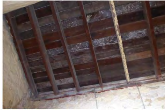
Figure 171: Timber raked ceiling to Cell 4
