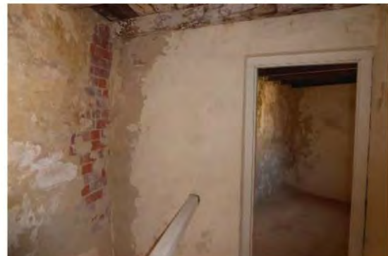
Figure 149: East and south walls of Room 14
