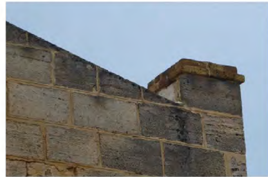
Figure 18: Parapet
