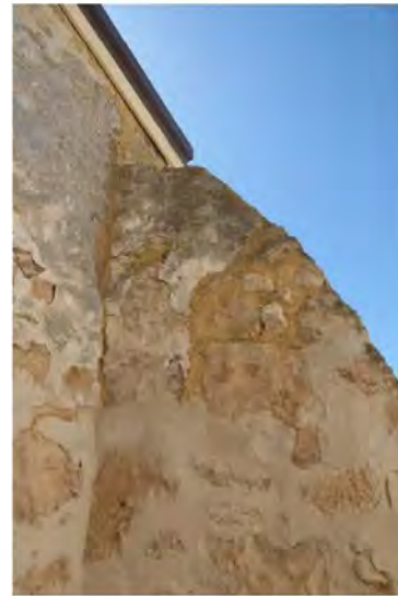
Figure 116: Hard cement and lime repairs
