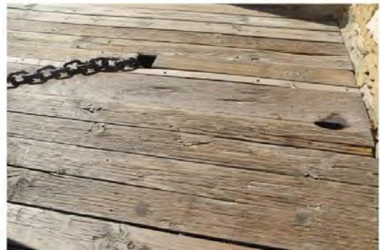
Figure 88: Drying timbers to deck
