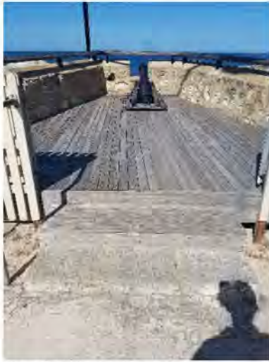
Figure 65: Arthur Head parapet walls
