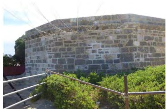
Figure 99: West wall (Face 7) with signal mast ropes attached
