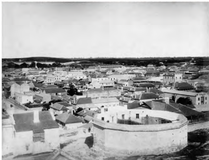
Plate 5. c.1880-90 photograph looking south-east over Round House (State Library WA, SLWA_011246D)
