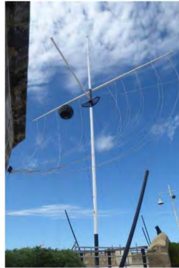
Figure 108: Signal mast yard arms and ropes
