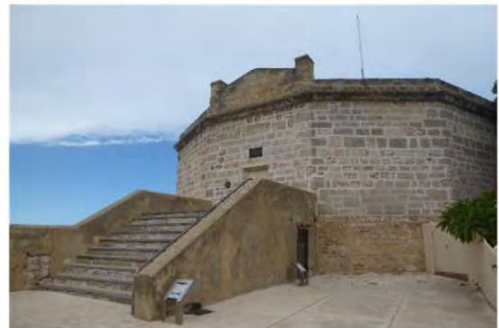
Figure 87: Face 1 and 12, main entrance steps and Bakehouse
