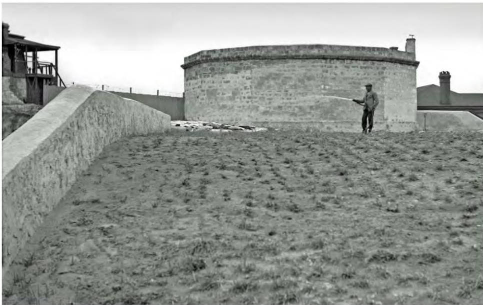
Figure 32: Creation of the grassed area alongside the Round House, 1938 Courtesy Fremantle Port Authority
