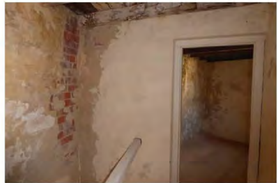
Figure 158: Brick infill
