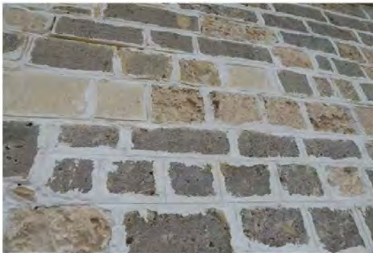
Figure 41: Repaired joints and replacement limestone
