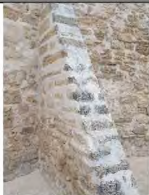
2004 lime mortar – harder capping mortar
