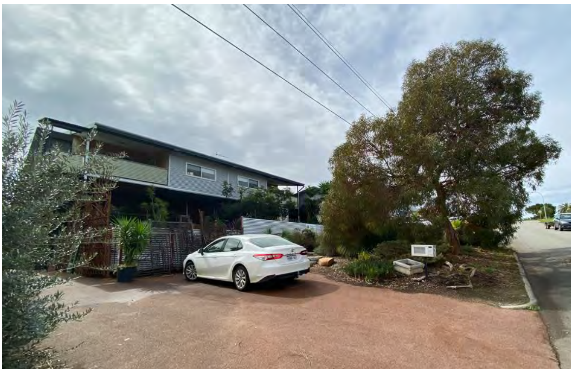
Photo 19: view of eastern neighbour along Stack Street.
