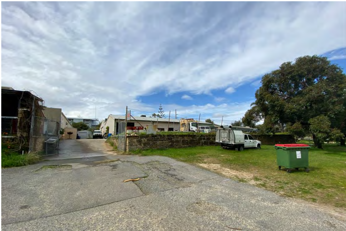
Photo 3: No. 2 Stack Street viewed from Amherst Street
