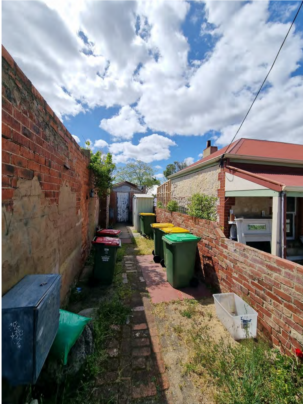
Photo 5: Rear existing common property area to rear of terraced houses and southern adjoining property (10 Francisco Street) side setback area.
