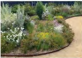
Curten steel edging with crushed aggregate pathway (image: Yerrabingin)
