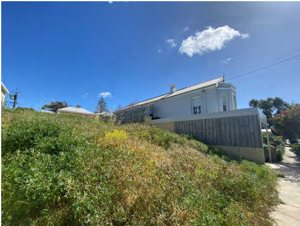
Photo 4: View of south-western elevation of subject site
