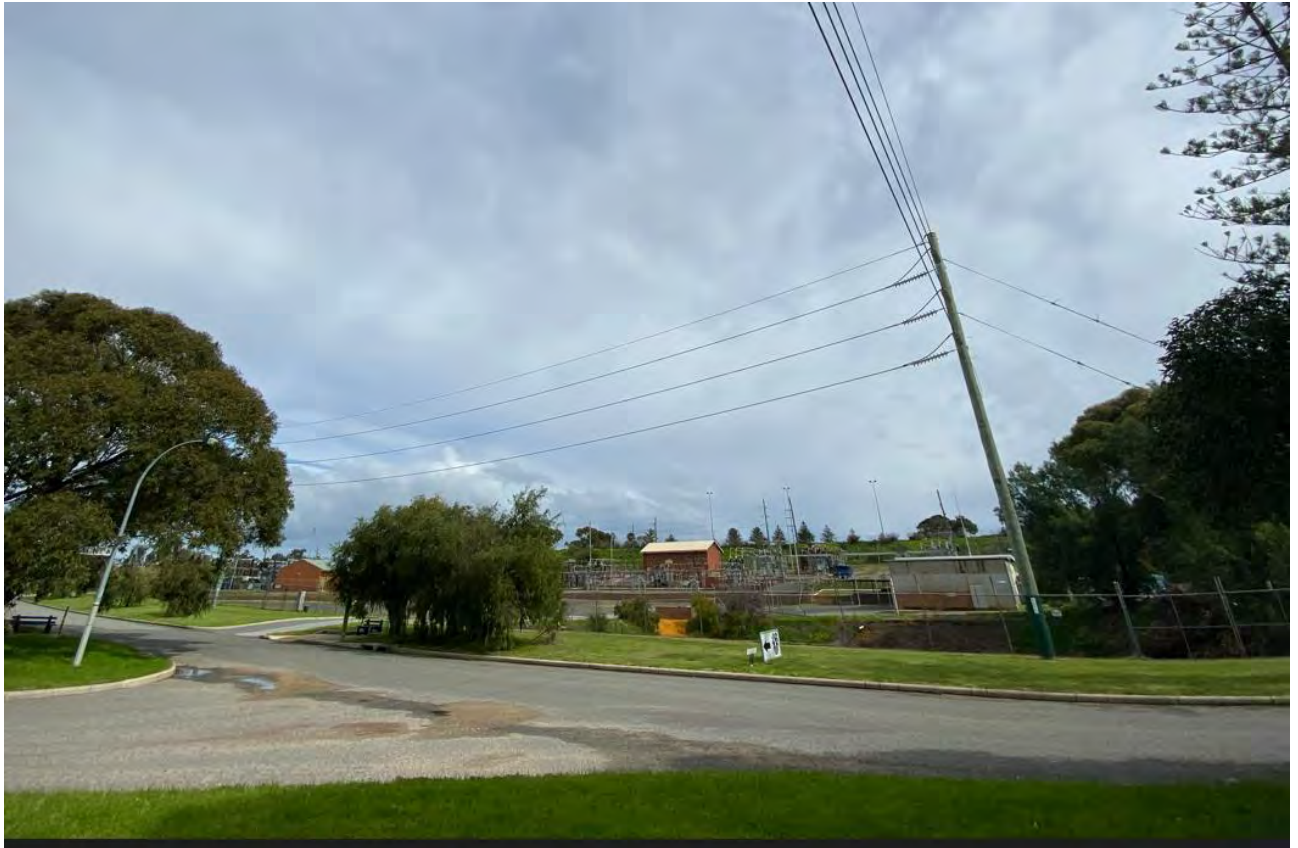
Photo 21: view of Western Power facility
