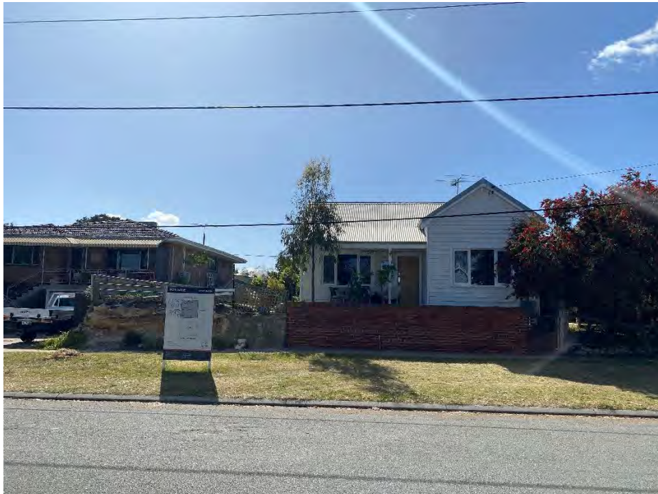
Photo 1: Subject site as viewed from Edmund Street
