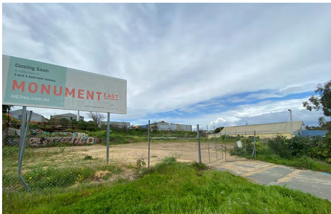
Photo 7: view of No. 34 Amherst Street looking south-east
