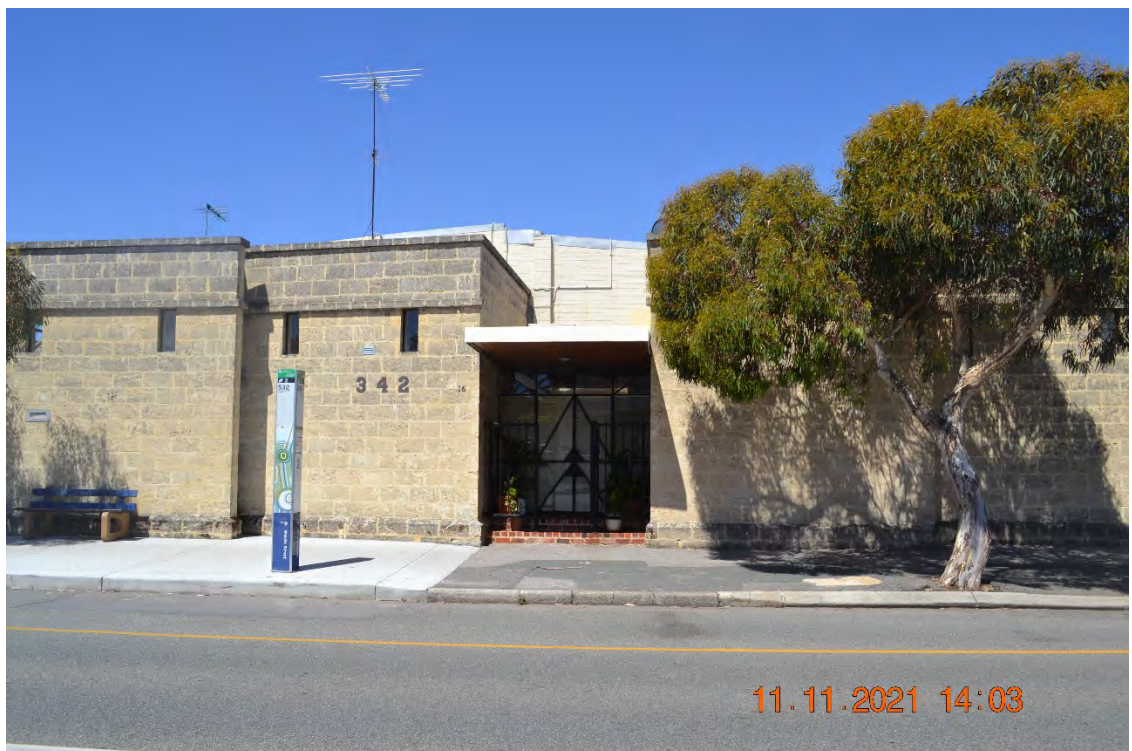
Photo 4: View of opposite side of South Terrace viewed from subject site
