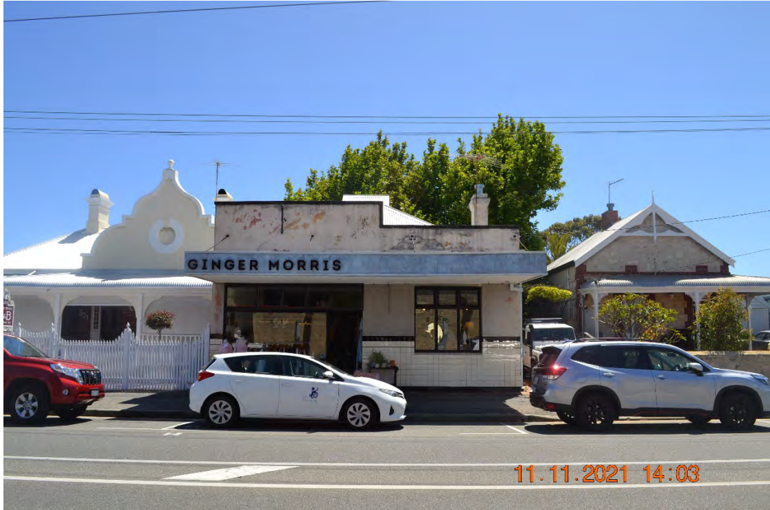
Photo 1: Subject site as viewed from South Terrace
