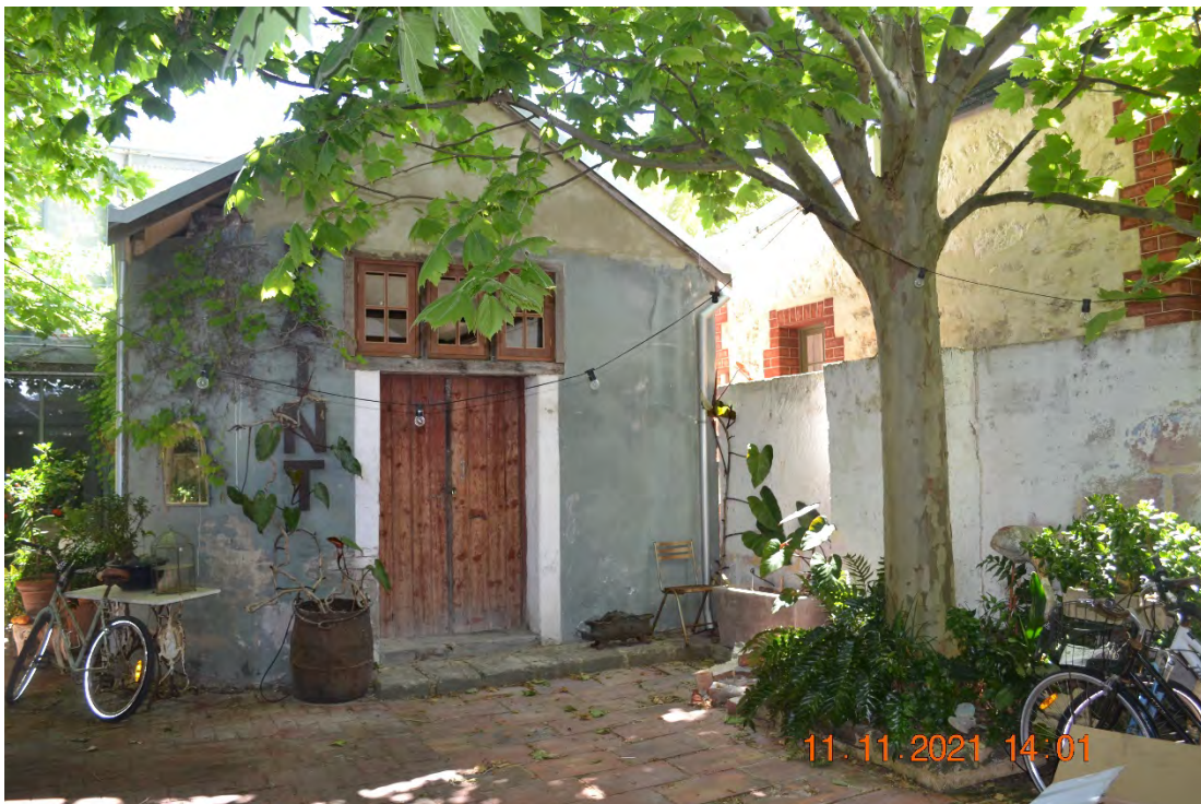
Photo 8: View of Old Bakehouse and neighbouring property from subject site rear courtyard looking north
