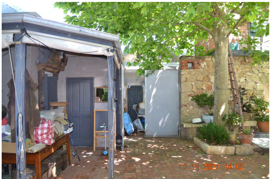
Photo 10: View of rear courtyard looking south where proposed additions are to occur.
