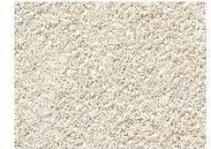
Rendered masonry walls
