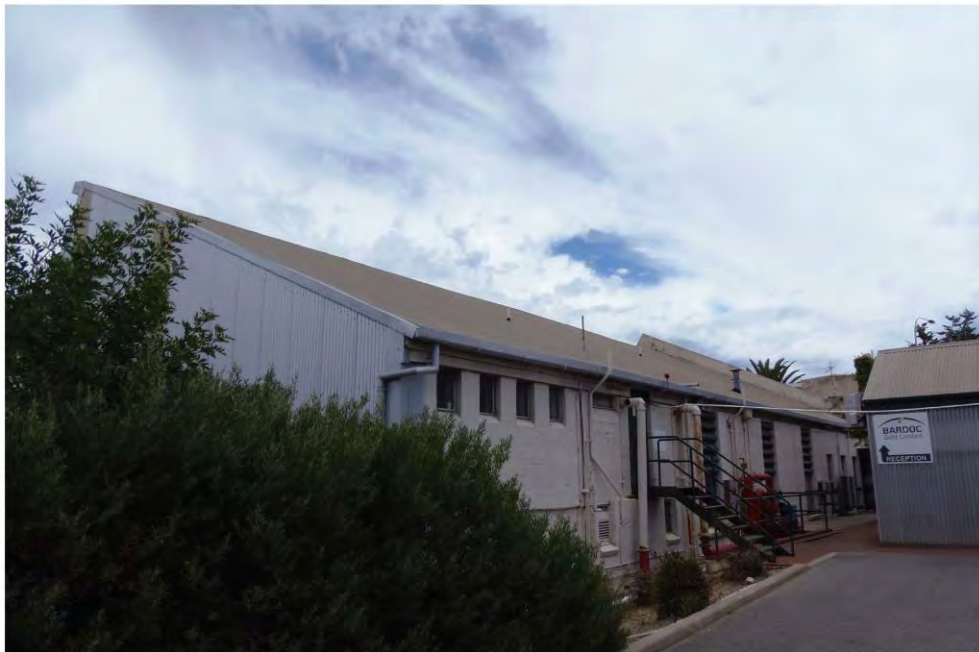
14 North Elevation - Workshop Wing Building: Facade
