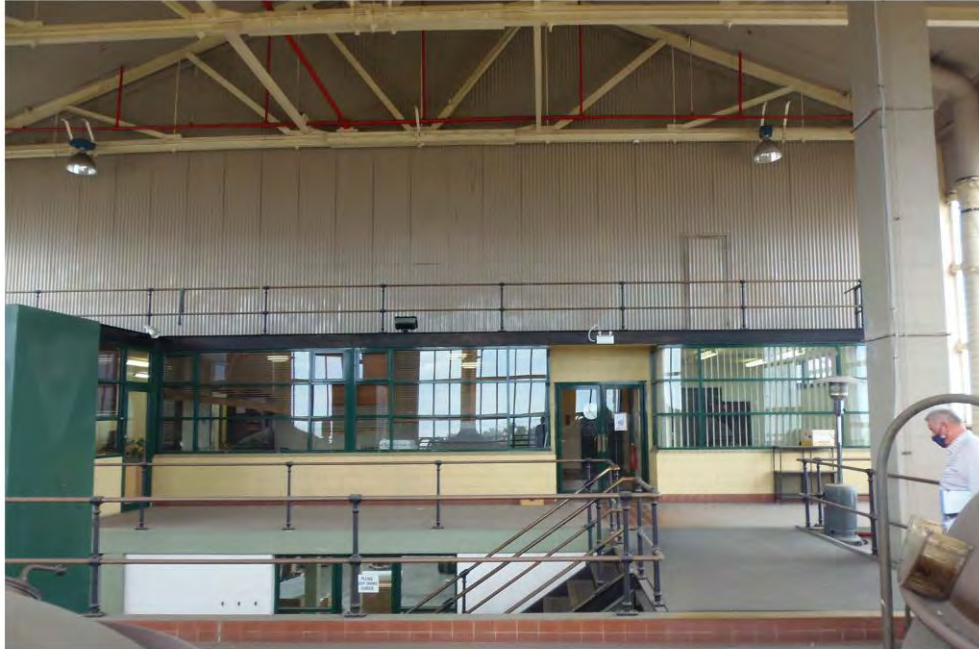
21 Internal - Factory Building: Mezzanine level (Offices)
