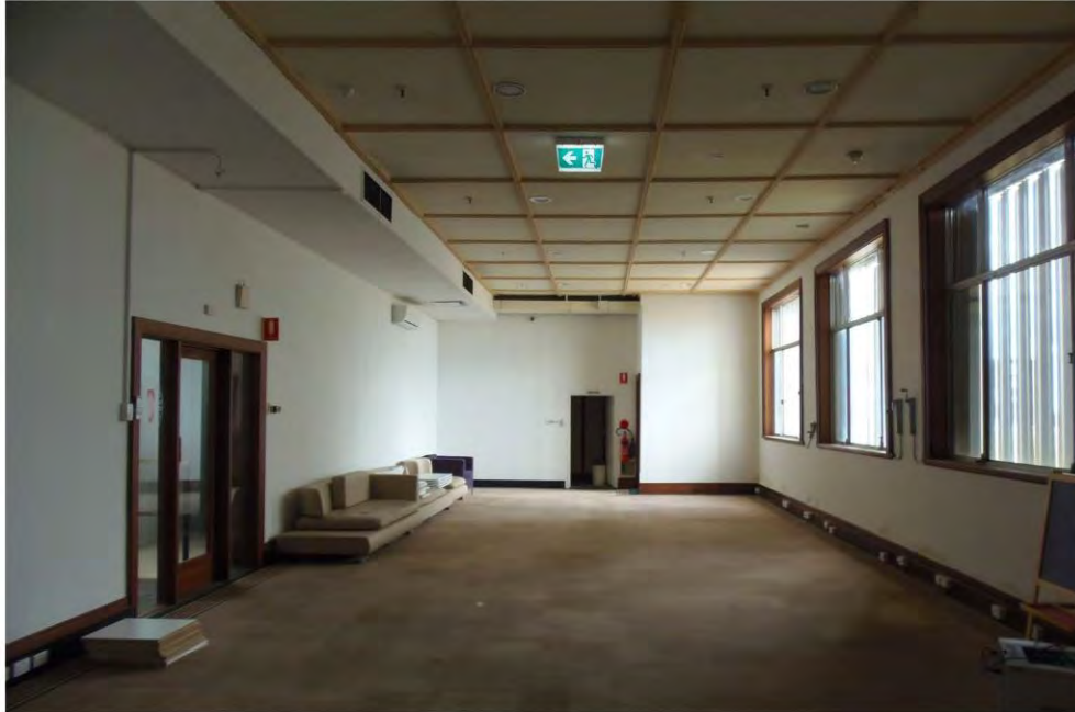
23 Internal - Office Building: Southern End
