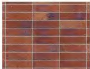
Stack bond red bricks
