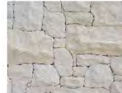
Limestone rubble cladding
