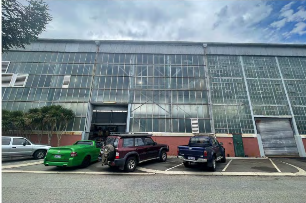
09 South Elevation - Factory Building: Opening 2 + 3
