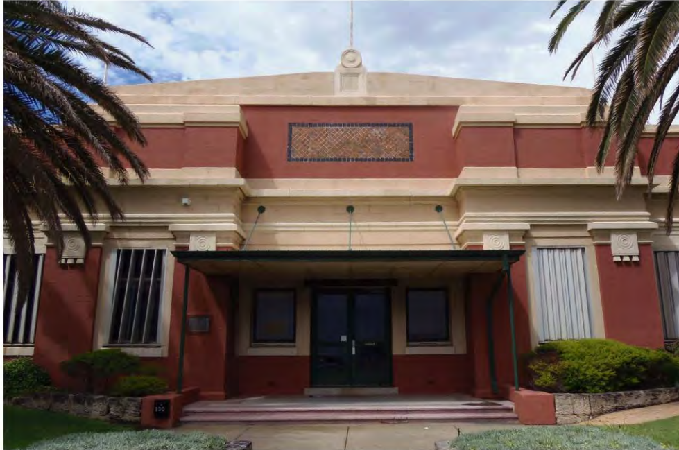
01 West Elevation - Office Buildin: Entrance
