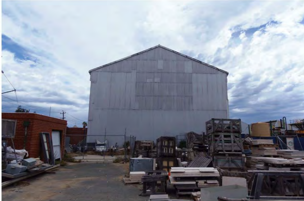
11 East Elevation - Factory Building: Facade
