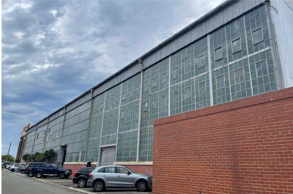
07 South Elevation - Factory Building: 1929 Original + 1947 Addition
