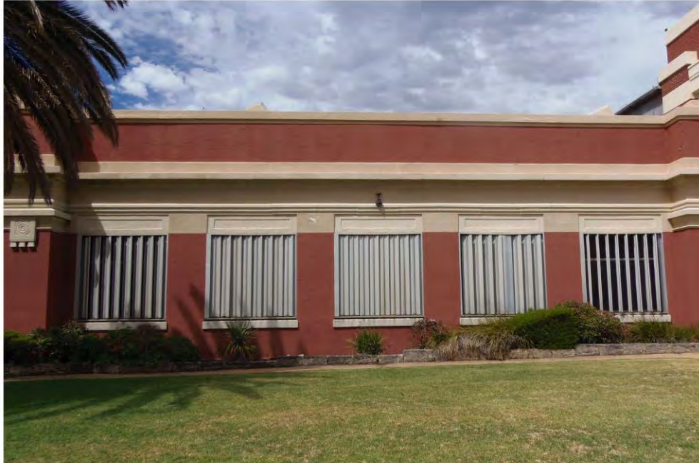
03 West Elevation - Office Building: Bays of aluminium framed windows
