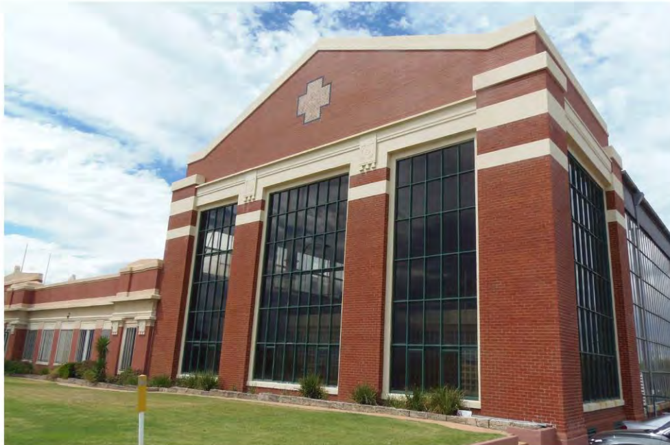
05 West Elevation - Factory Building: Facade
