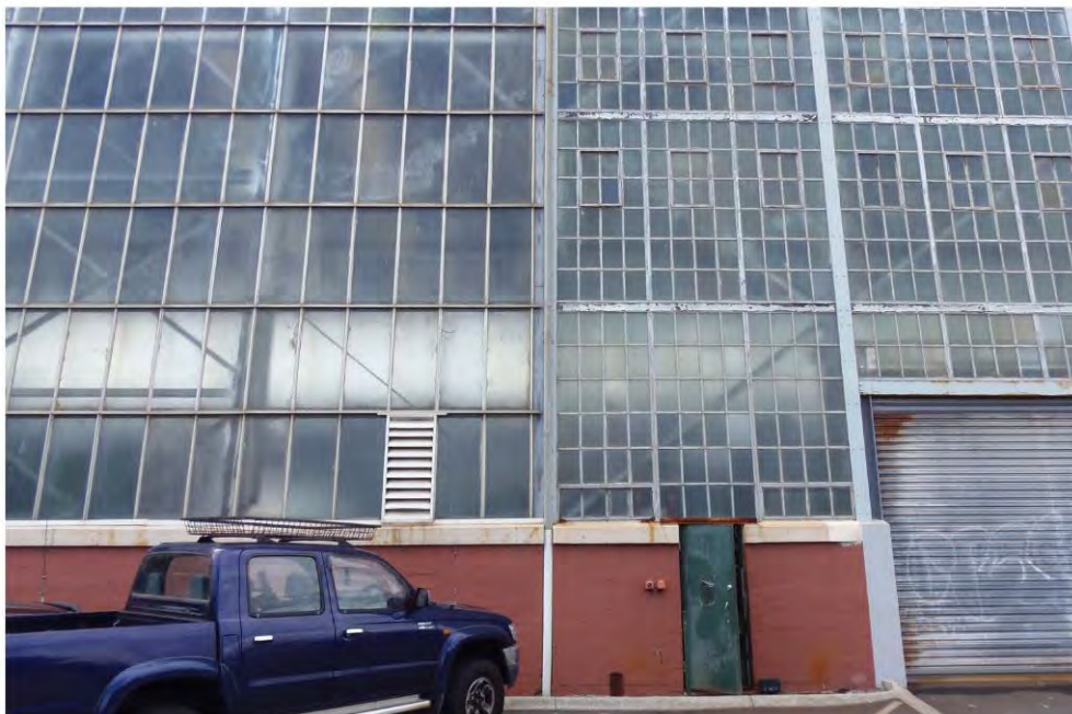
10 South Elevation - Factory Building: Connection 1929 Original to 1947 Addition
