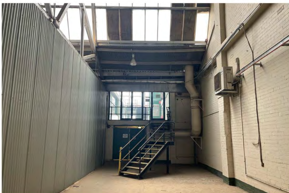
18 Internal - Workshop Wing Building: Connection to Factory Building
