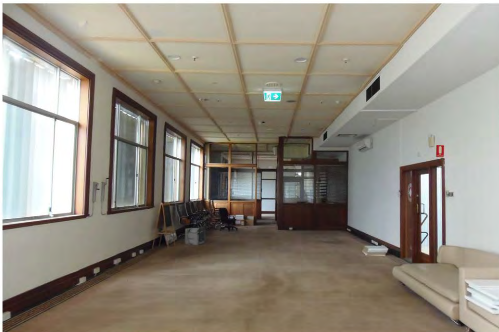
24 Internal - Office Building: Southern End
