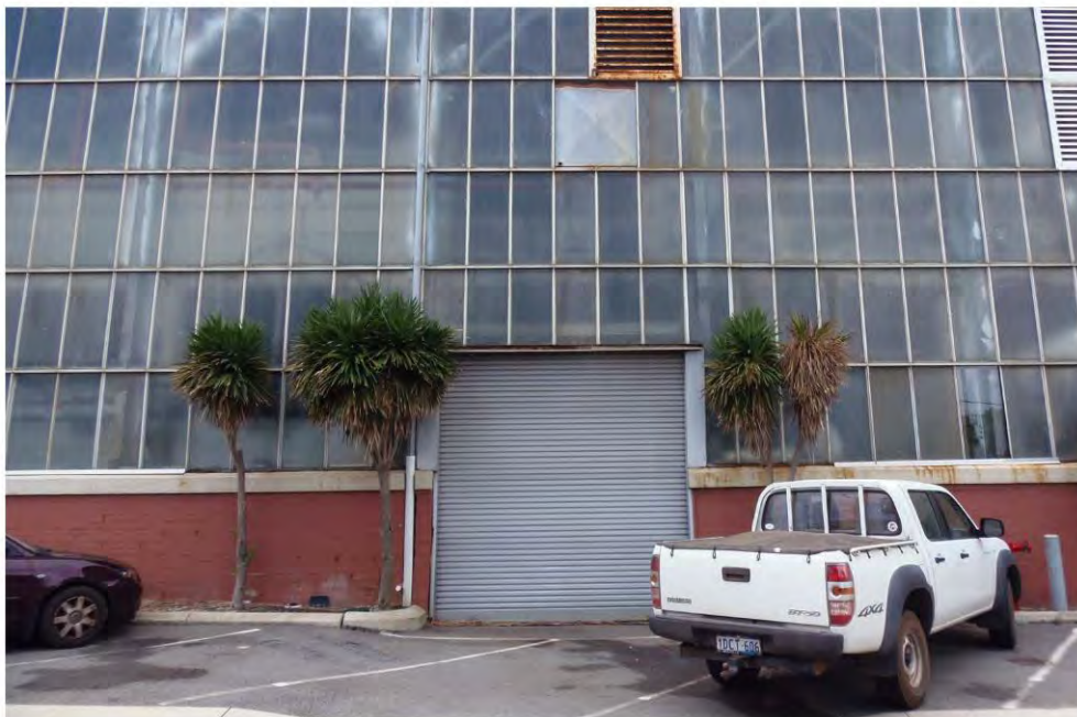
08 South Elevation - Factory Building: Opening 1
