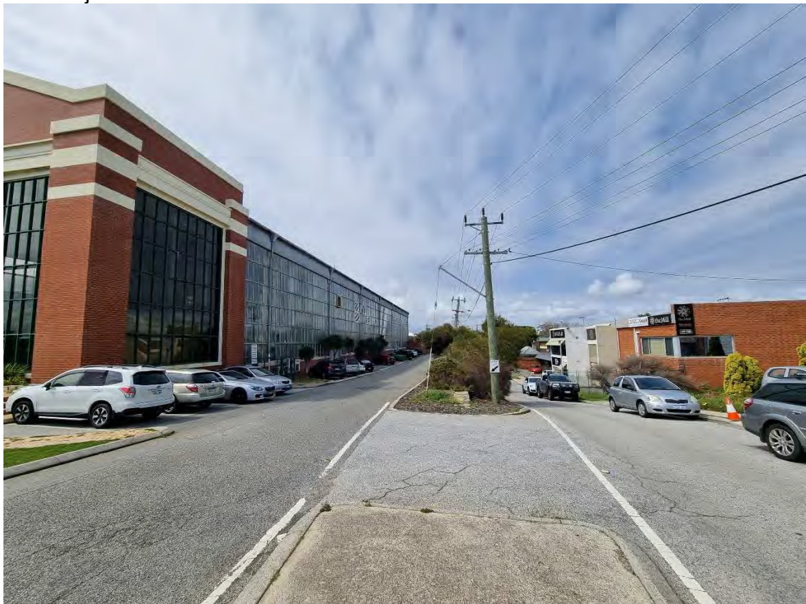
Photos 7 & 8: western and eastern view down Coventry Parade on southern side of subject site
