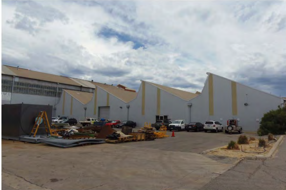
13 East Elevation - Workshop Wing Building: Facade - 'Sawtooth' Roof feature
