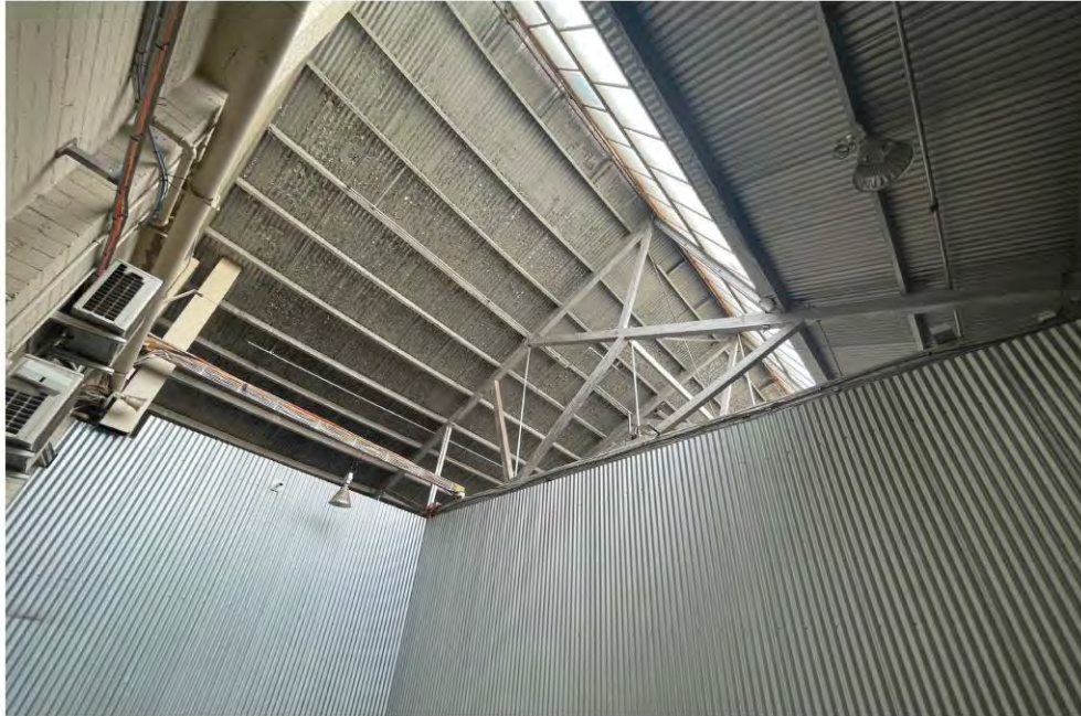
15 Internal - Workshop Wing Building: 'Sawtooth' Roof
