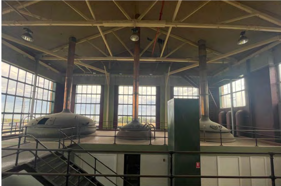
19 Internal - Factory Building: Mezzanine level (Kettles/VATS)
