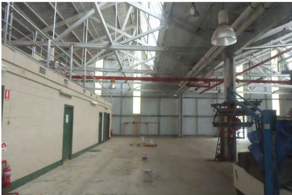
16 Internal - Workshop Wing Building: Interior
