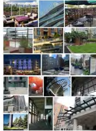
Image 7: Examples of Wind Control Measures
