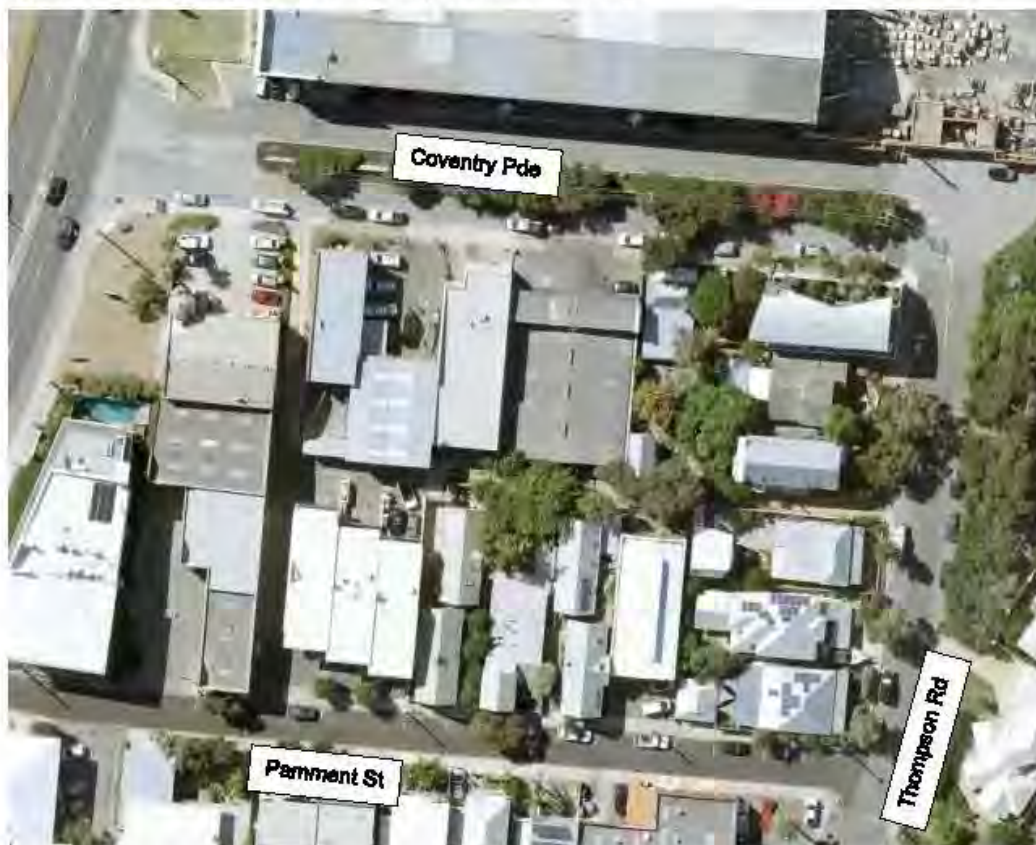
Figure 2-13 Parking Along Coventry Parade, Thompson Road Pamment Street
