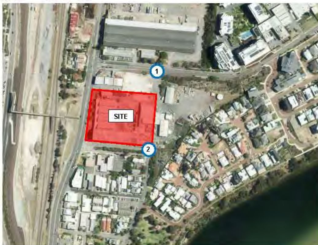
Figure 3-2 Site Access Location
