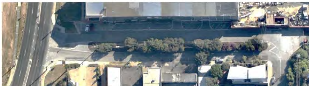
Photograph 2 – Aerial photograph of Coventry Pde east of Stirling Hwy showing existing parking
