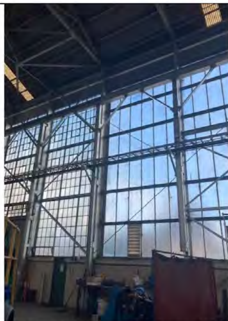
Glazing to south elevation of Factory Wing. Original small pane glazing to 1947 section and replacement glazing to 1929 section.
