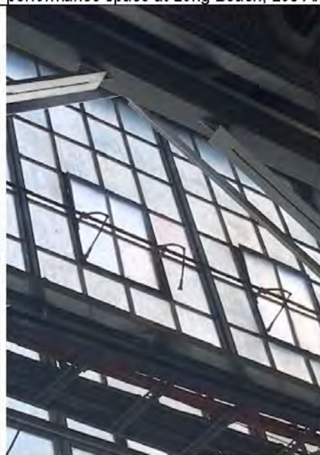
Detail of original small pane glazing to 1947 section of Factory Wing which is proposed for demolition.
