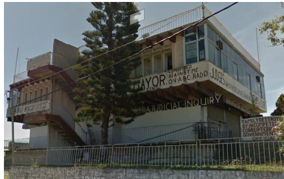
2015 Street View of 20 Moran Street, Google Maps.
