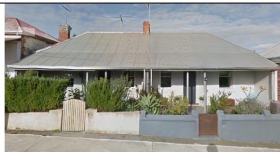
2018 street view of 48 & 50 Lilly Street, Google Maps.
