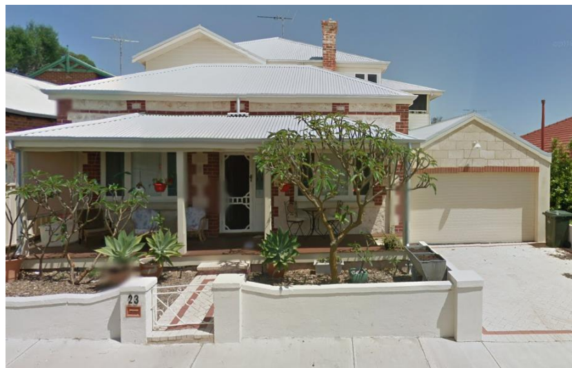
2015 Street View of 23 Martha Street, Google Maps.
