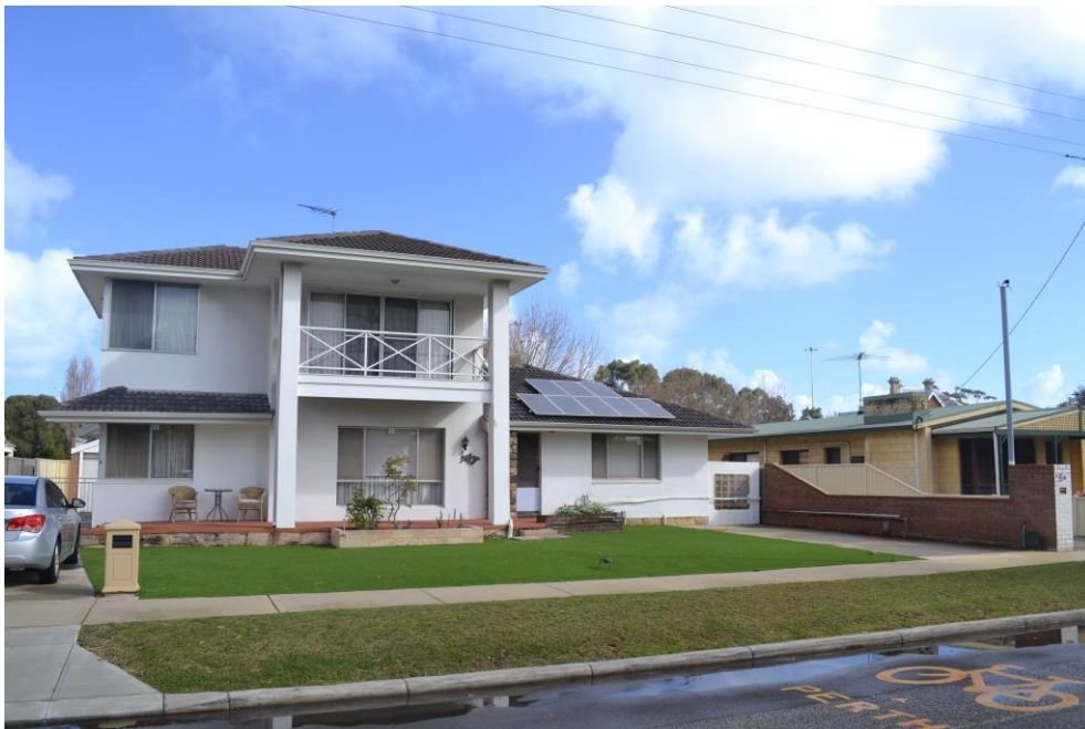
Photo 4: No. 5 Johannah Street with subject site in view.
