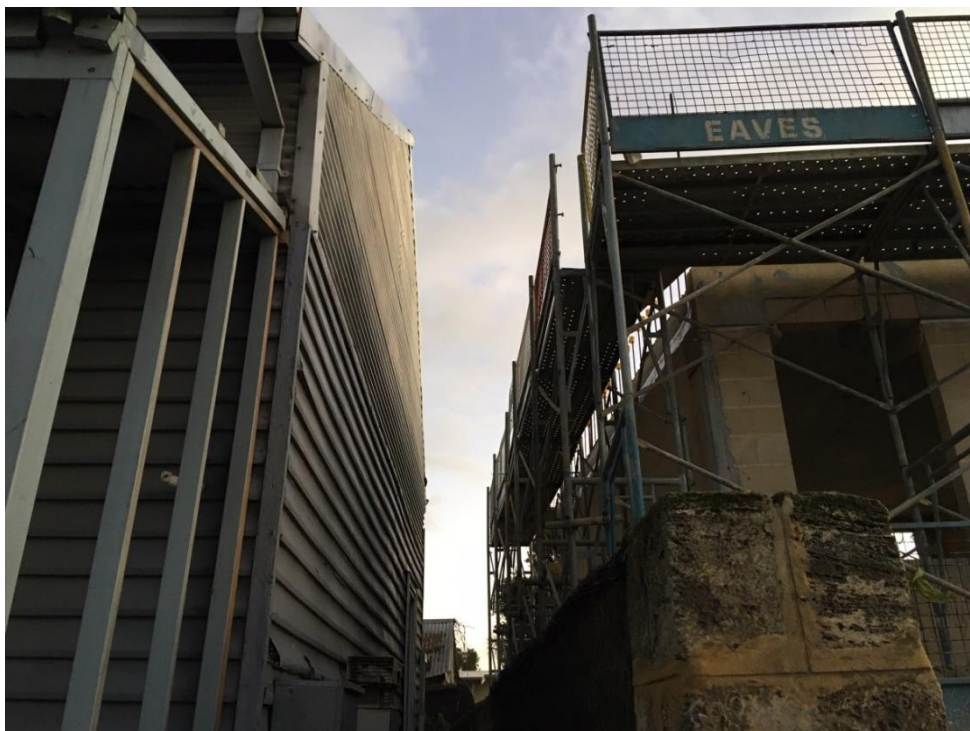
Photo 2: Rear of proposed dwelling and blank gable wall of adjoining house
