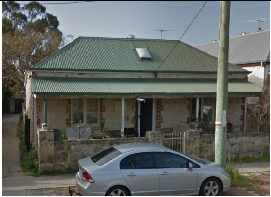
2018 Street View of 62 South Street, Google Maps.
