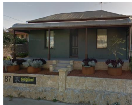
2018 Street View of 1/87 Stirling Highway, Google Maps.
