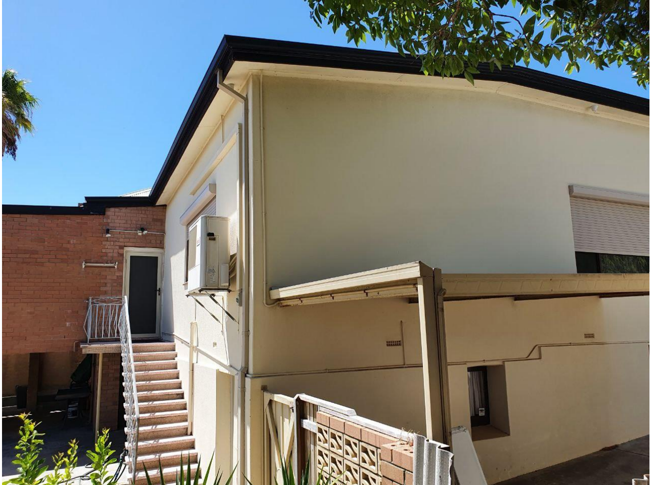
Photo 2: Rear of existing dwelling as viewed from 47 Solomon Street
