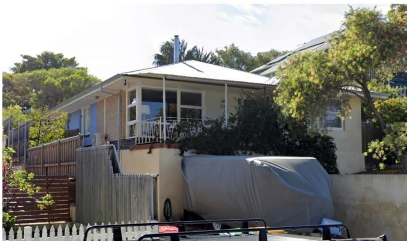
22 Hulbert Street, Google Streetview November 2021
