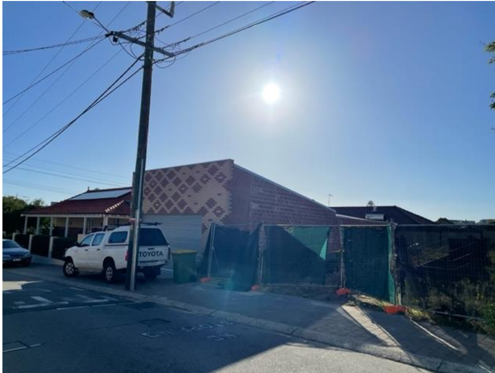
Photo 3: Subject site looking towards No.57 South Street
