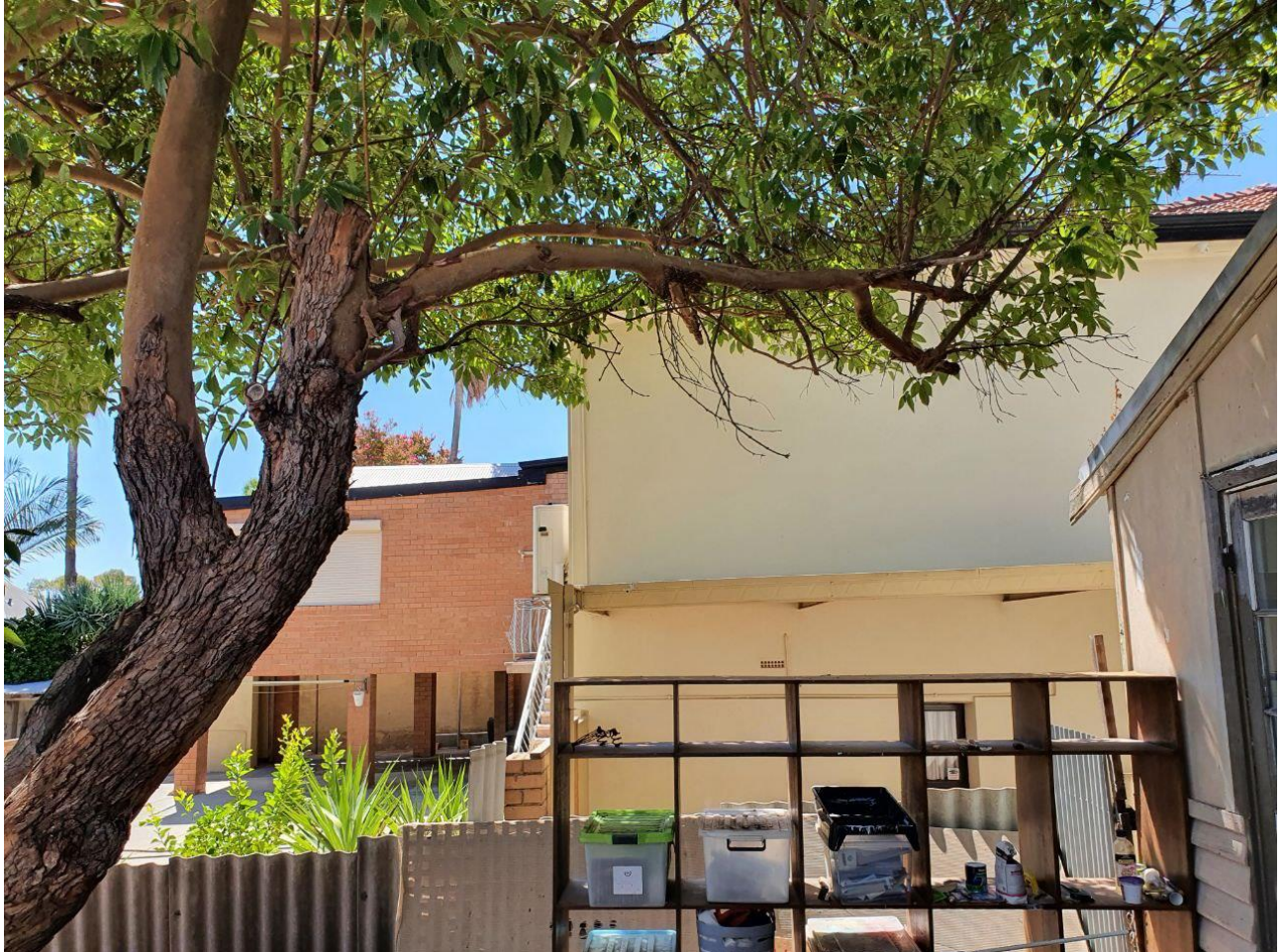
Photo 4: Rear of 45 Solomon Street as viewed from existing rear deck of 47 Solomon Street
