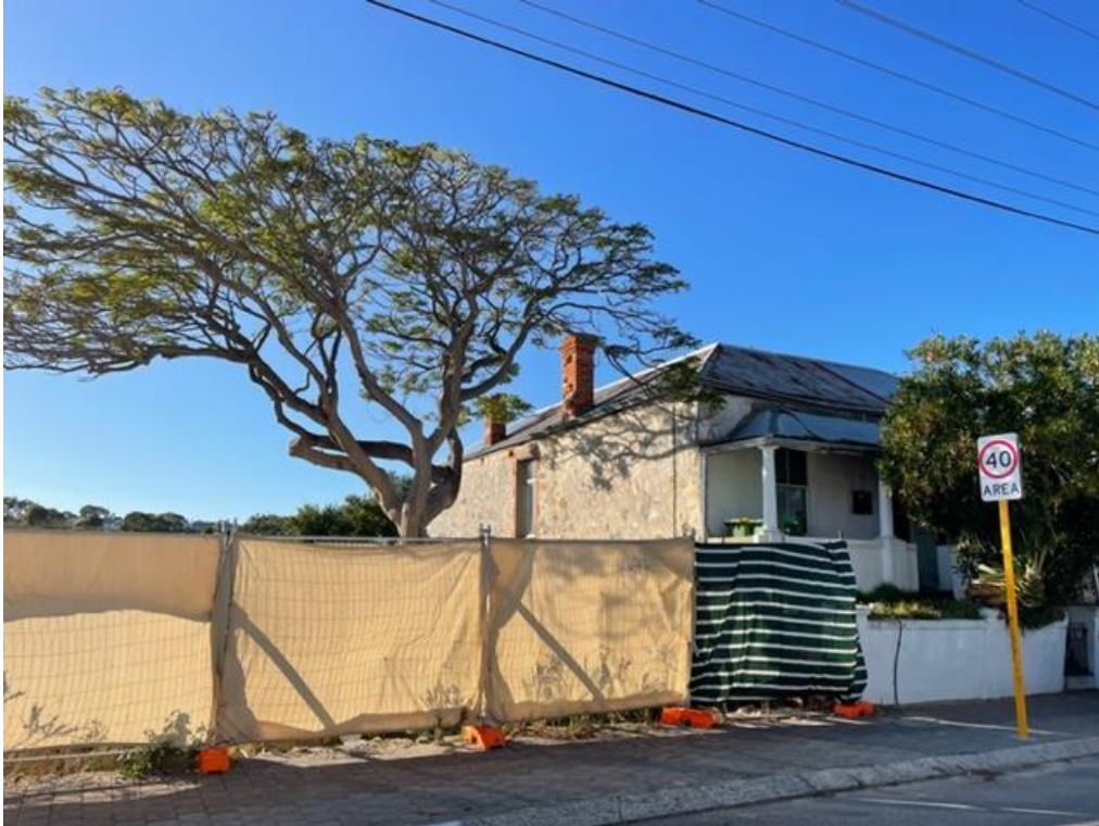
Photo 3: Subject site looking towards No.2 Lilly Street
