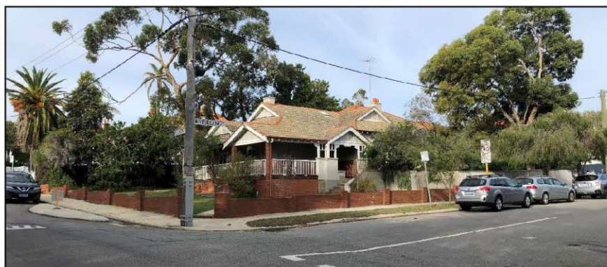
Photograph 2: Wyn Carr House (subject site) viewed from corner of Ellen Street / Stirling Street, looking south-east.
