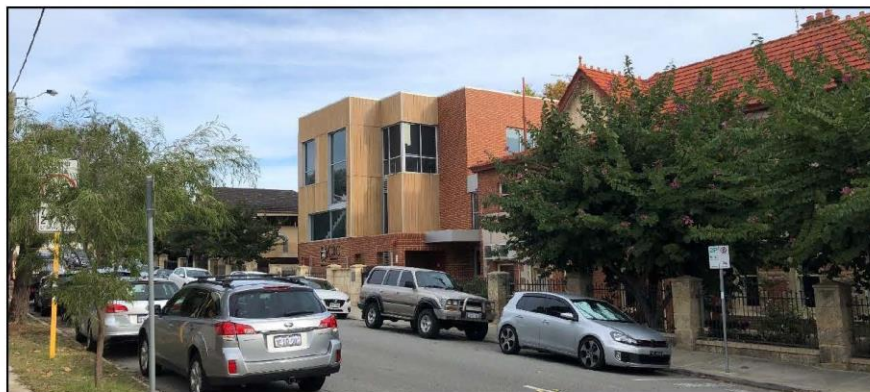
Photograph 5: Christian Brothers College, Stirling Street frontage, viewed from subject site looking south-west.
