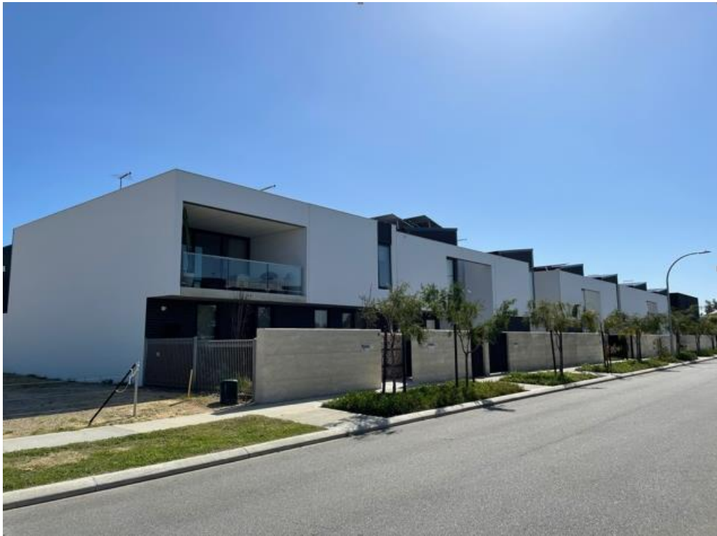
Photo 3: Existing development on Rochfort Way
