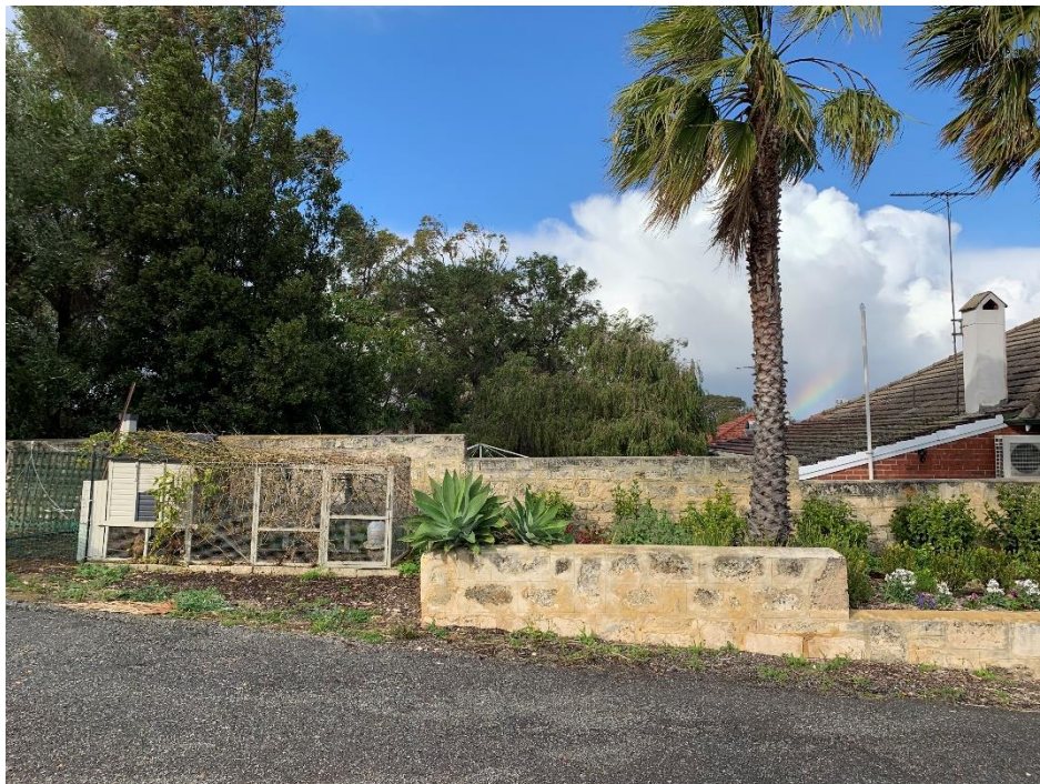
Photo 2: South elevation towards south-western lot. Location of proposed balcony located approximately at the leftmost kink in the dividing fence.
