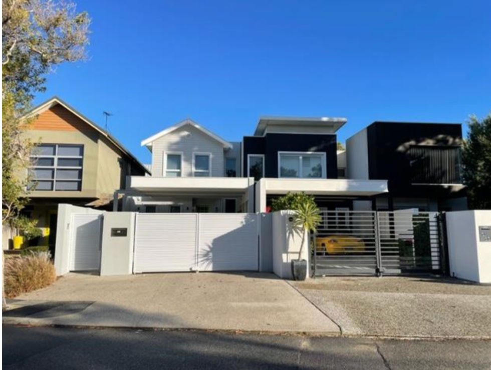
Photo 3: Existing carport structures at 5/86 and 6/86 Thompson Road
