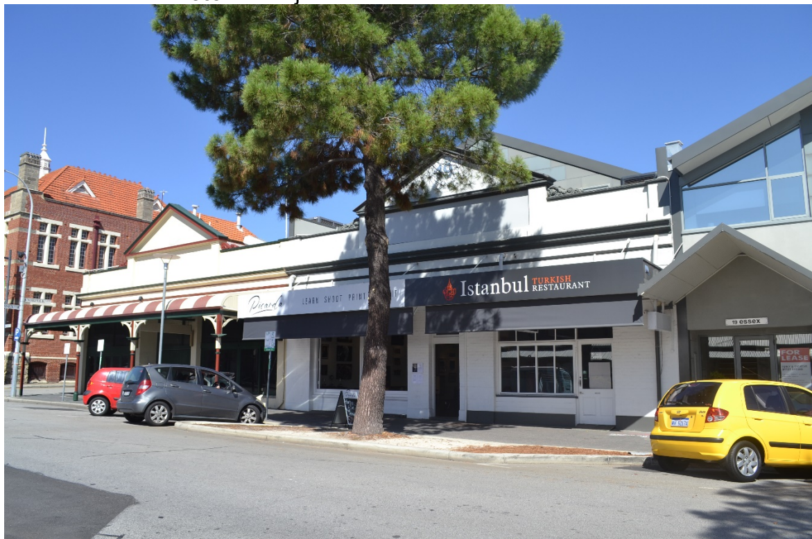
Photo 2: Northern portion of subject site and No. 21 Essex St and Fremantle Technical College to left side of image.
