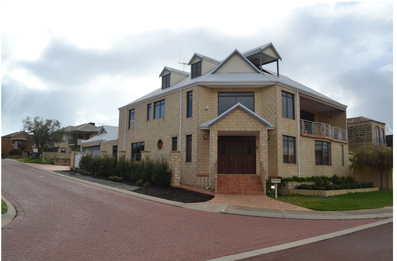
Photo 4: Entrance to Keel Place
