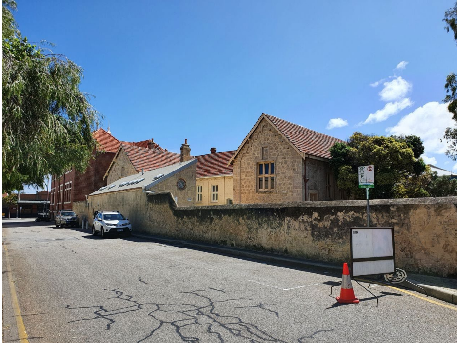
Photo 1 – Site from Norfolk Lane
