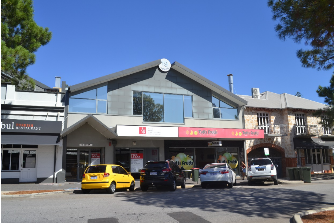
Photo 1: Subject site as viewed from Essex Street
