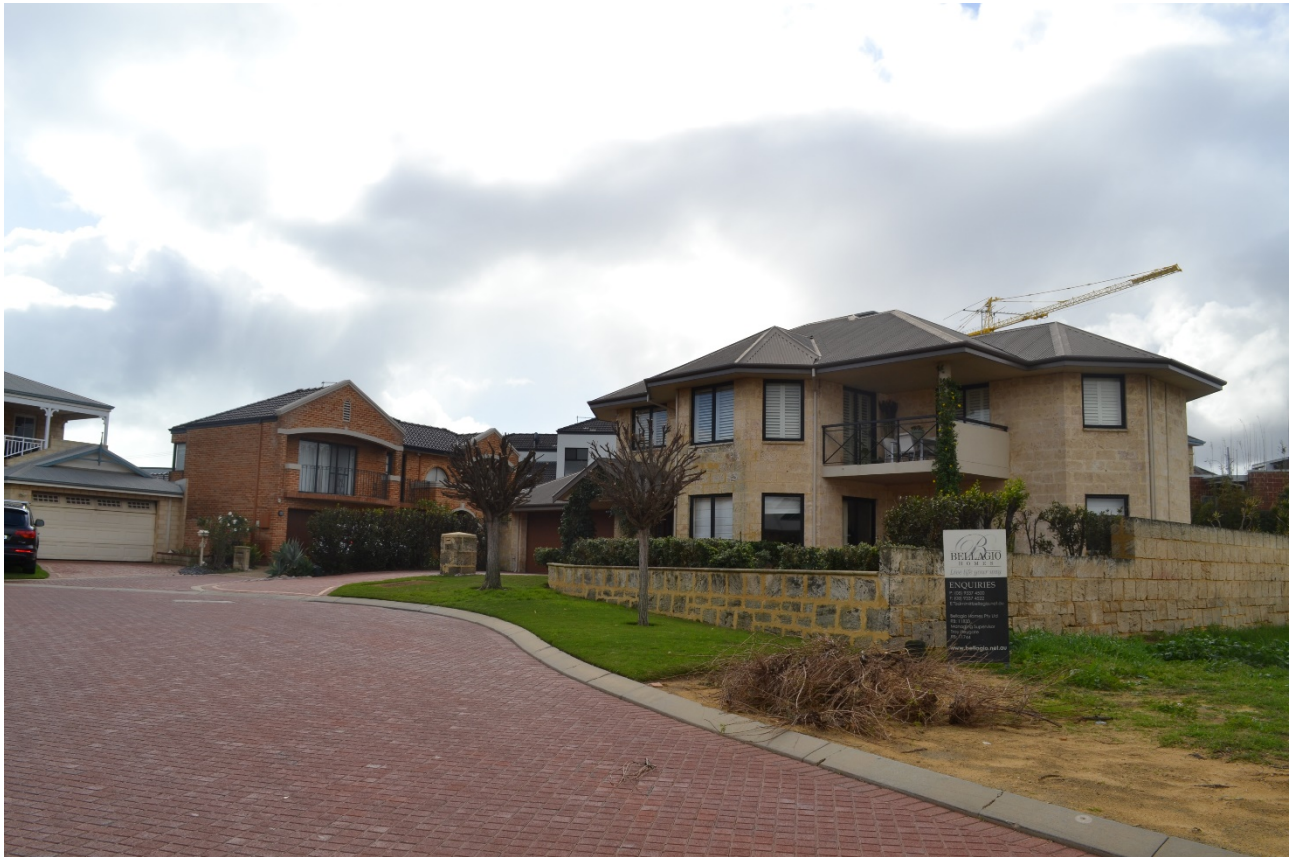
Photo 6: Existing streetscape of Keel Place
