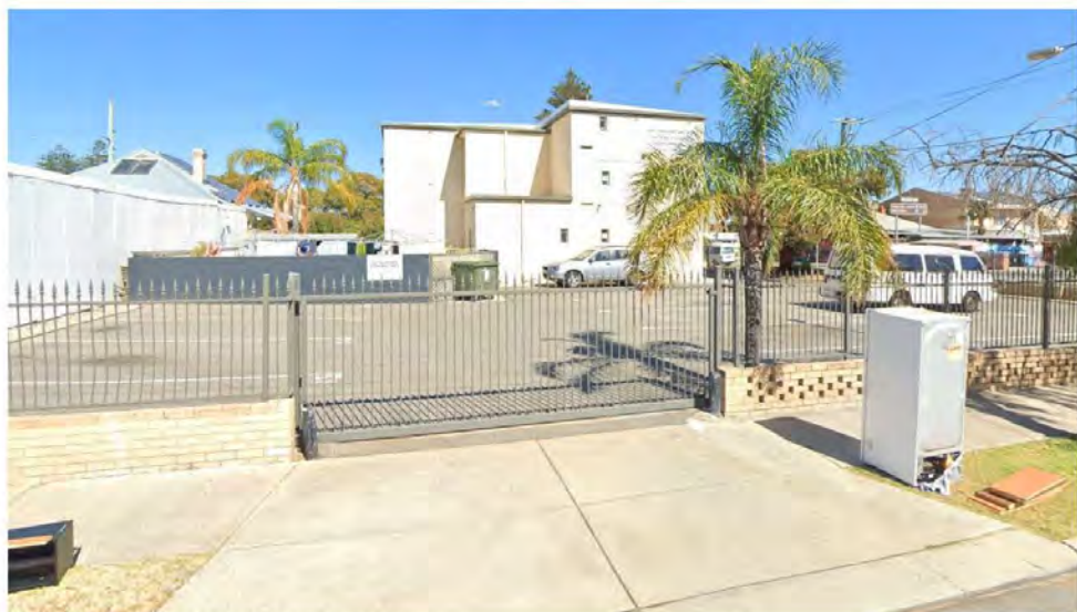
1 Douro road (view from Hickory street)
