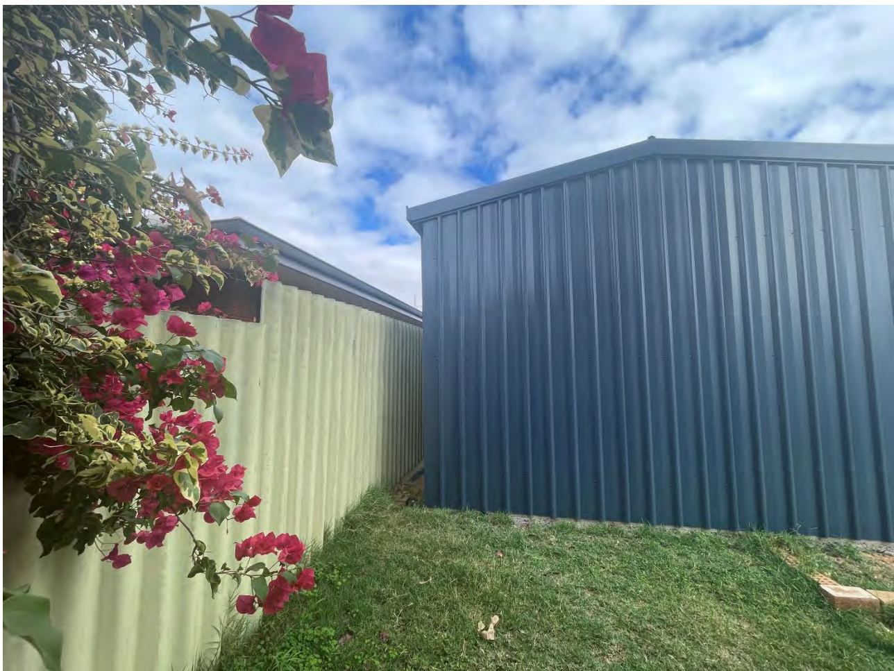
Photo 4: Outbuilding addition view South east towards adjoining property – showing height above boundary fence and rear of outbuilding
