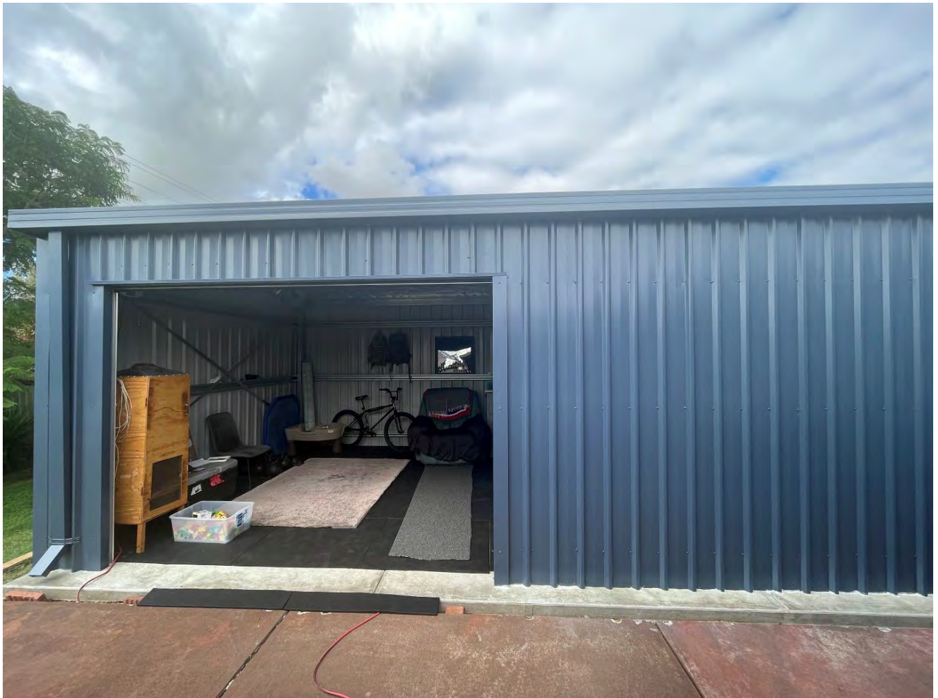
Photo 3: Outbuilding addition view East towards adjoining property
