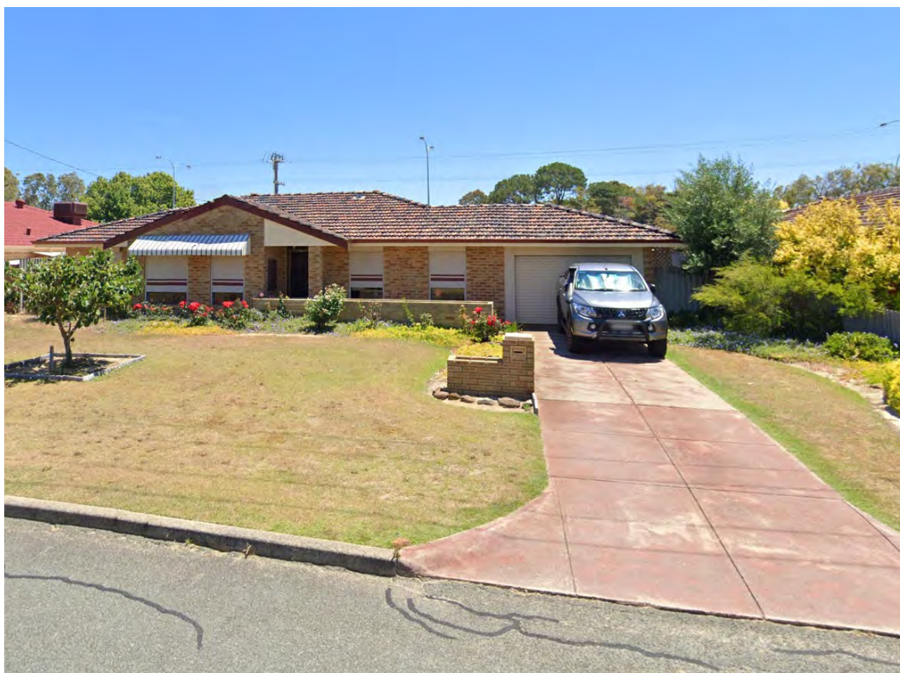
Photo 1: Subject site as viewed from Bradbury Way (Google Maps).
