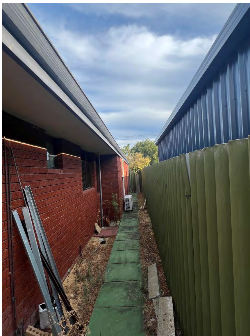
Photo 6: View from Eastern adjoining property – showing rooms adjacent to unauthorised outbuilding addition
