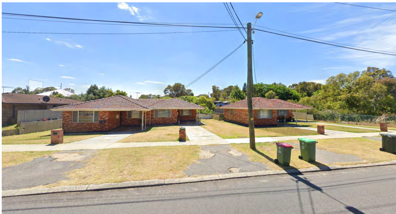
Photo 1: Subject site as viewed from Edmund Street
