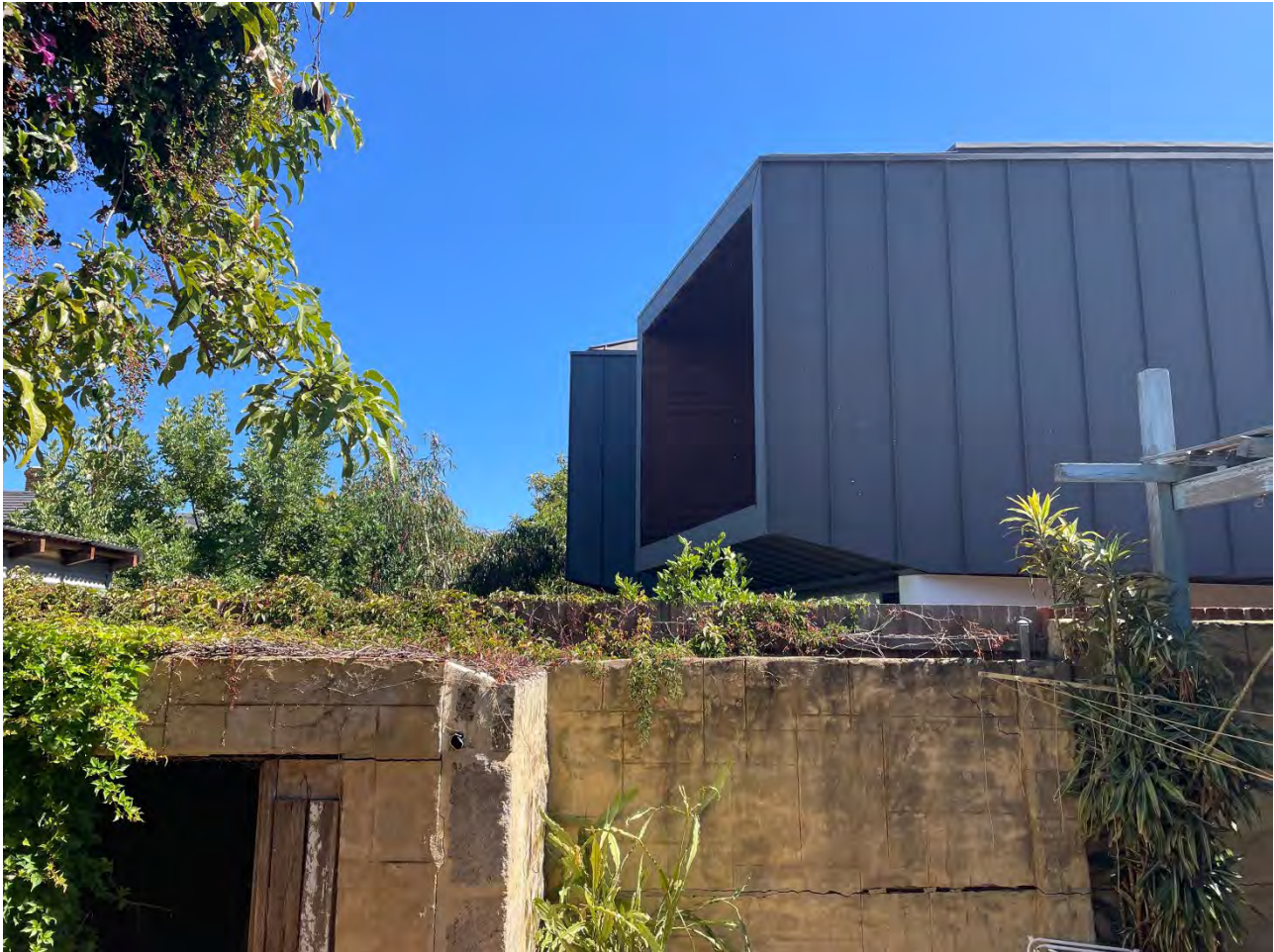
Photo 5: Adjoining properties to the North (27A Swanbourne Street) – extent of rear extension
