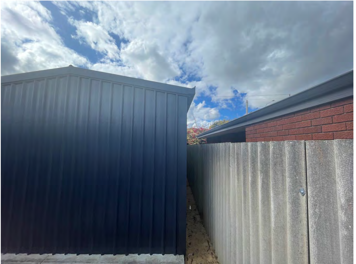
Photo 2: Outbuilding Addition view North – showing height above existing boundary fence
