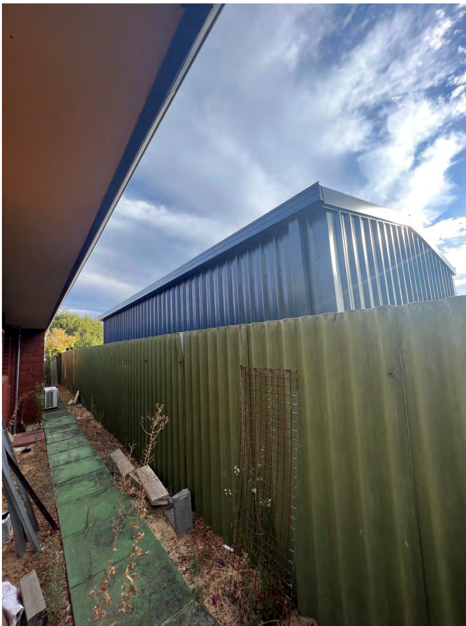
Photo 5: Outbuilding addition view from Eastern adjoining property – showing height above boundary fence and rear of outbuilding
