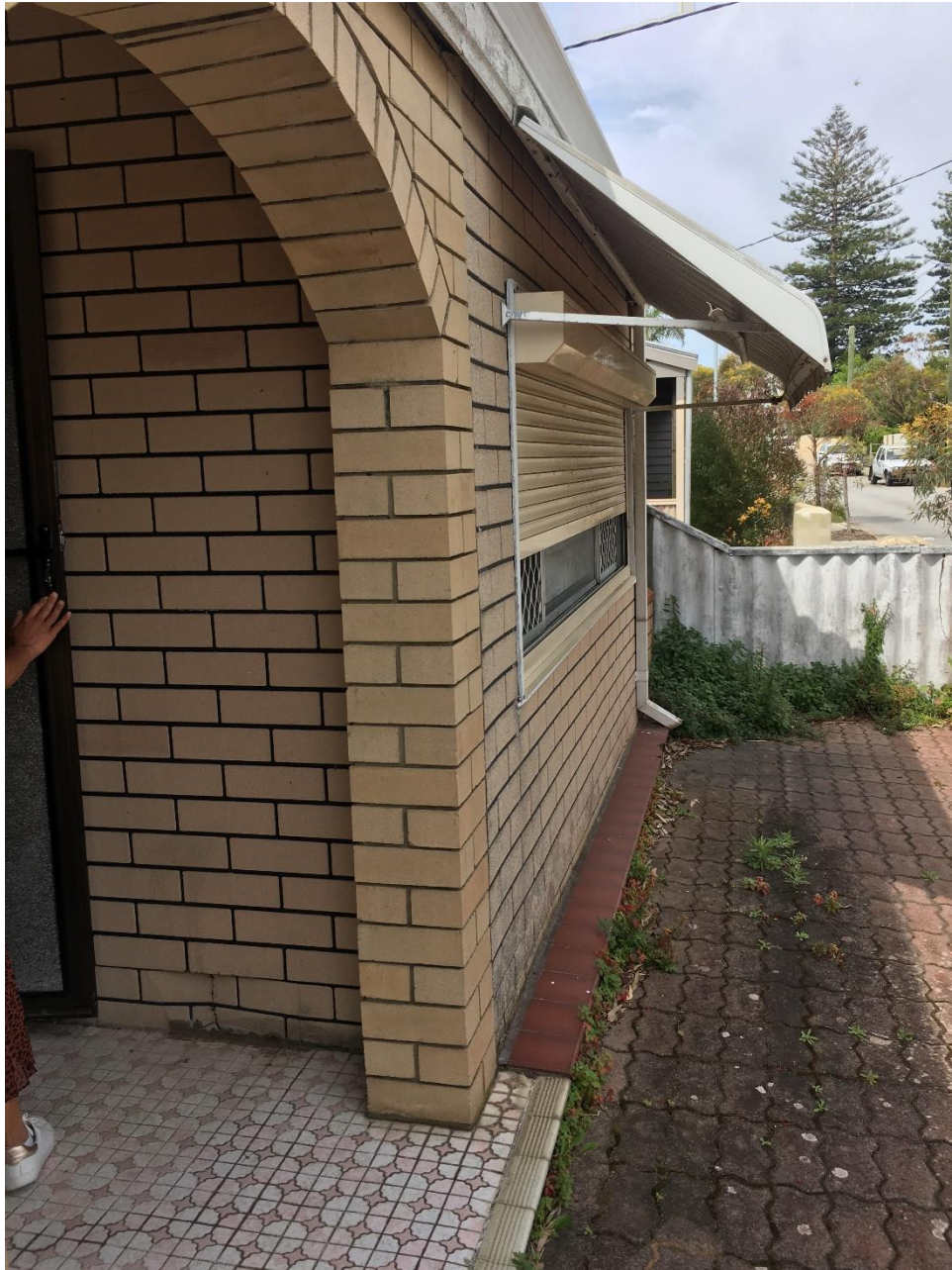
Front verandah with concrete and tiles floor, brick columns and faux brick cladding to walls and infilled verandah section
