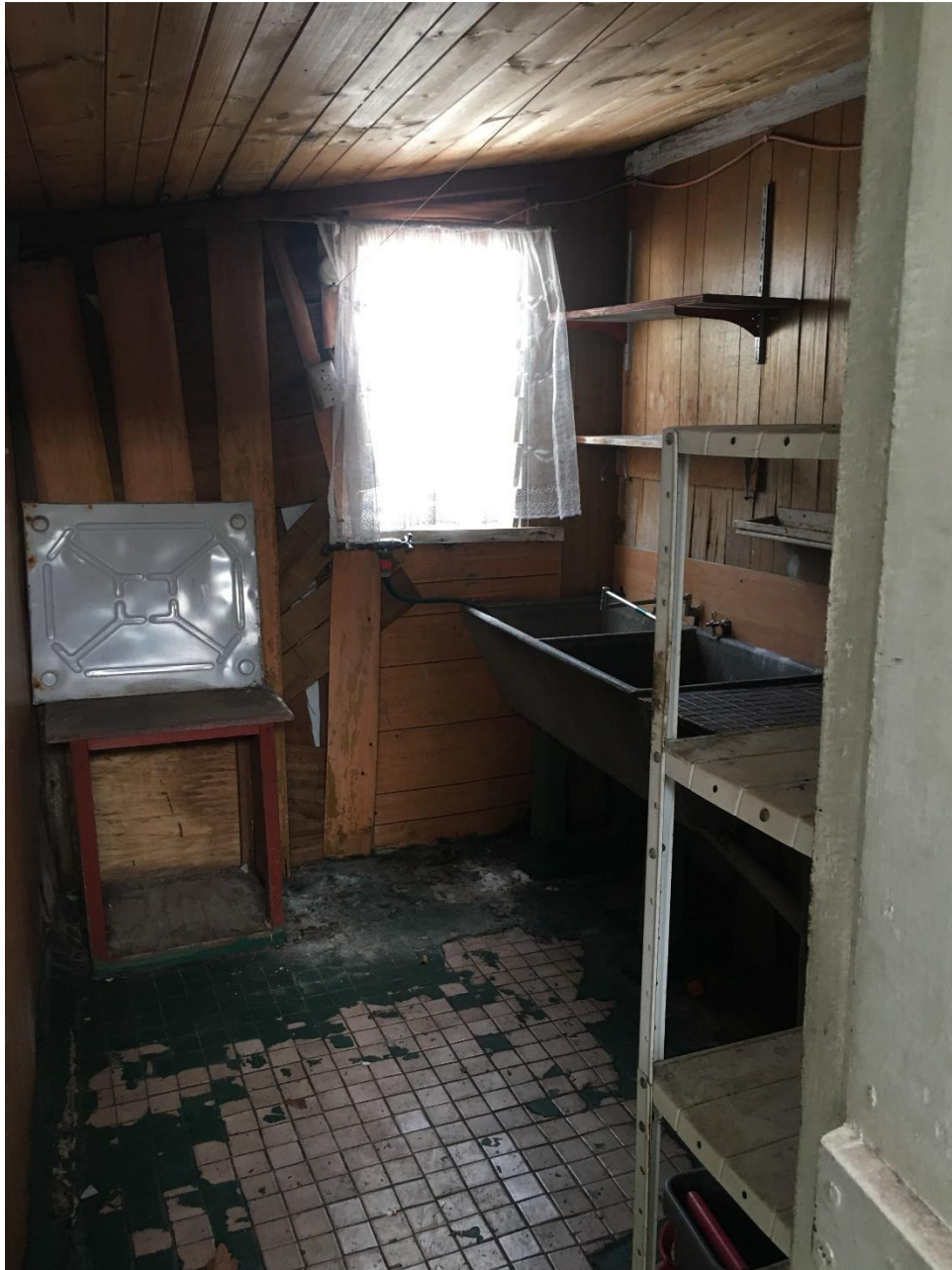
Laundry in rear skillion
