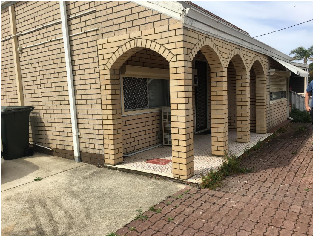
Front verandah with concrete and tiles floor, brick columns and faux brick cladding to walls and infilled verandah section
