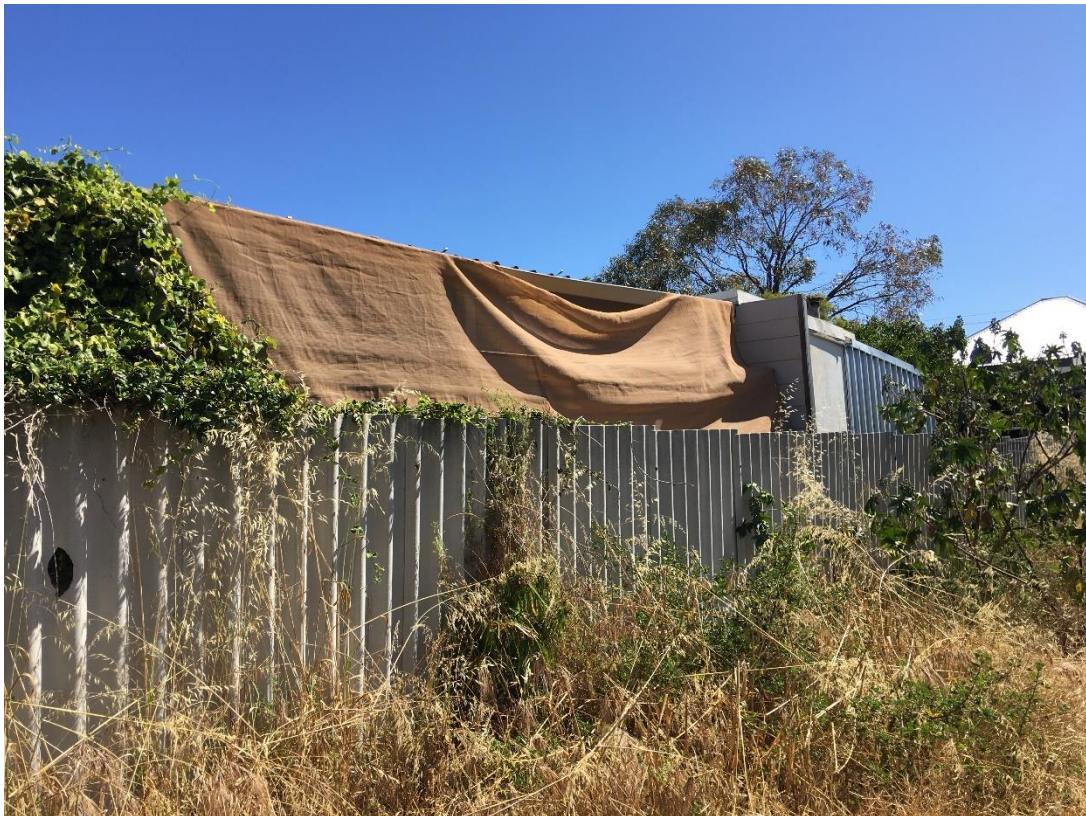
Photo 2: West elevation of site showing adjoining existing outbuilding
