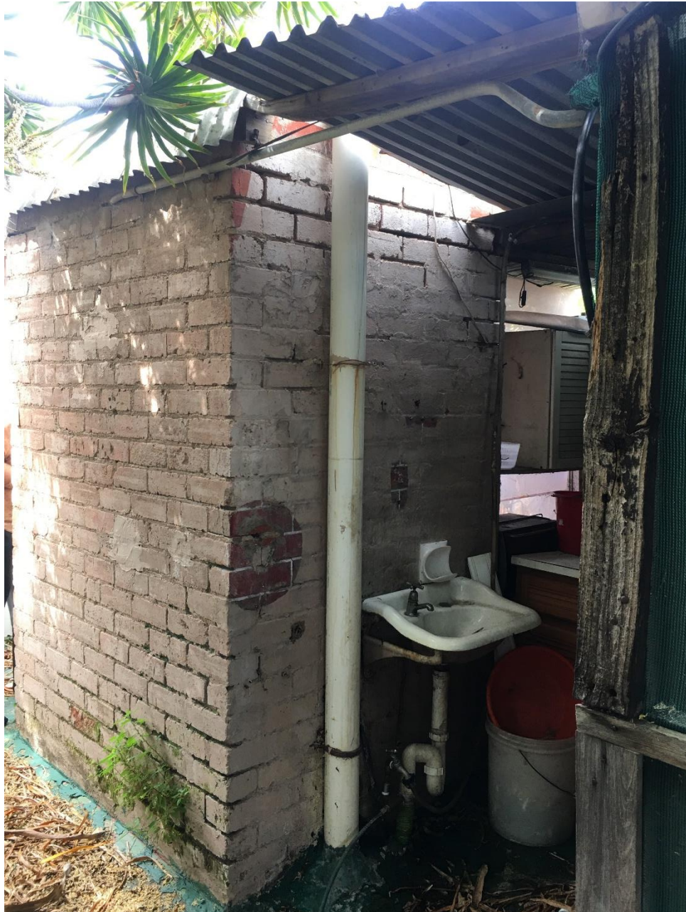
Rear brick WC
