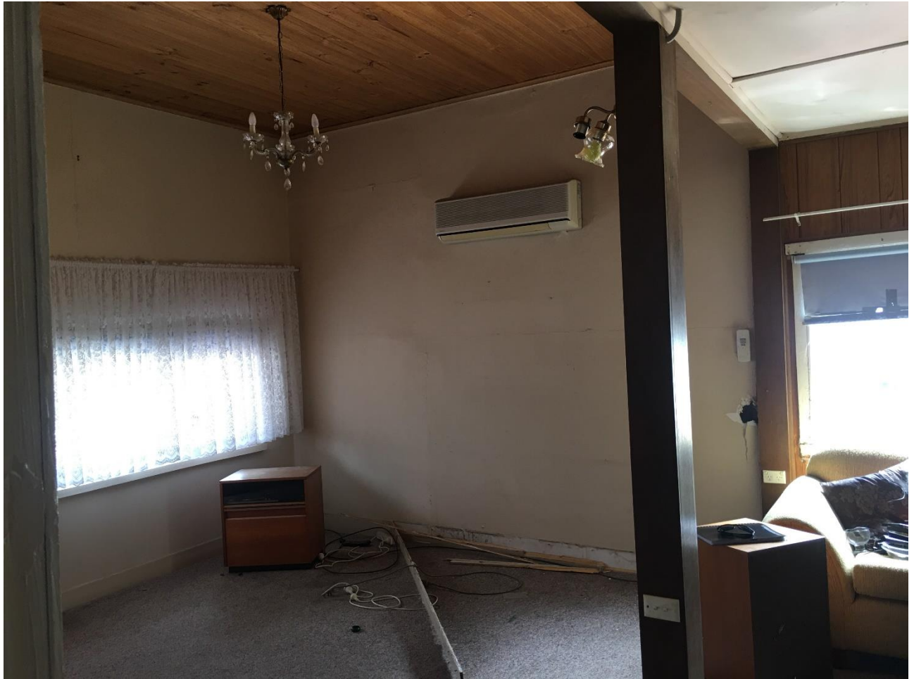
Front room under main hipped roof
