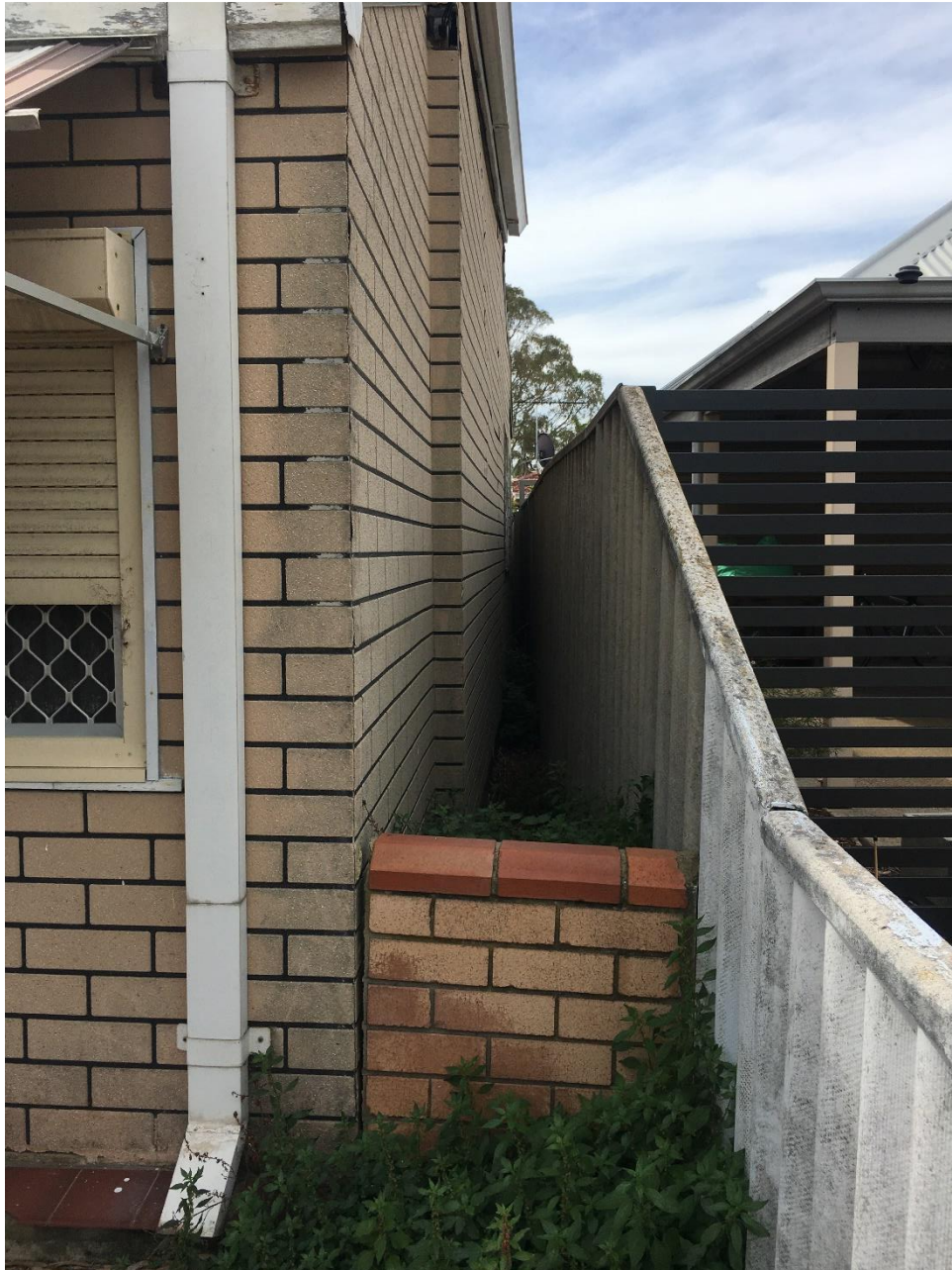
Boundary between 6 and 8 Commercial Street
