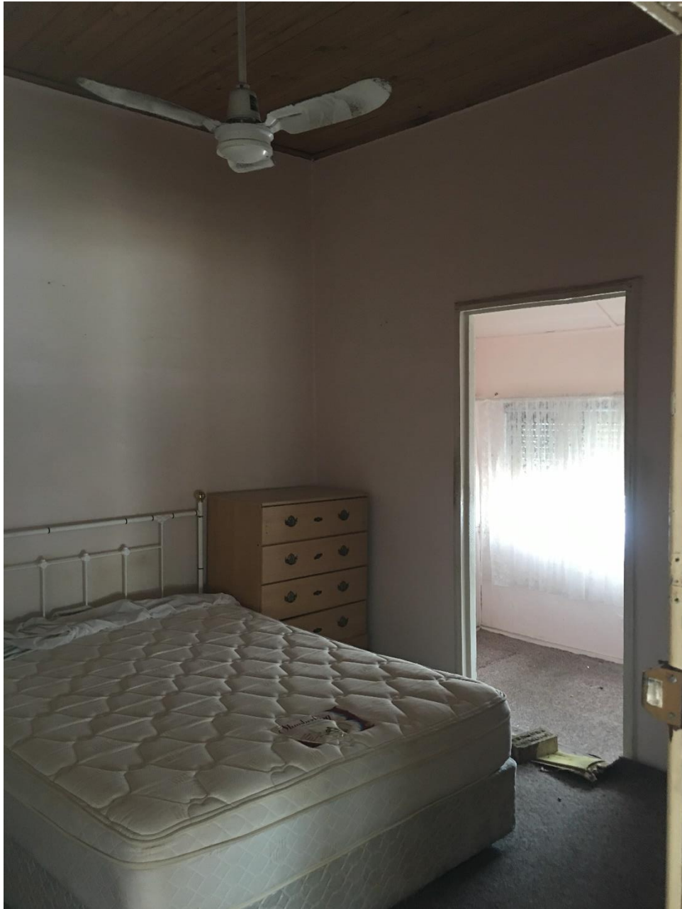
Front Bedroom – under main hipped roof – looking through to enclosed verandah
