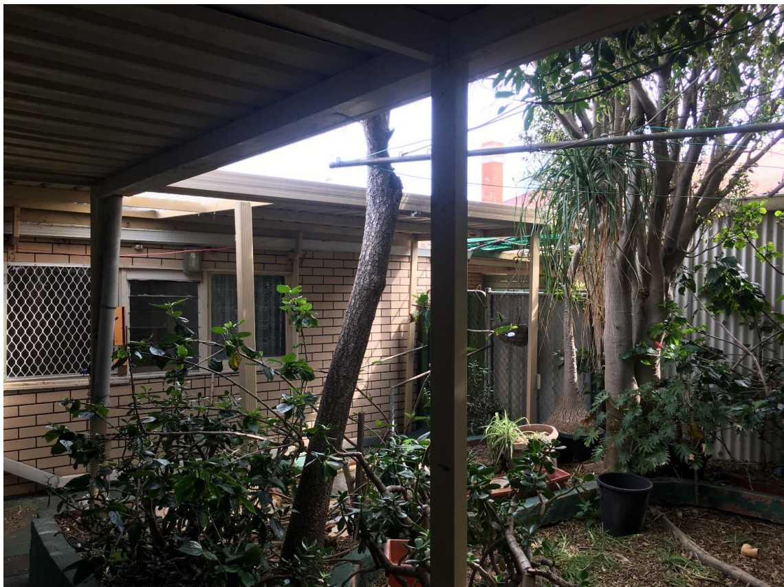
Rear Garden adhoc additions
