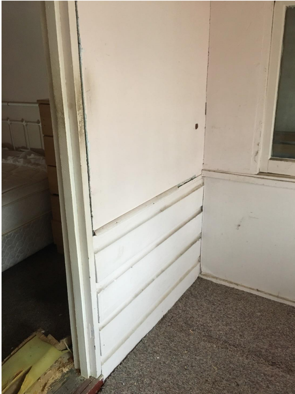
Enclosed front verandah room – with original or early weatherboards
