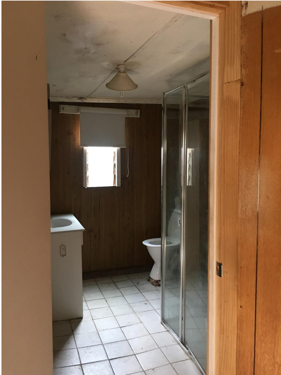
Bathroom under rear skillion
