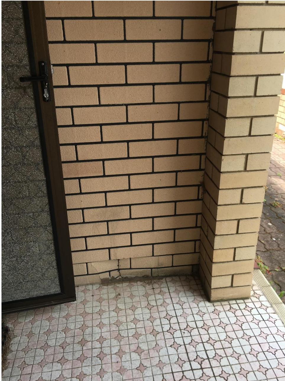
Front verandah with concrete and tiles floor, brick columns and faux brick cladding to walls
