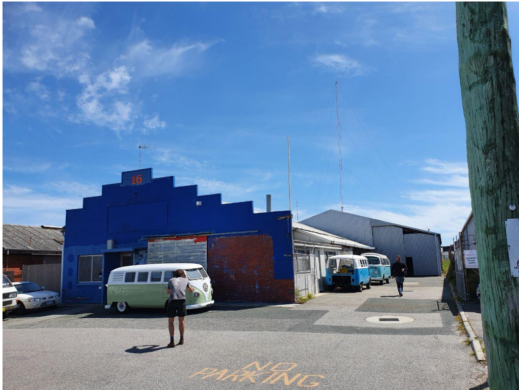
Photo 1: Building frontage and side access
