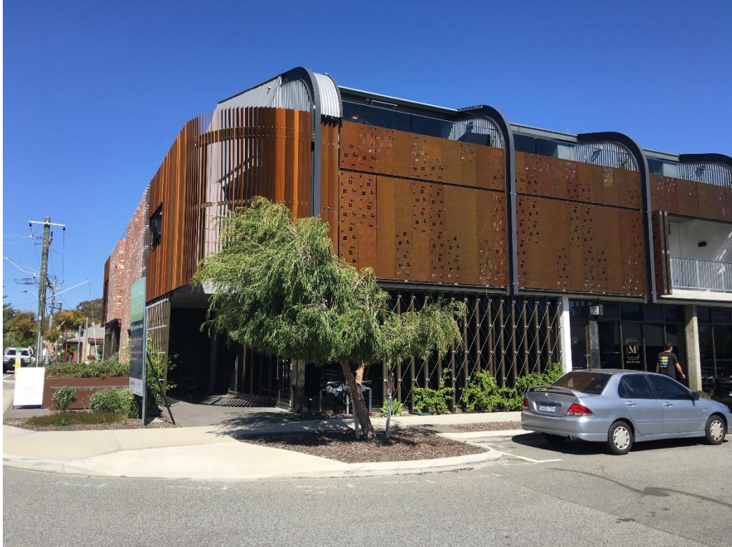
Photo 1: Douro Road and Hulbert Street intersection elevation
