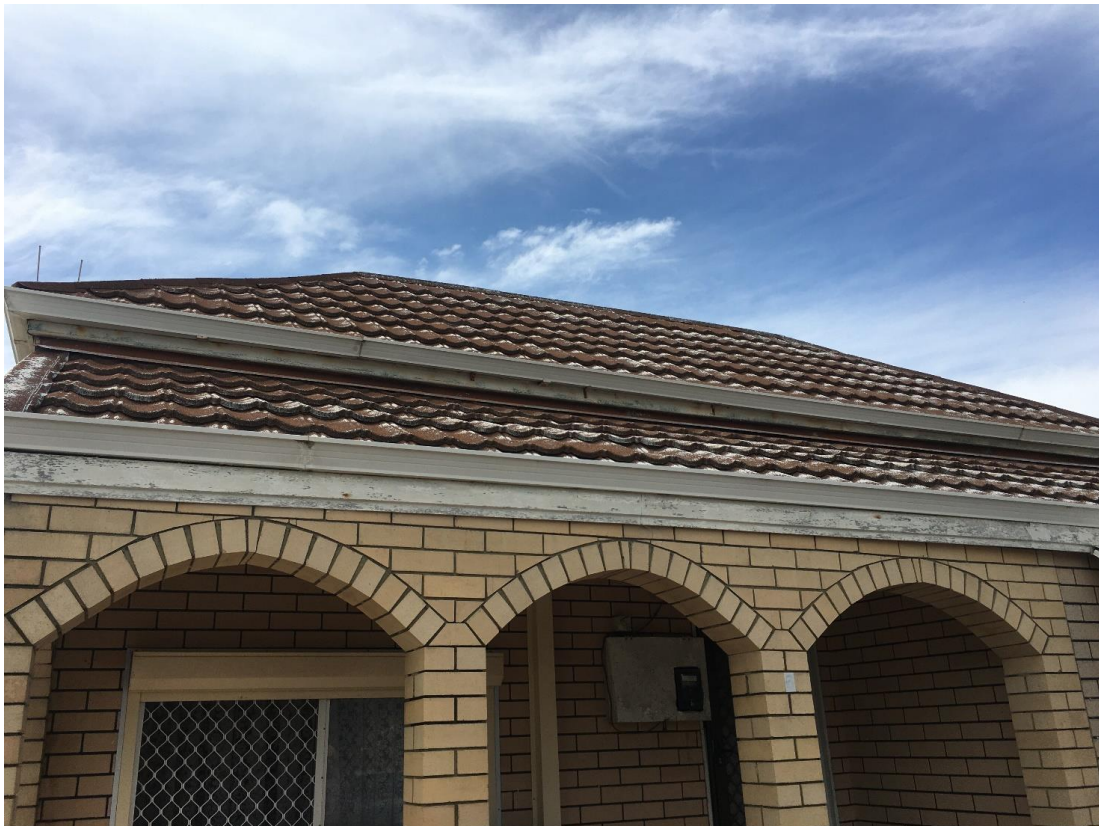
Front verandah with brick columns and faux brick cladding to walls – evidence of weatherboards behind this section of faux brick cladding exists. Decramastic pressed metal roofing.
