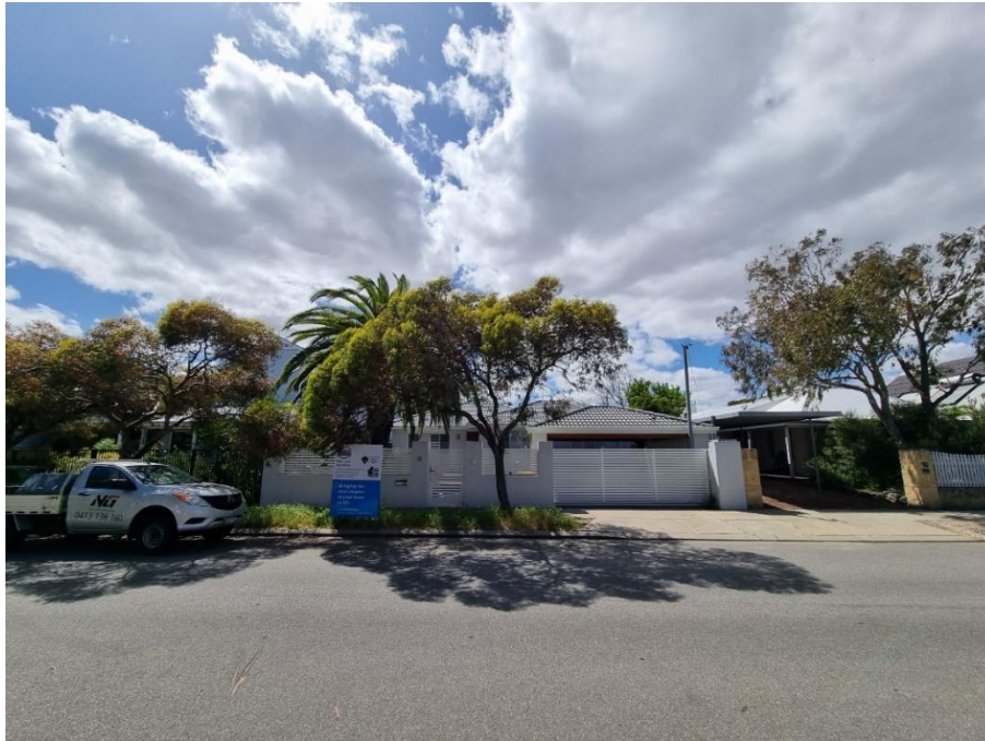
Photo 1: Subject site as viewed from Hickory Street
