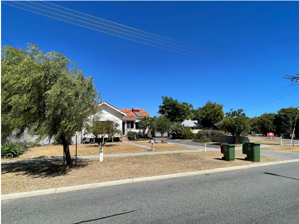
Photo 3: Subject site as viewed from Oldham Crescent (view southward)
