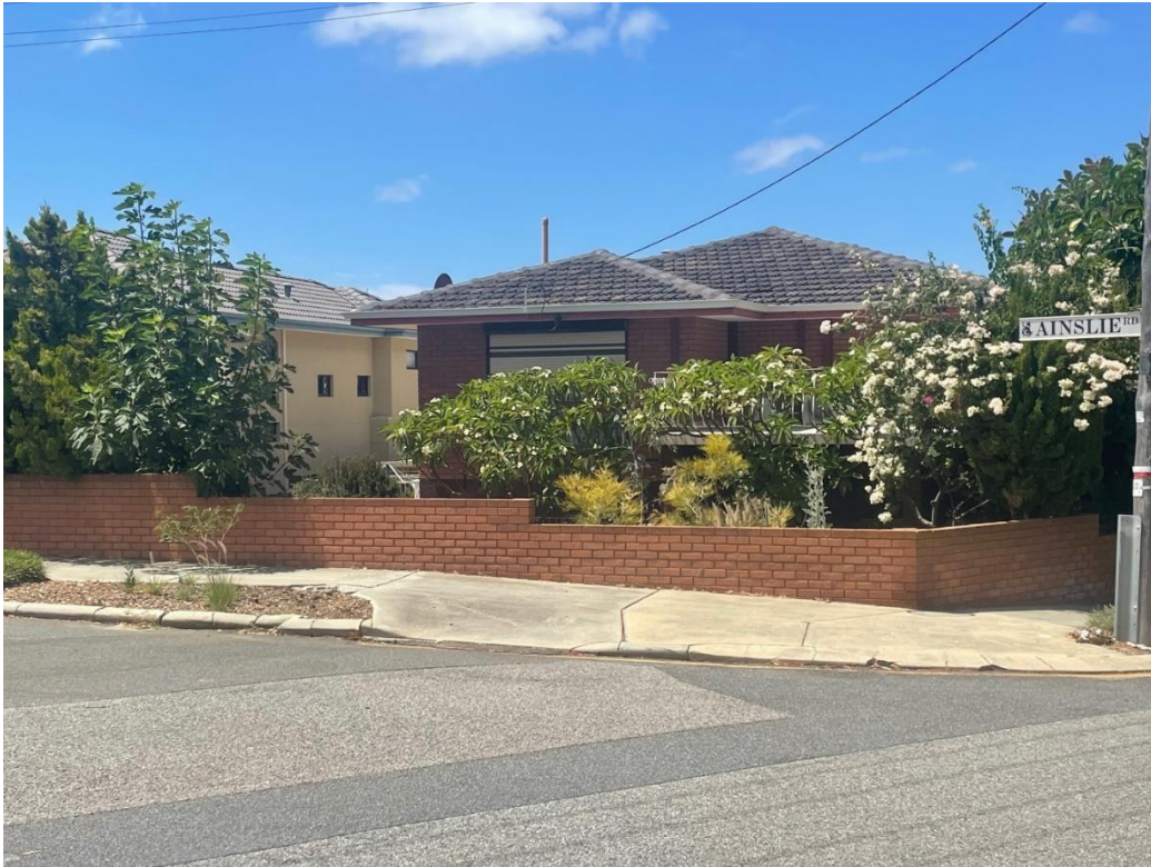
Photo 3: Adjoining property to the west (2 Rule Street) as viewed from Ainslie Road
