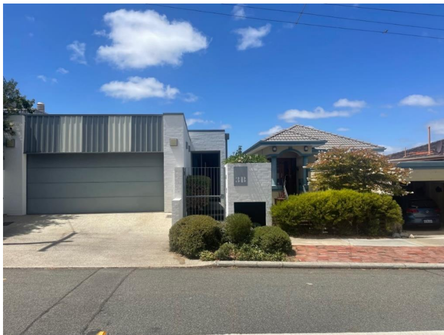
Photo 2: Adjoining property to the east (3B Ainslie Road) as viewed from Ainslie Road
