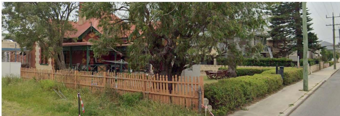
Figure 2 – Adjoining dwelling to the north east.
