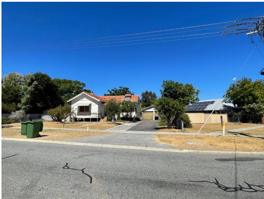
Photo 2: Subject site as viewed from Oldham Crescent (view eastward)
