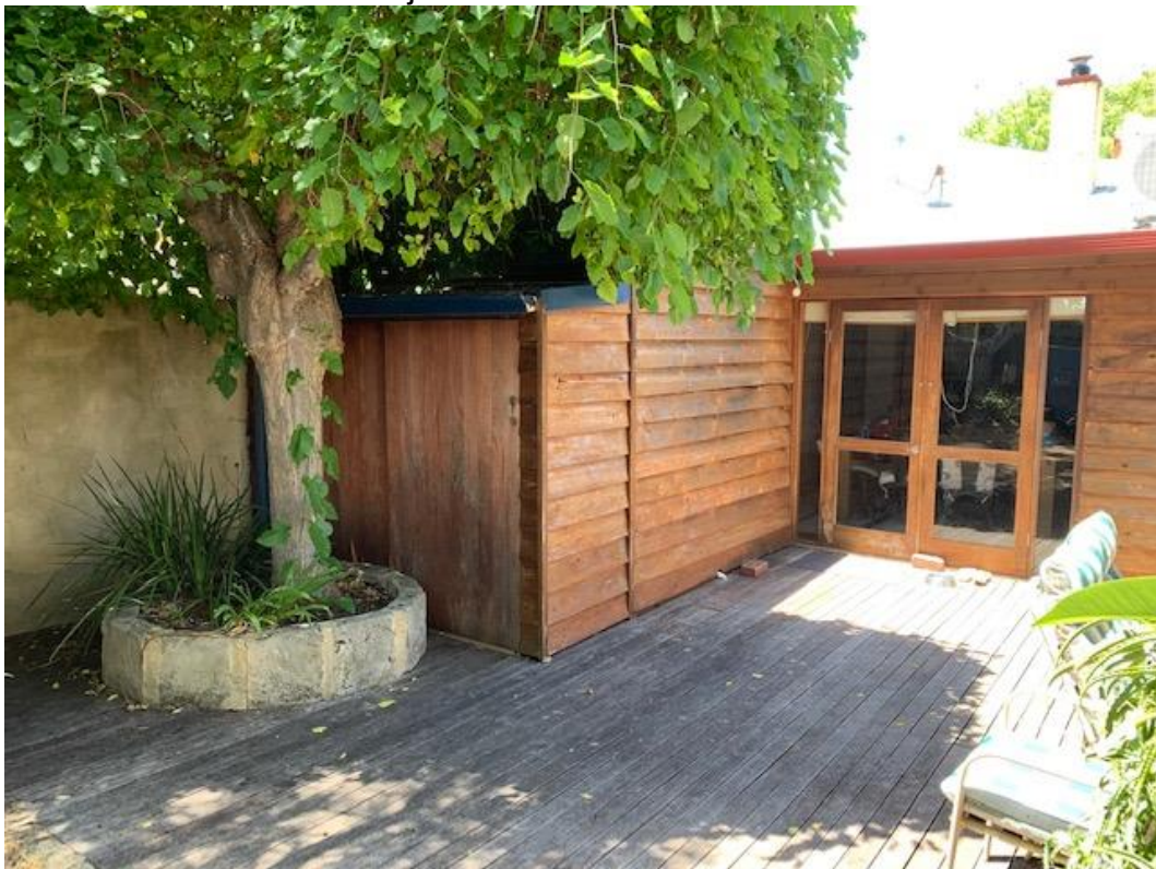
Photo 2: Existing rear elevation of subject site (to be demolished)
