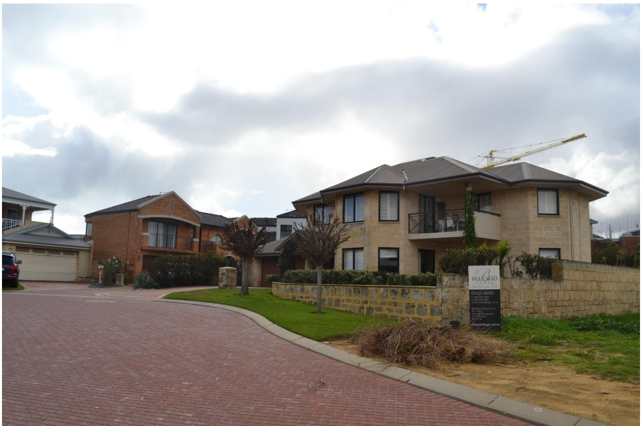
Photo 6: Existing streetscape of Keel Place
