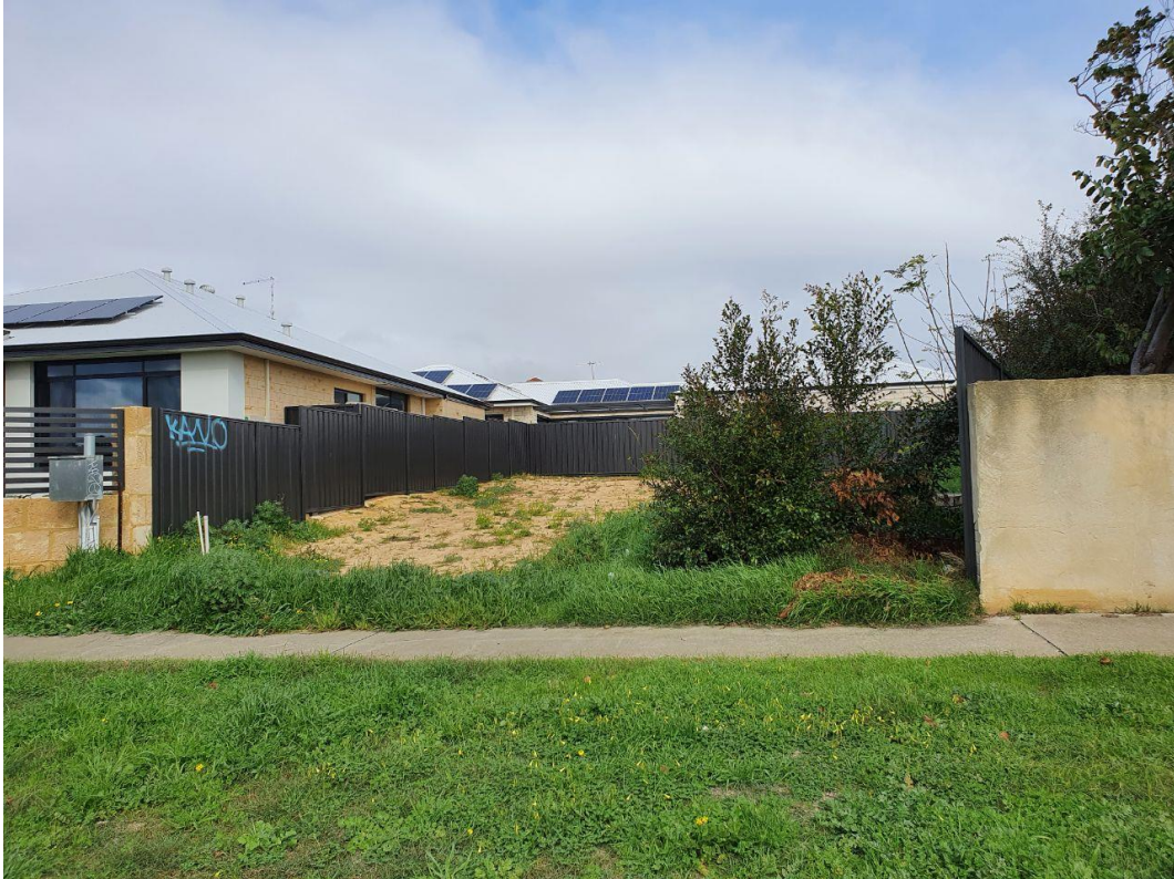
Photo1: Subject site as viewed from Watkins Street
