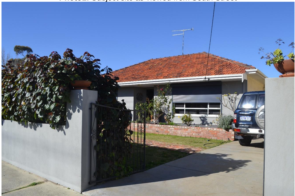
Photo 2: Subject site as viewed from South Street (behind front wall)
