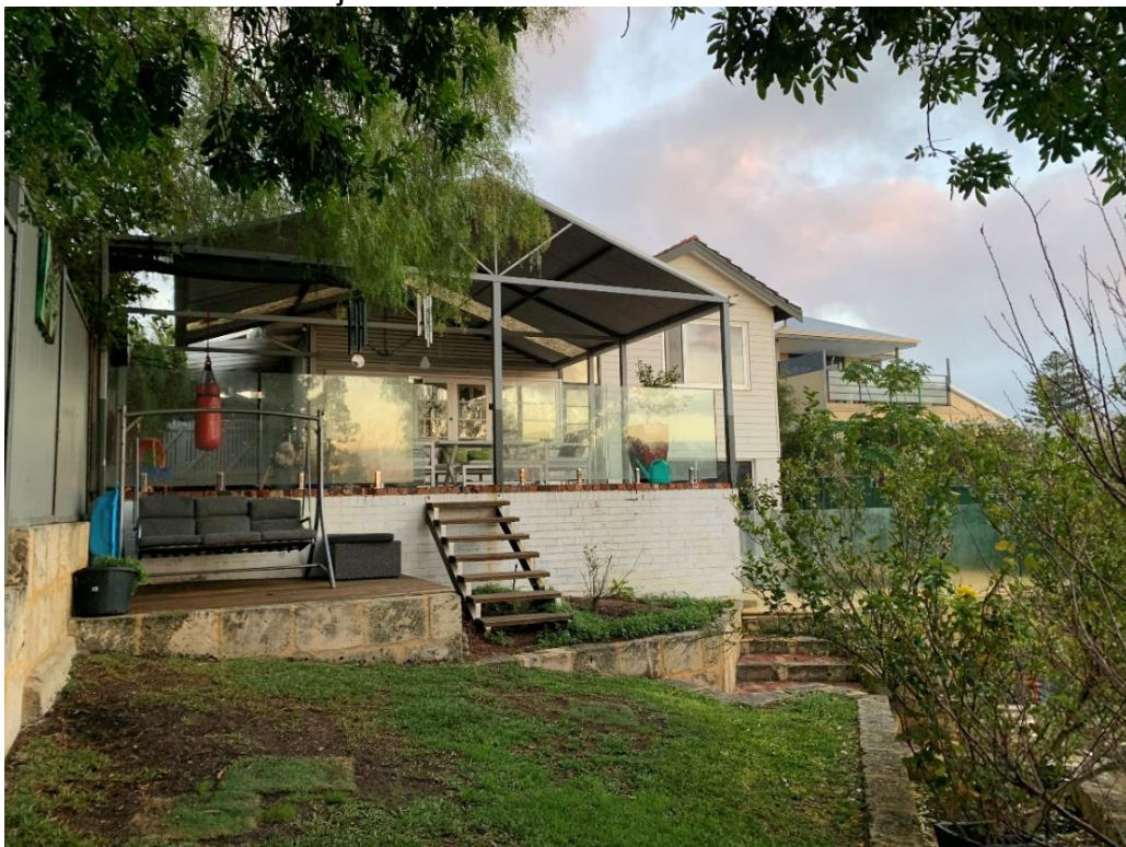
Photo 2: Rear of the subject site
