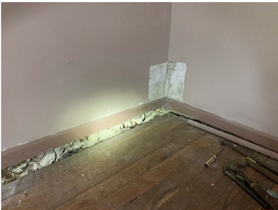
FIGURE 13 LIMESTONE CONSTRUCTION BELOW SKIRTINGS
