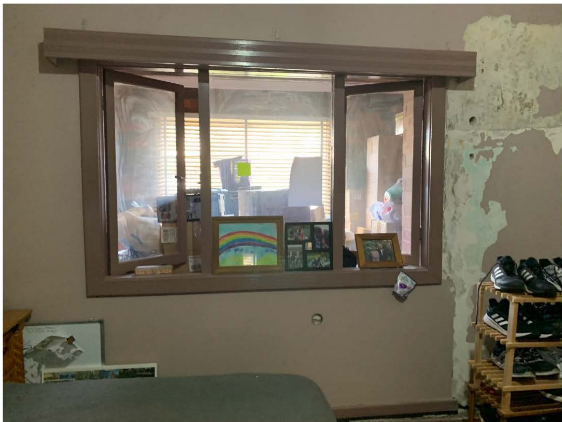
FIGURE 8 REPLACEMENT WINDOWS IN FRONT TWO ROOMS
