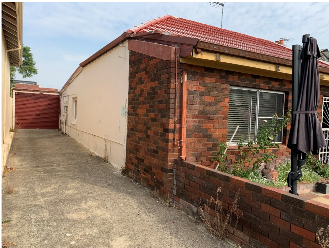
Photo 2: East elevation of existing house
