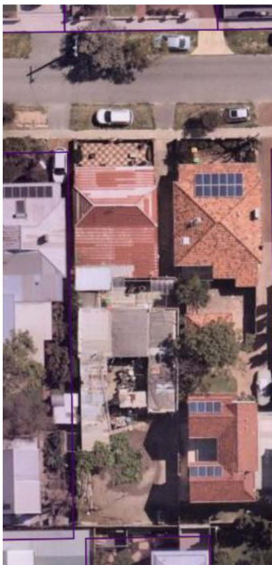
15 McLaren Street, Aerial photograph, ESRI, 27/11/2020
