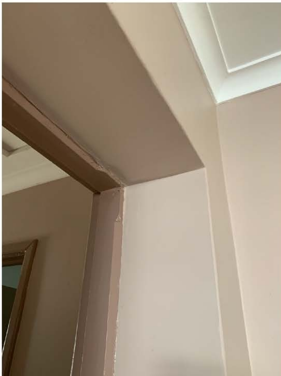
FIGURE 9 WIDTH OF ORIGINAL REAR WALL
