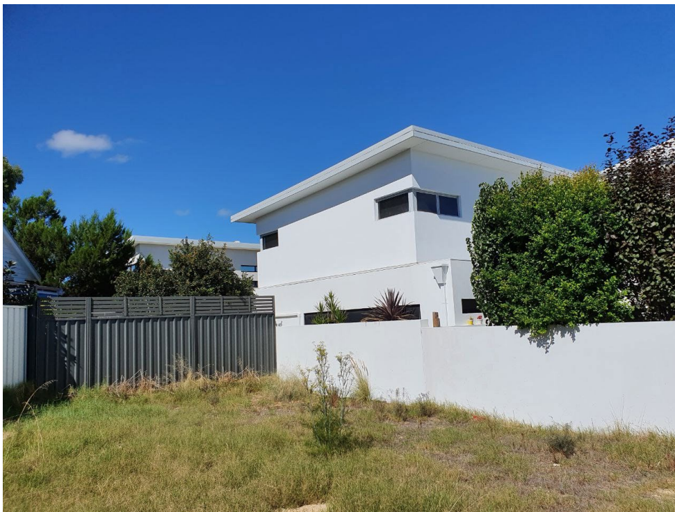
Photo 6: Rear elevation of lot 84
