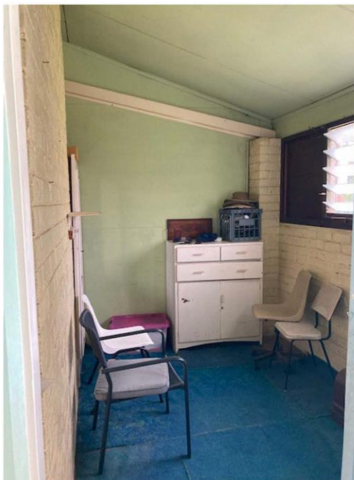
Photograph 14. Enclosed back verandah, north
