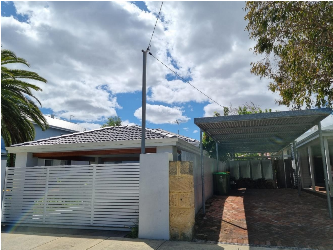
Photo 3: Subject site and carport area of adjoining southern property (No. 10)
