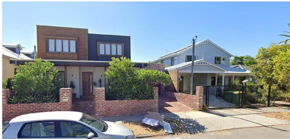
4 & 6 Hickory street (neighbouring two storey properties to the north)
