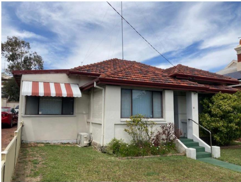
Photograph 2. Street façade, Hampton Road, showing detail of enclosed front porch.
