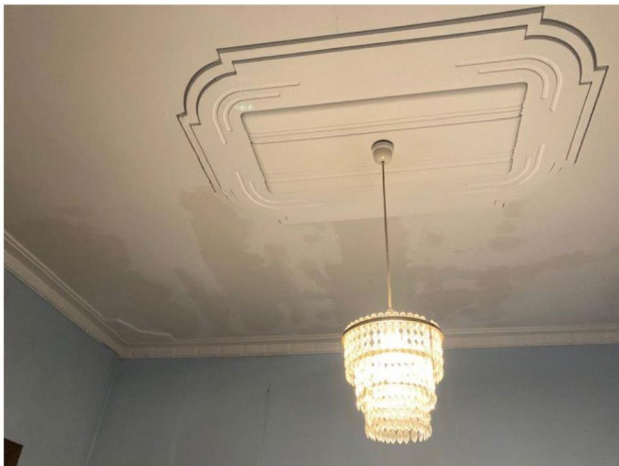
Photograph 8. Cast plaster ceilings, rose and cornices to Lounge.
