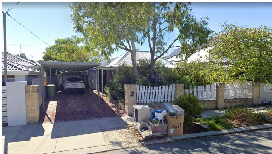
10 Hickory street (neighbouring property to the south)
