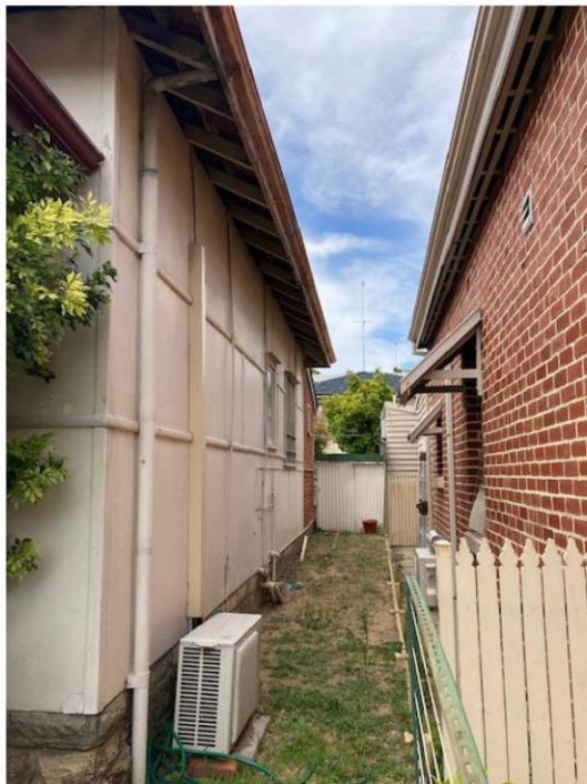
Photograph 6. South elevation of 32 Hampton Street.
