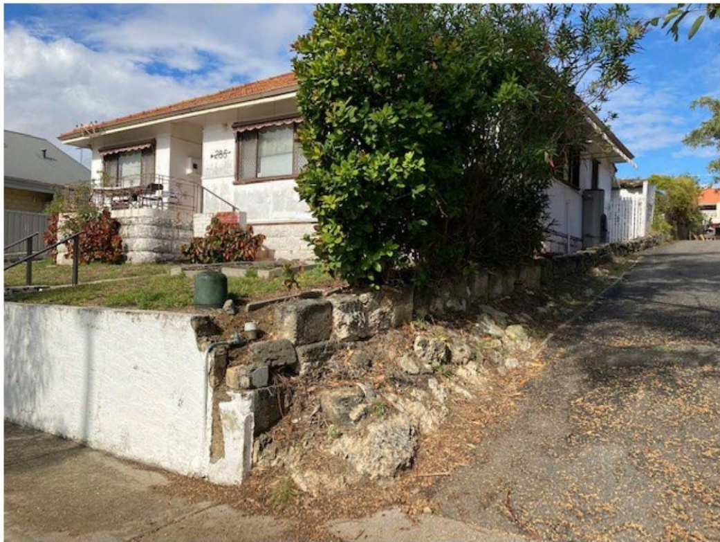
West side boundary wall
