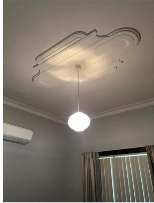
Photograph 10, Ceiling in front bedroom.
