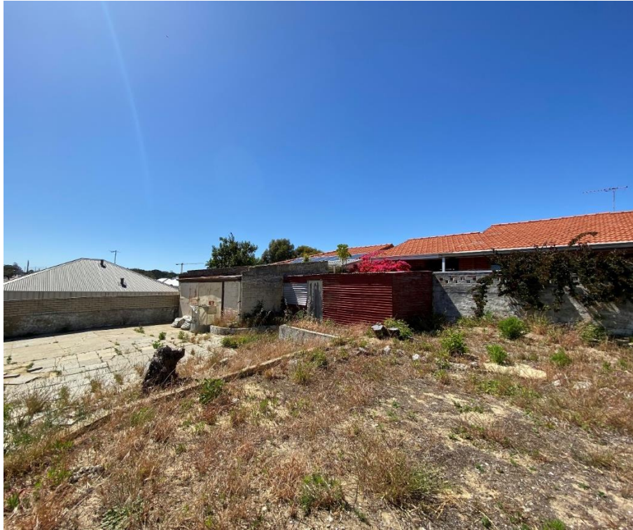
Photo 5: view of rear outbuildings and southern neighbouring properties
