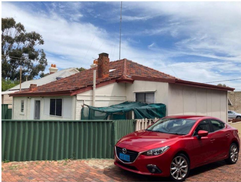
Photograph 3. North and east elevations and projecting timber framed sleepout.
