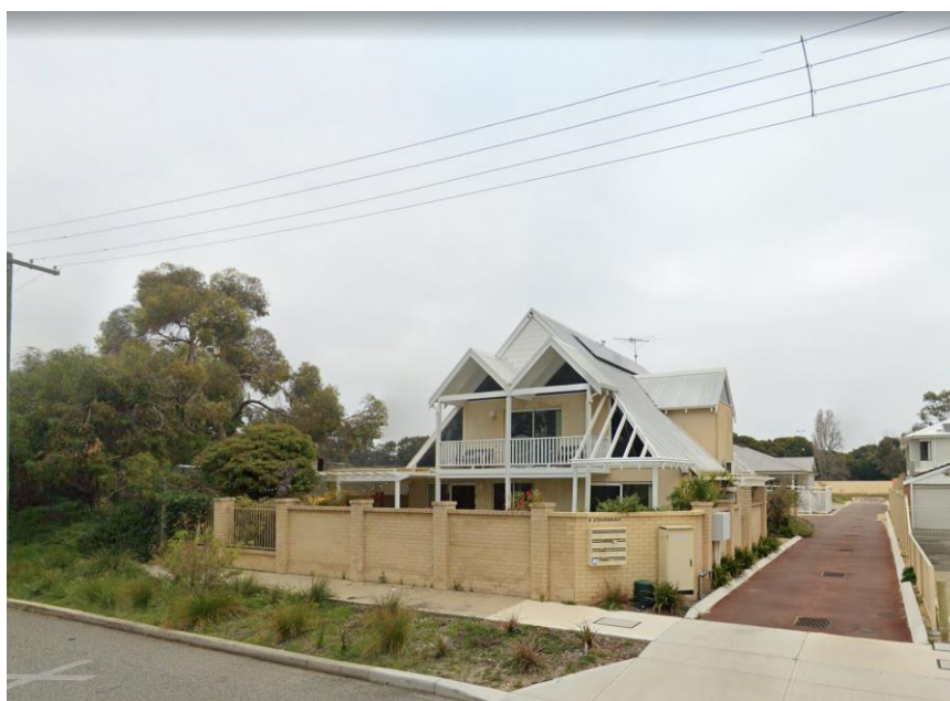
Photo 2: Southern adjoining property (4 Johannah Street)
