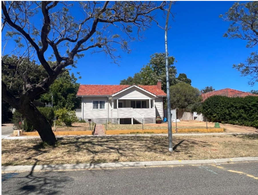
Photo 1: Subject site as viewed from Nicholas Crescent
