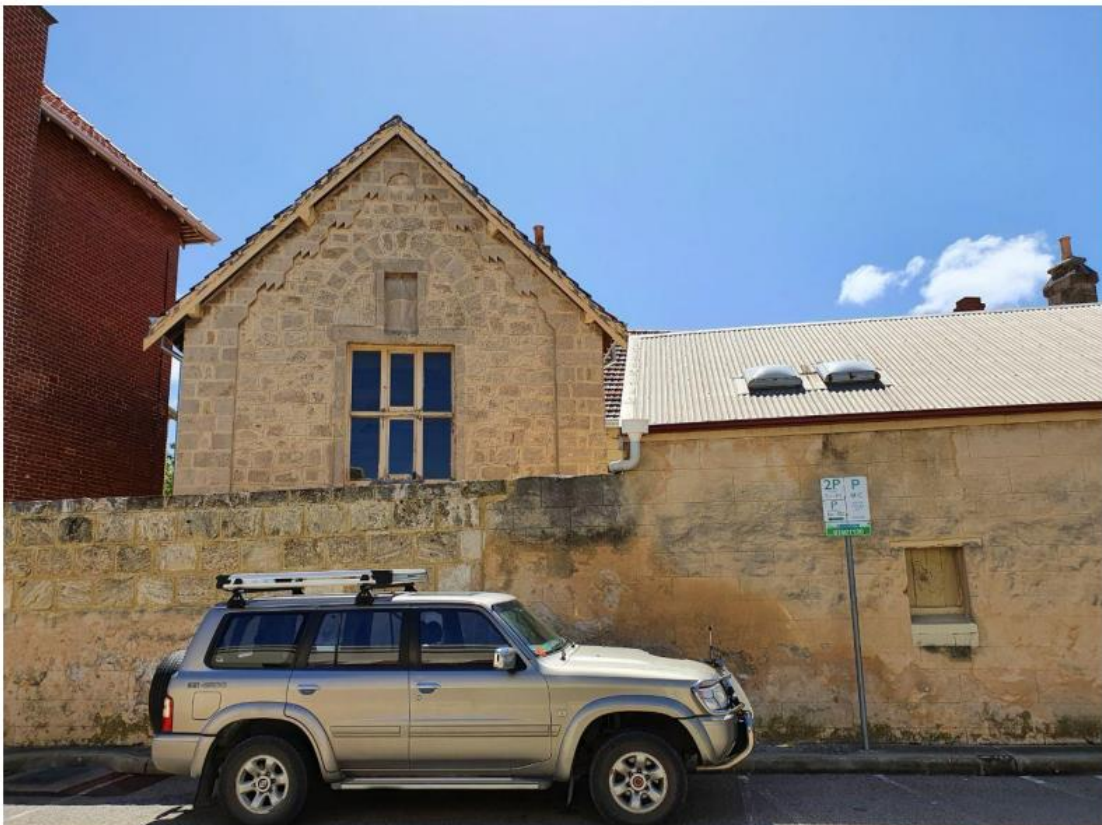
Photo 6 – Existing buildings from Norfolk Lane
