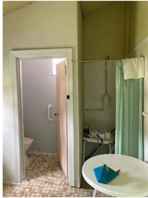
Photograph 13. Enclosed back verandah with toilet, shower and laundry.
