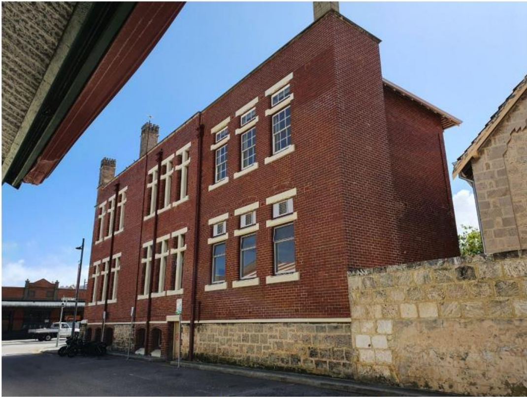
Photo 7 – Existing building not included in this application
