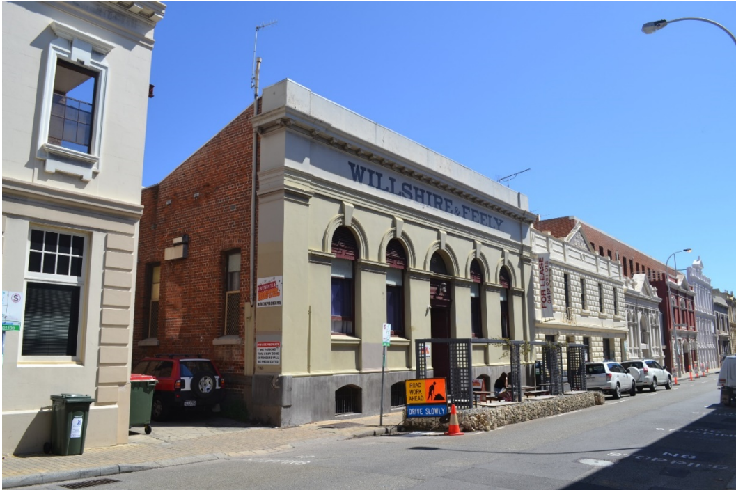
Photo 1: View of subject site.
