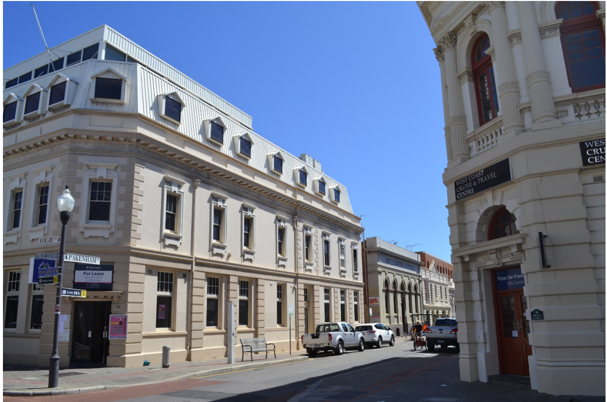
Photo 3: View of Pakenham St from High St (subject site in background).
