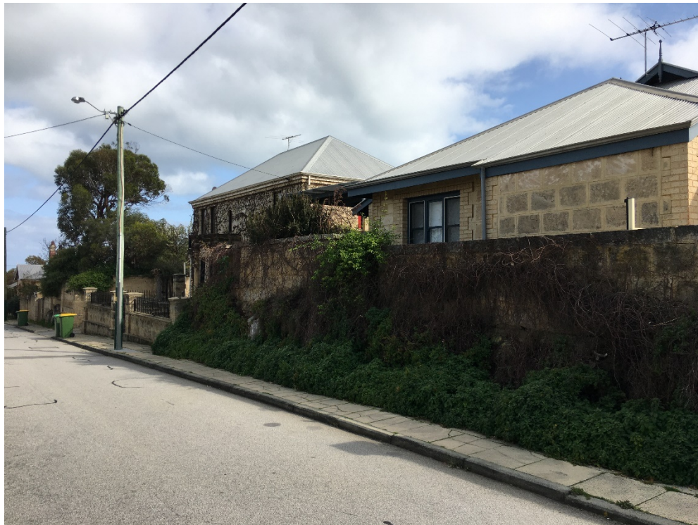
Photo 2: Martha Street elevation showing the rocky outcropping at the street boundary
