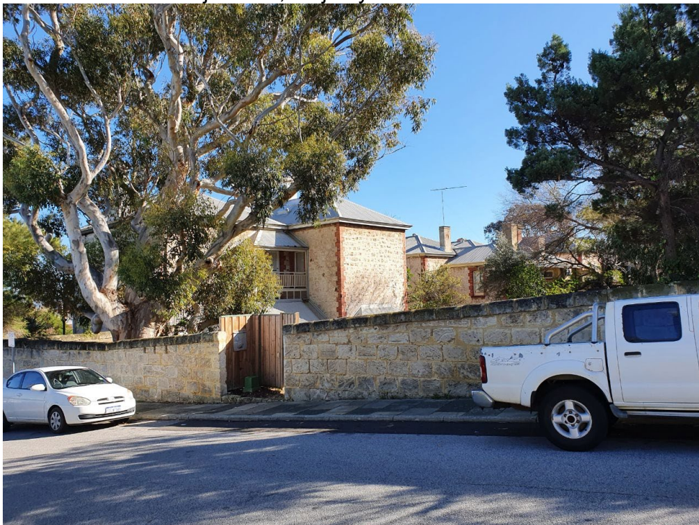
Photo 2: View across subject site towards 24 Ord Street
