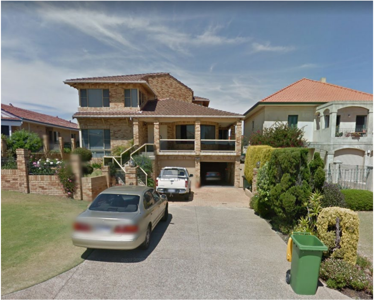
Photo 3- Neighbouring northern site
