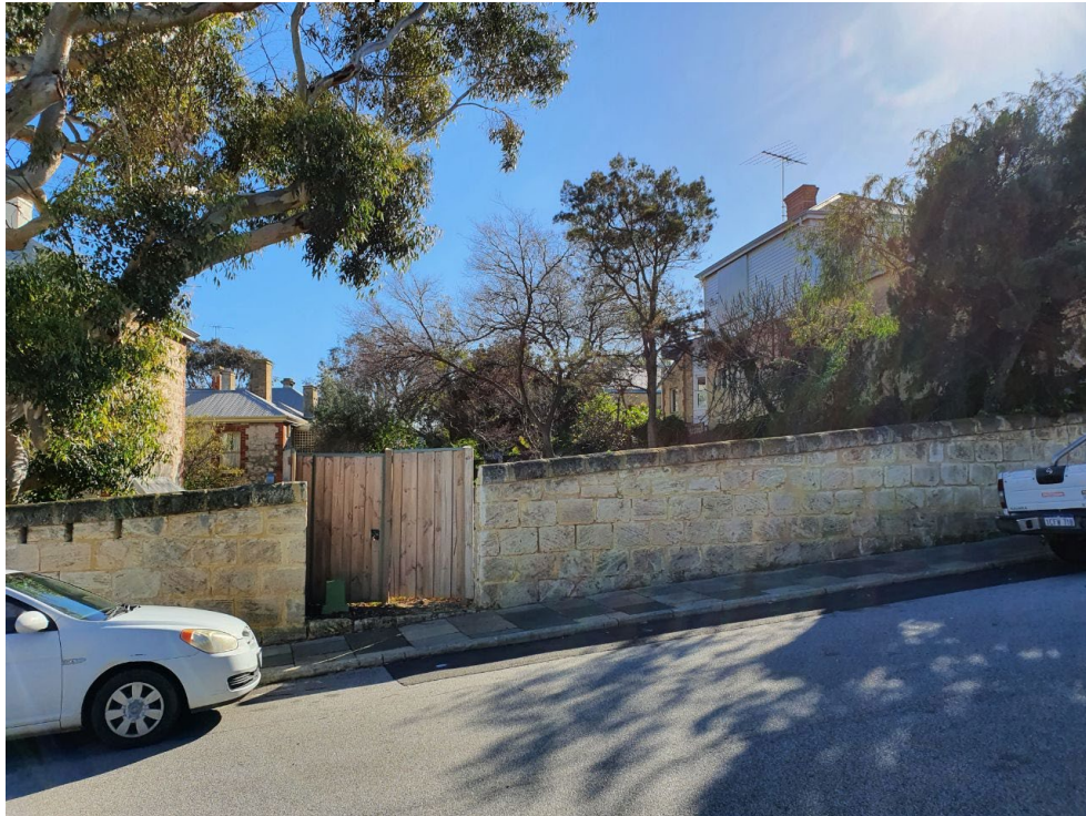
Photo 1: Subject site, majority of limestone wall to remain
