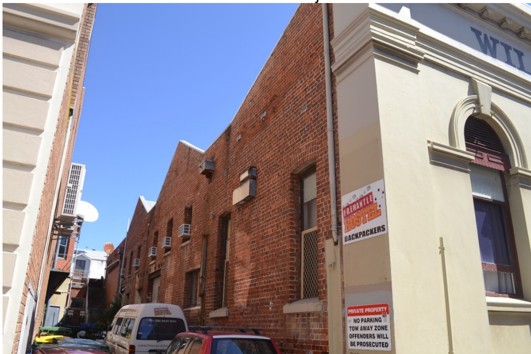
Photo 2: View along laneway (subject site in right of frame – proposal at rearmost portion of site).
