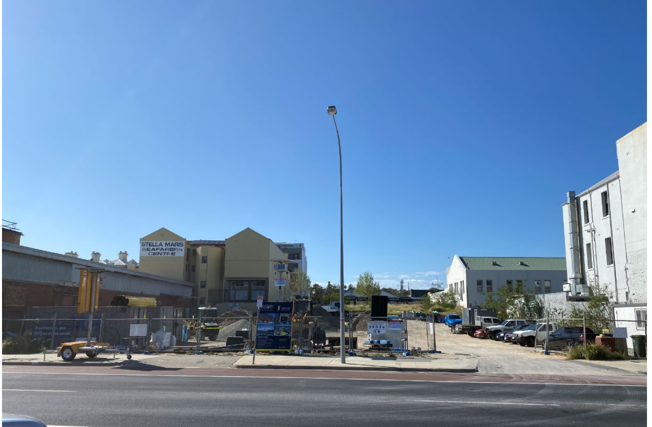
Photo 1: Subject site as viewed from Beach Street (currently being used as a laydown site for another project)
