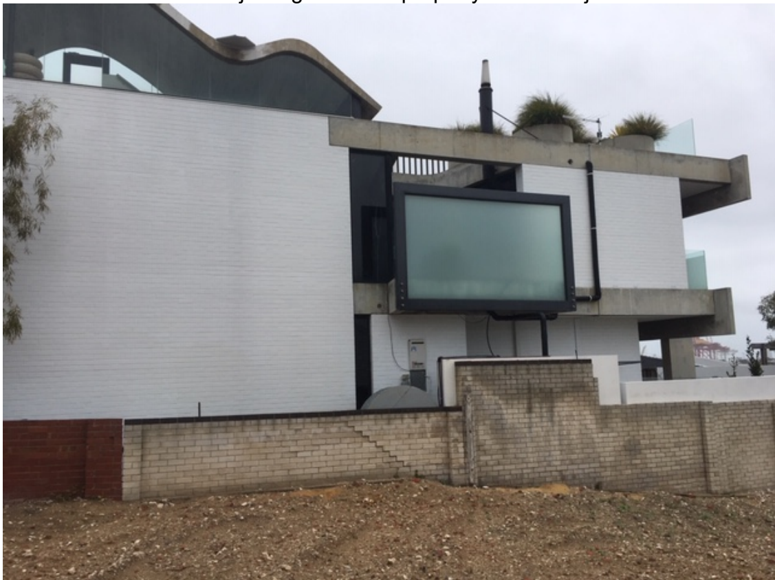
Photo 6: Southern adjoining dwellings northern wall
