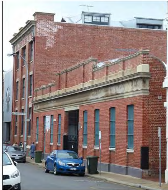
7.3.3 Modern detailing, with lesser depth (Note non-traditional red mortar)
