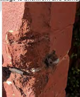
7.3.6 Example of damage to brickwork and damage to steel from acrylic paint
