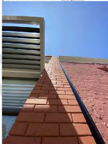
7.3.4 Example of curtain wall connection between buildings
