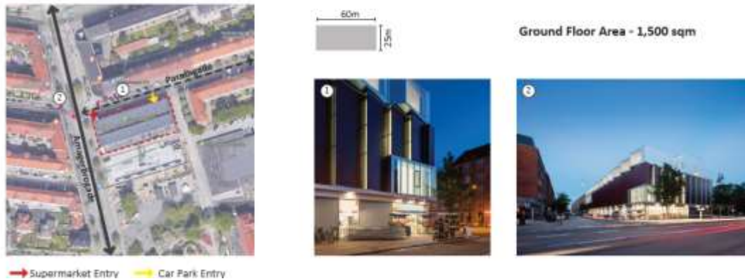
SH2-Sundbyøster Hall II / Denmark
