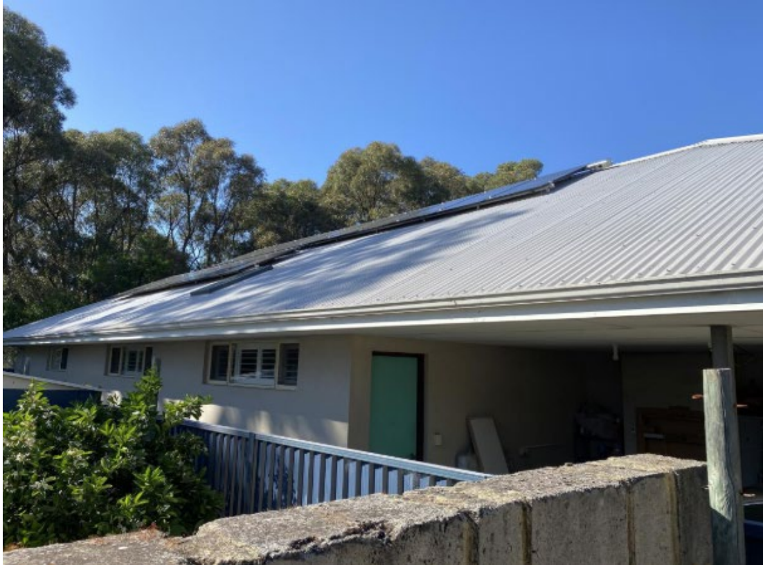
Image 1 - No.30 Bromley Road Sky light and Solar device
