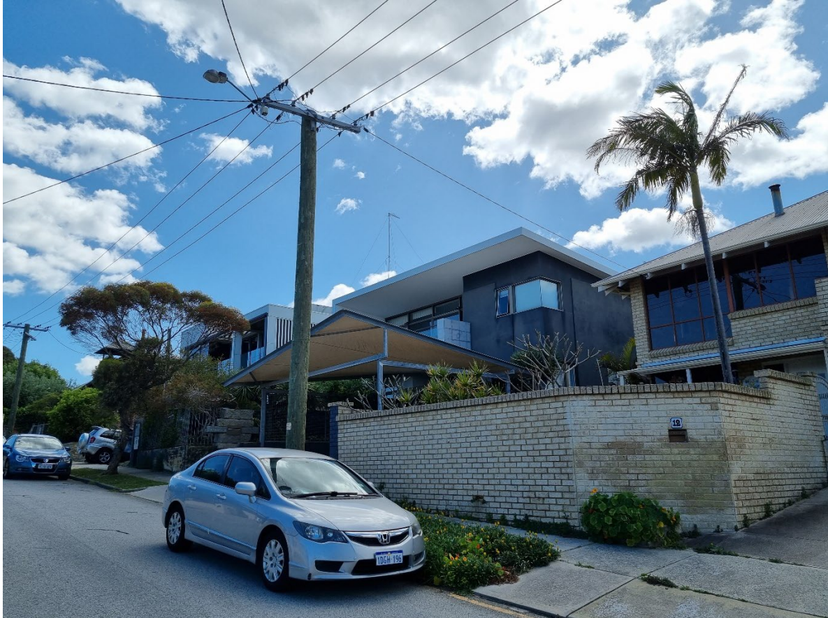
Images 2 & 3. Images of Existing Carport at Subject Site
