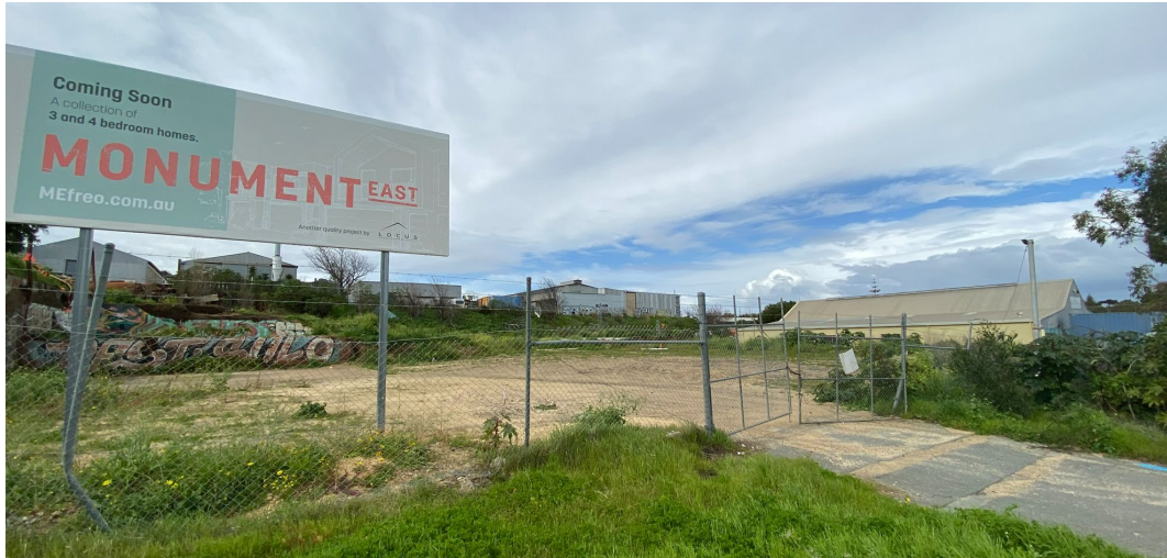
Figure 2: View towards existing retaining walls at subject site, highlighting the topography changes throughout the site.
