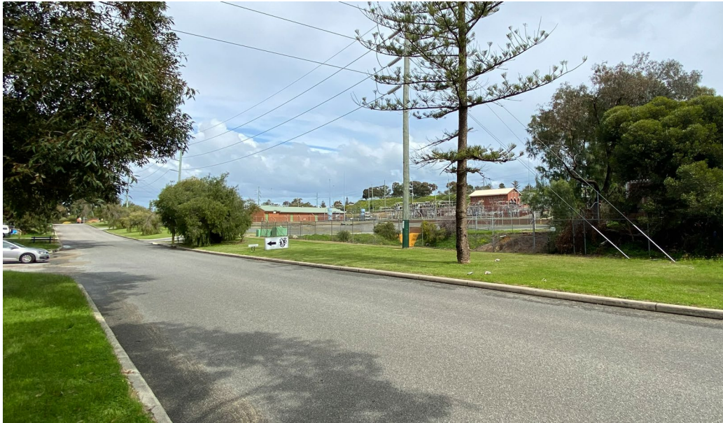
Figure 4: View towards the south-west towards Western Power Depot.
