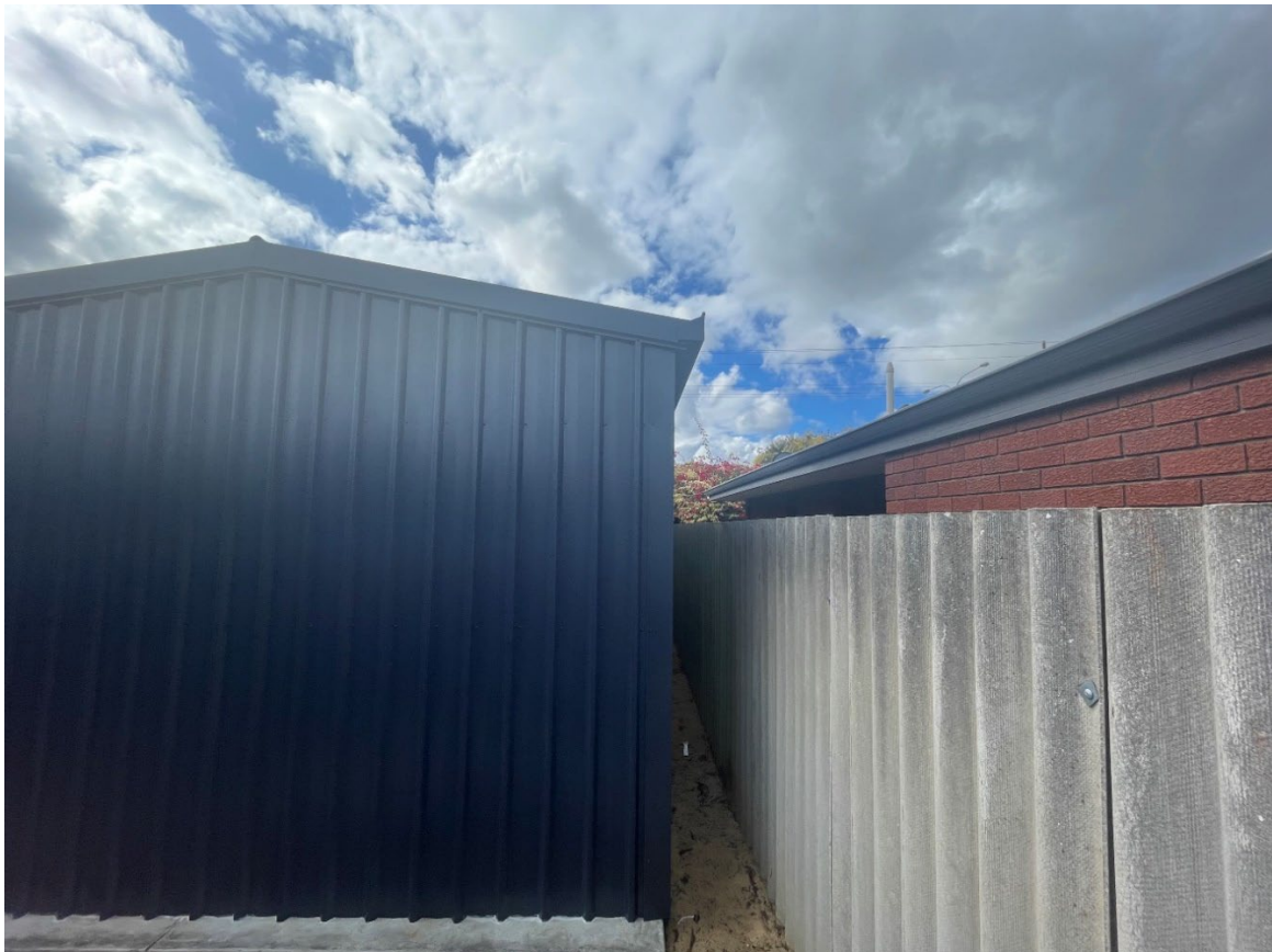
Figure 1 - Outbuilding Addition view North – showing height above existing boundary fence.
