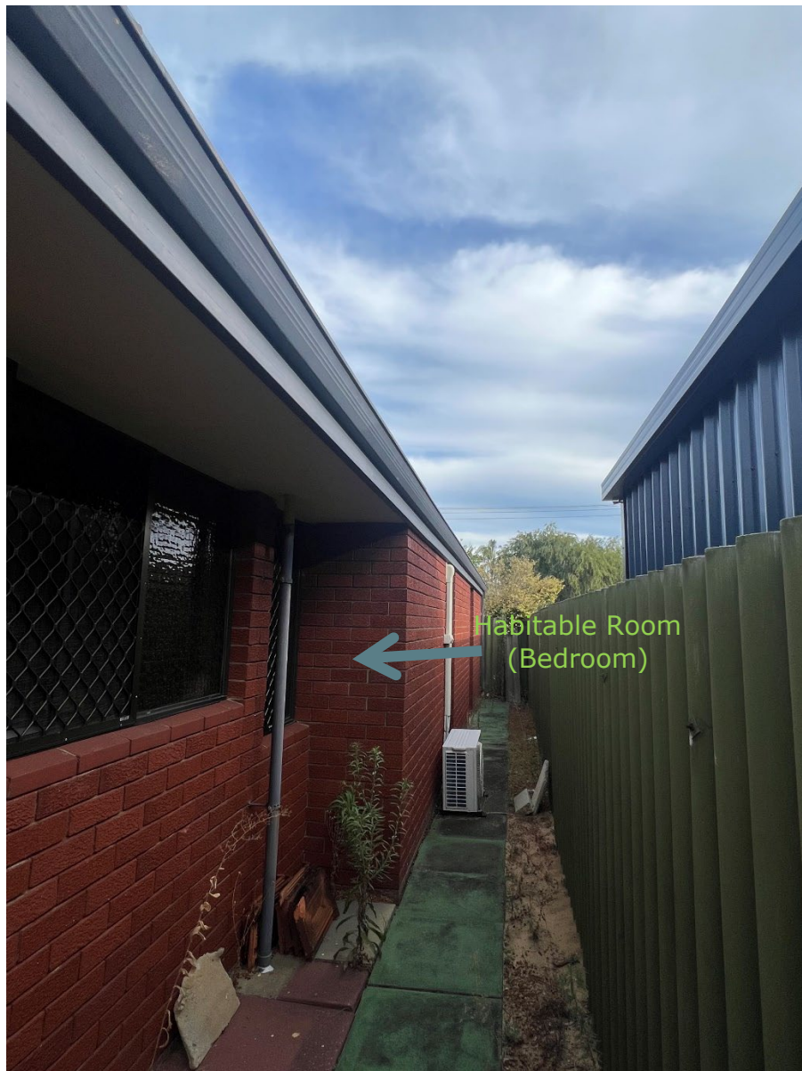
Figure 2 – View of Outbuilding addition from Eastern adjoining property – showing one habitable room (bedroom) adjacent to the outbuilding.
