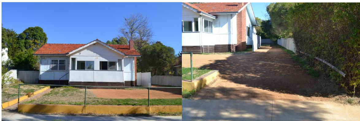
Figure 1 – Existing Crossover and Hardstand
