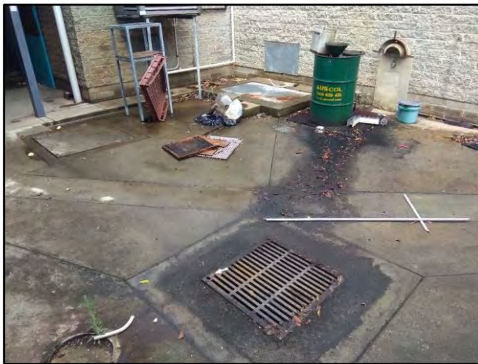
Plate 4: Fat and cooking oil storage drum, spilt fats and cooking oils on the ground surface toward a stormwater drain to the north of Building F.
