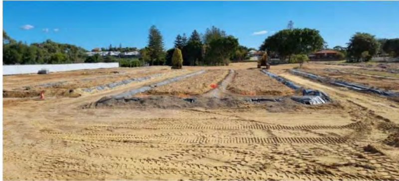
Photograph 1: Looking west across the site
