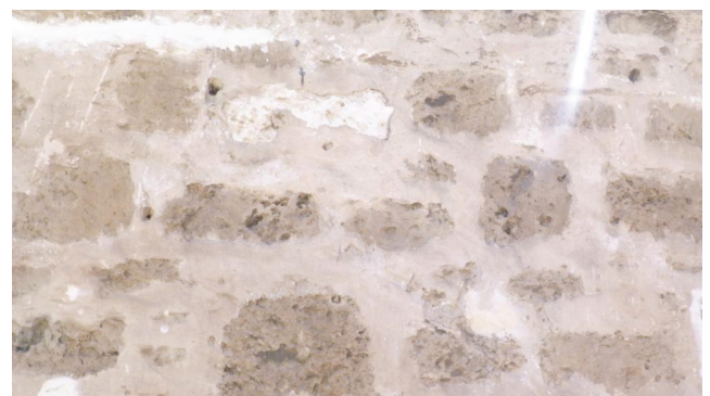
Flush-finished random rubble; mortar often covers most of the stones.
