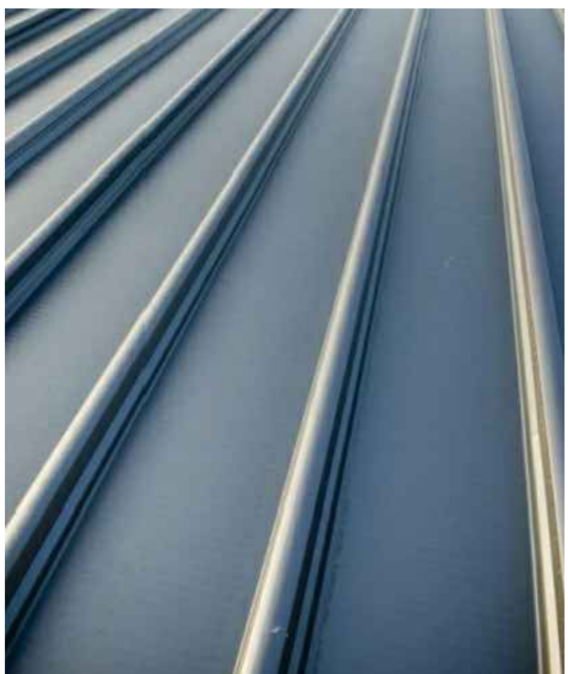
⑦ ROOF SHEETING LYSAGHT KLIPLOK - COLORBOND "WINDSPRAY"
