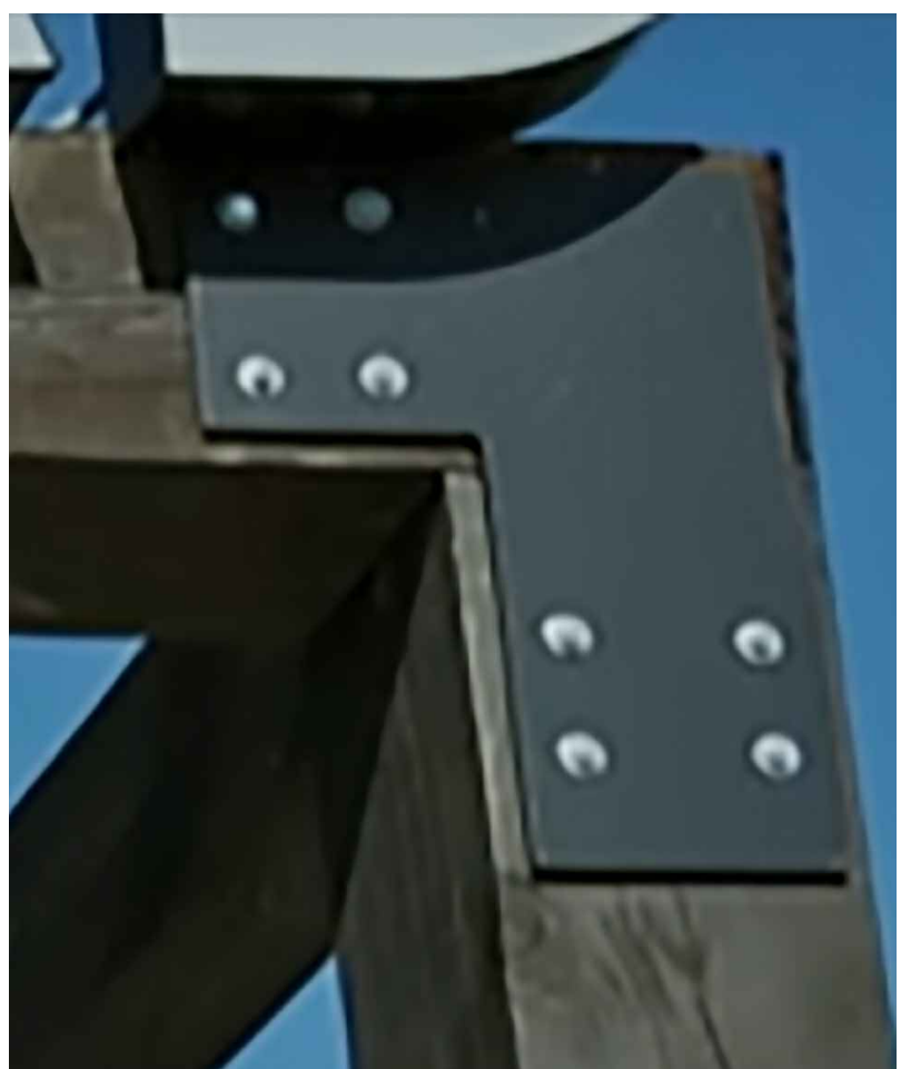
⑧ COLONADE EXPOSED STEEL BRACKETS BLACKENED STEEL
