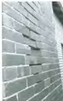
Masonry brickwork large gaps and loose bricks evident
