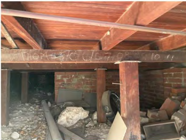
Sub-floor space showing timber floor structure and stumps
