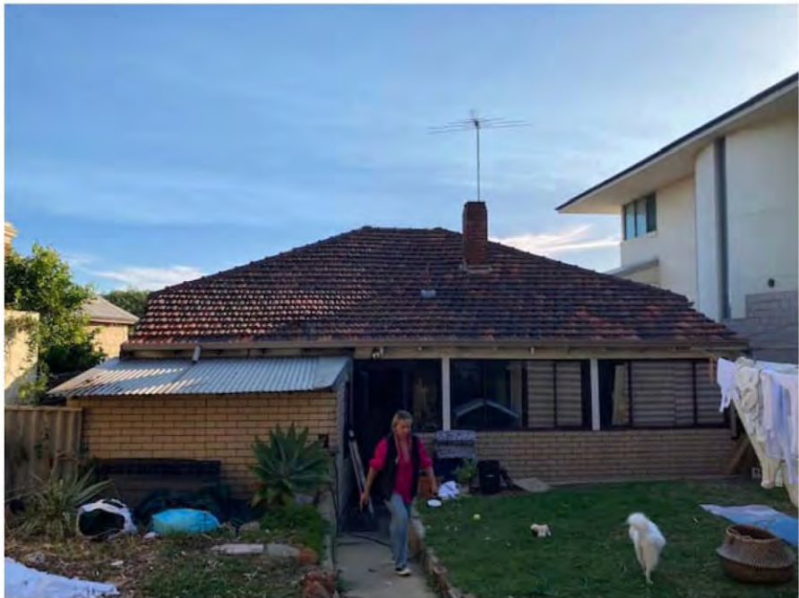
Rear (east wall) of house
