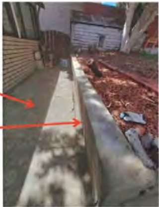
RETAINING WALL – BACK YARD
