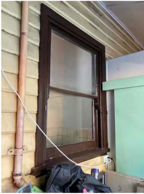
Kitchen window facing into rear verandah
