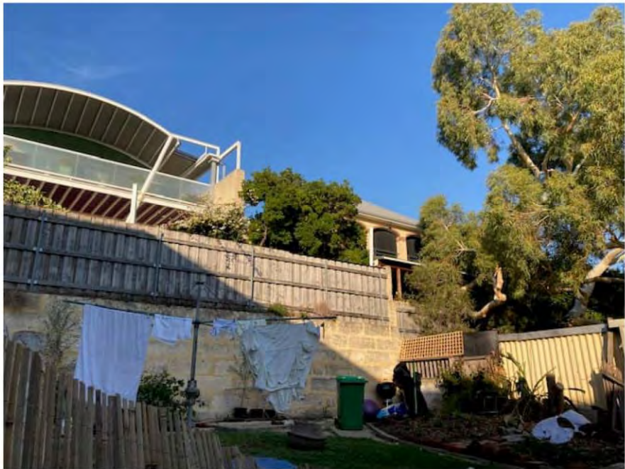
Back garden with high retaining wall
