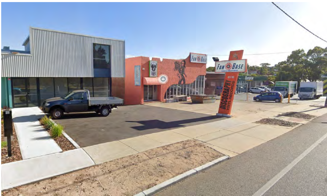
Photo 2: Subject site as viewed from South Street (western side)
