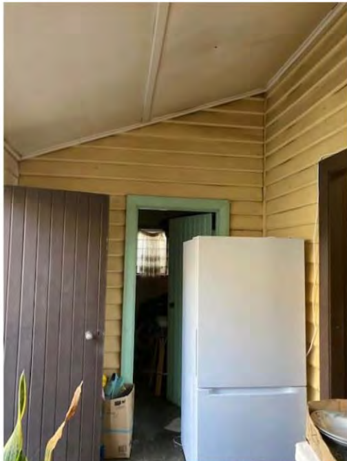
Enclosed rear verandah with original weatherboard external wall cladding
