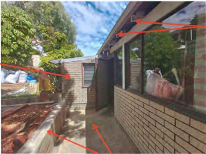
Cracked and miss-align retaining walls
