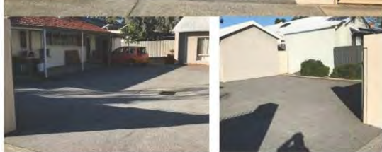
213 SOUTH AND CENTRAL AVE
