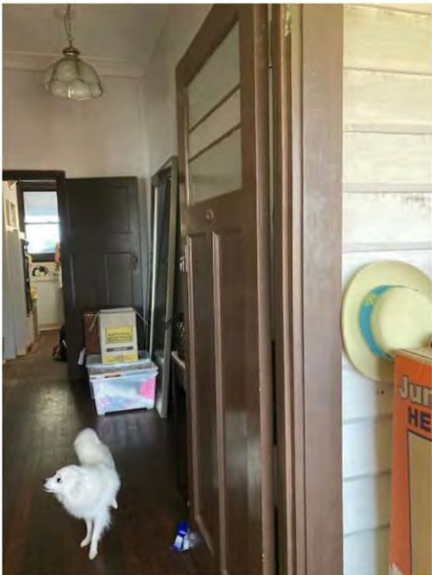
Front door and Hall
