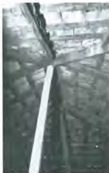
Chemical delignification present to timber roof battens and rafters. Advanced stage.
