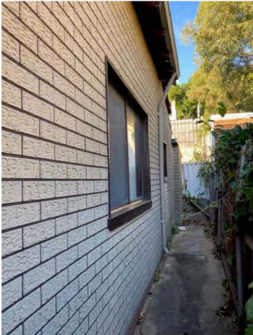
South wall of house
