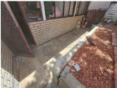
RETAINING WALL – BACK YARD
