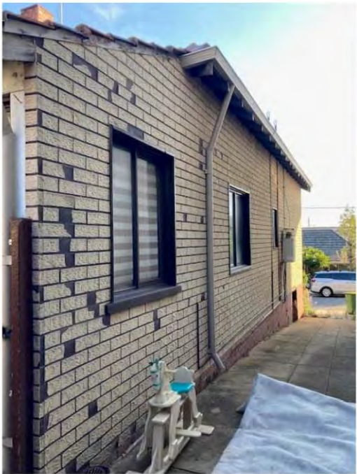
North wall of house
