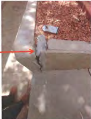
RETAINING WALL – BACK YARD
