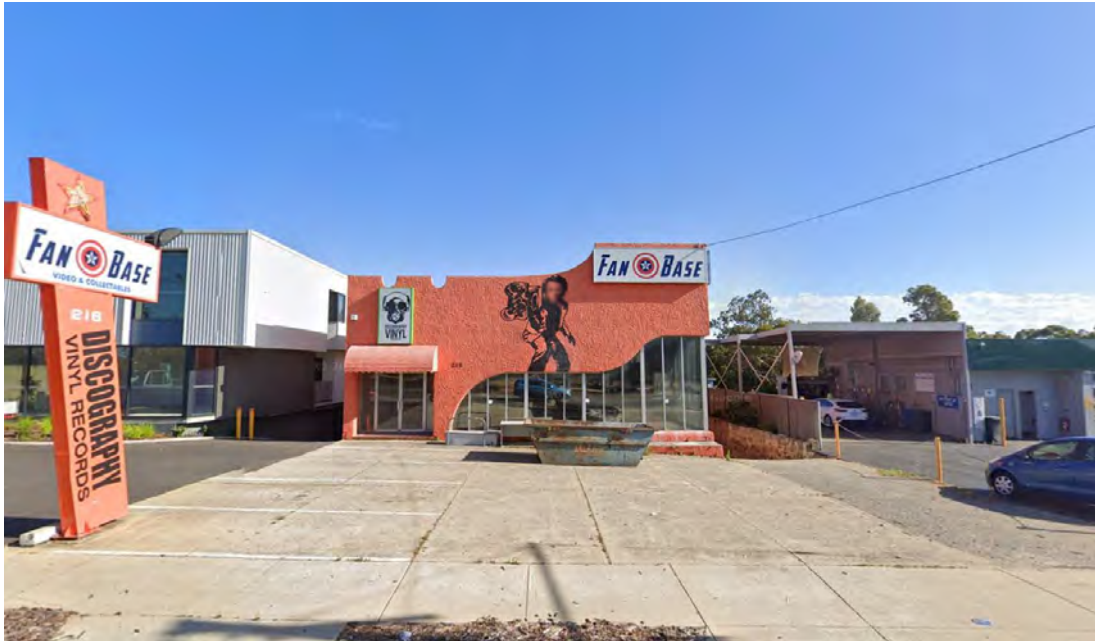
Photo 1: Subject site as viewed from South Street
