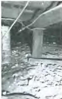
Loose timbers sitting in natural ground -sub floor
