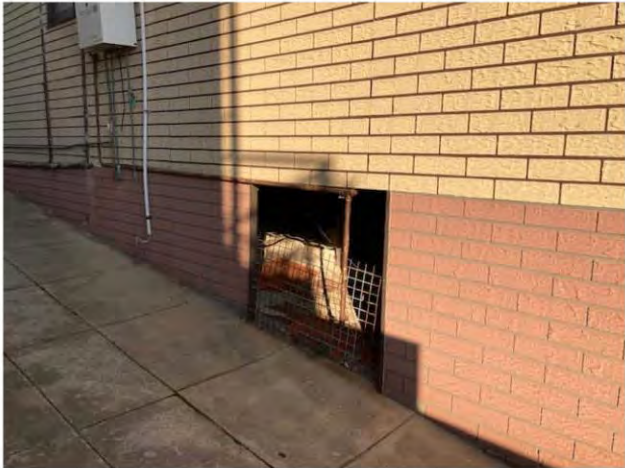
North wall, detail showing access to sub-floor space.
