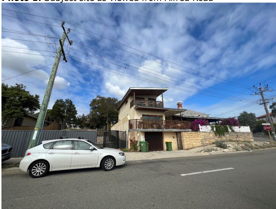
Photo 2: Subject site (behind fence) and adjoining property (18 Rule Street) as viewed from Alfred Road
