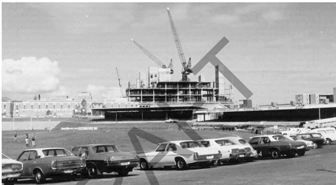
Photograph 012: A photograph showing Fremantle Oval as it was in 1978. The 1970 introduction of an internal carpark is shown in full effect. Construction is visible in the background of the image taking place at the Fremantle Hospital. Image courtesy Fremantle City Library, Ref no. 0984D.
