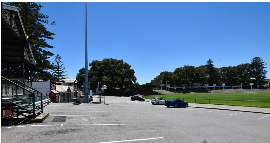
Photograph 26 The oval looking north with the bitumen paved area Victoria Pavilion, William Street gates, terraces and tree screen. Griffiths Architects December 2021. The original shallow gradient to the pavilion was later increased to its present form.
