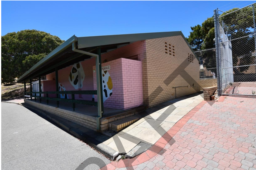
Photograph 41 One of two toilet blocks. Griffiths Architects December 2021.
