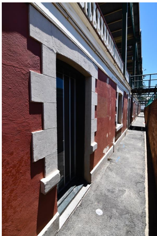
Photograph 36 Victoria Pavilion eastern ground floor wall. Griffiths Architects December 2021 . The wall to the right and gangways are later additions. The original bank was only 900 high.
