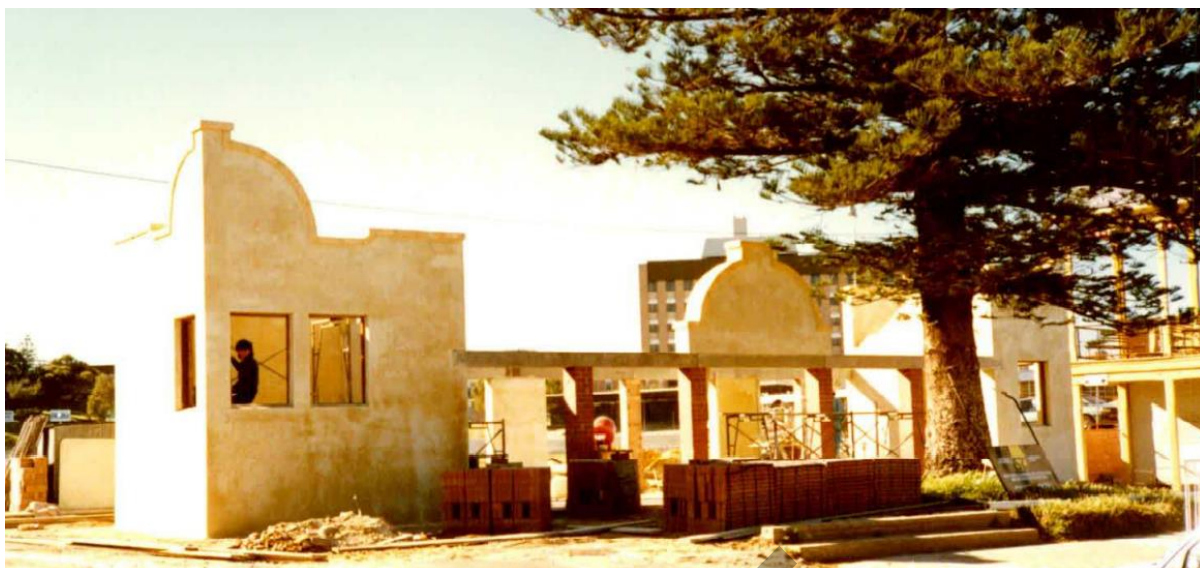
Photograph 17: A photograph showing the new turnstiles and gatehouse under construction c. 1986.
