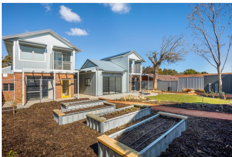
Figure 10. Units 3 and 4 viewed from the communal garden (Credit: The Green Swing and Shaina Bostin Photography)
