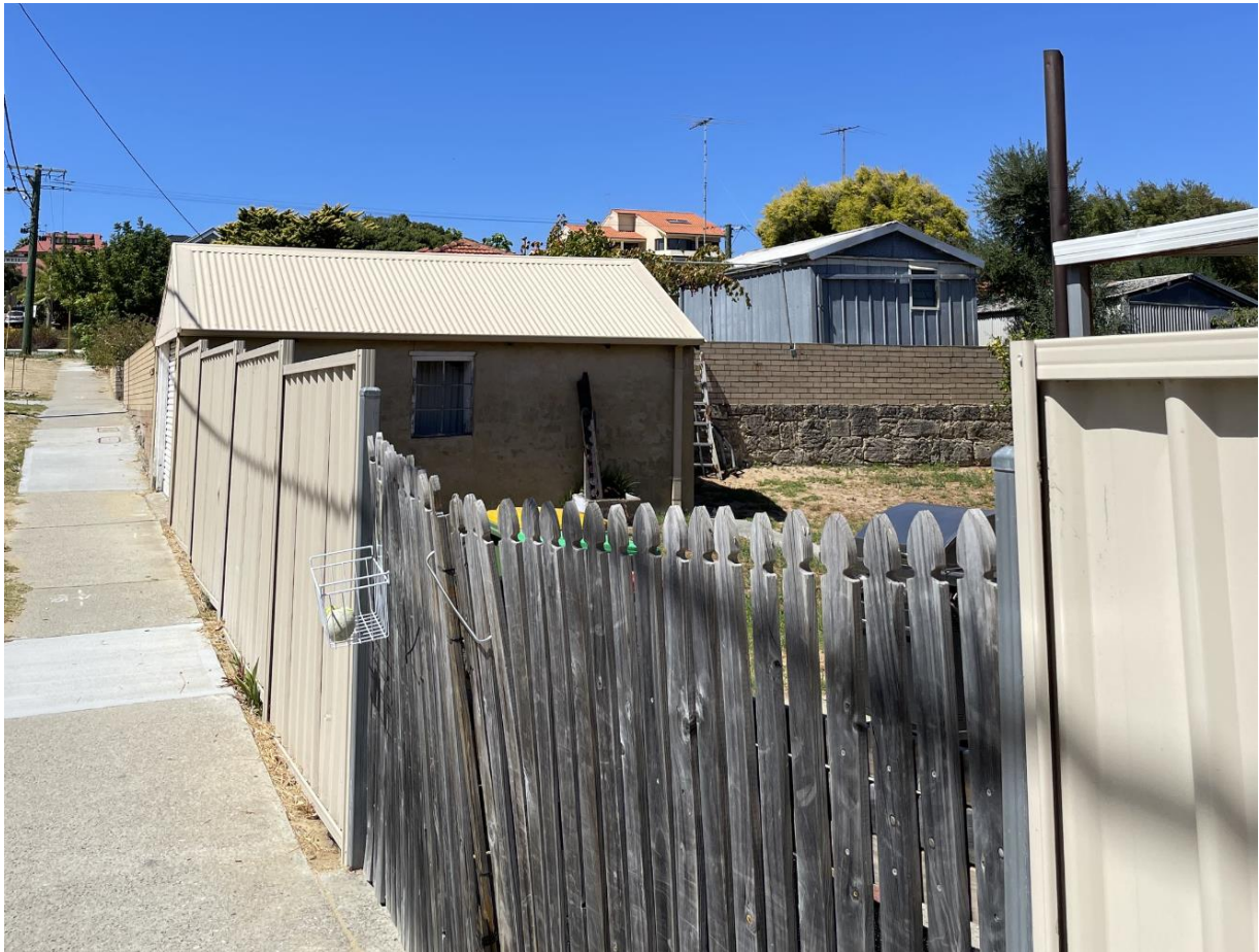
Photo 3: Subject site as viewed from adjoining lot on Scott Street looking east.
