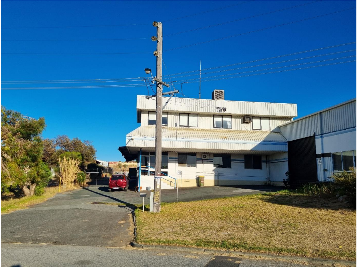
Photo 2: Subject site as viewed from Mather Road
