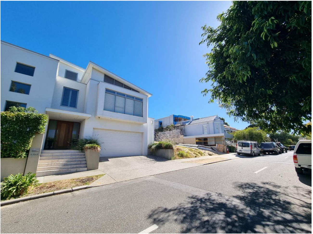
Photo 3: Subject site as viewed from Ainslie Road (west of subject site)
