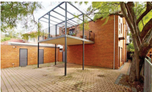
View from Site Car Parking
