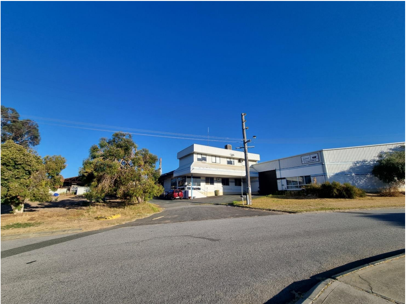
Photo 1: Subject site as viewed from Mather Road
