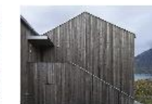
VERTICAL TIMBER CLADDING
