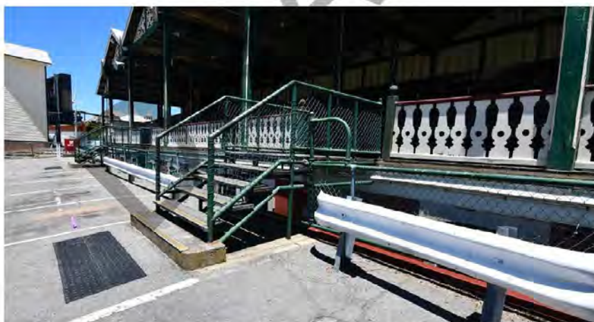
Photograph 29 Raised levels in front of the Victoria Pavilion. Griffiths Architects December 2021 The east face of the pavilion has been obscured by this intervention from the 1950s the balustrade is a reconstruction.
