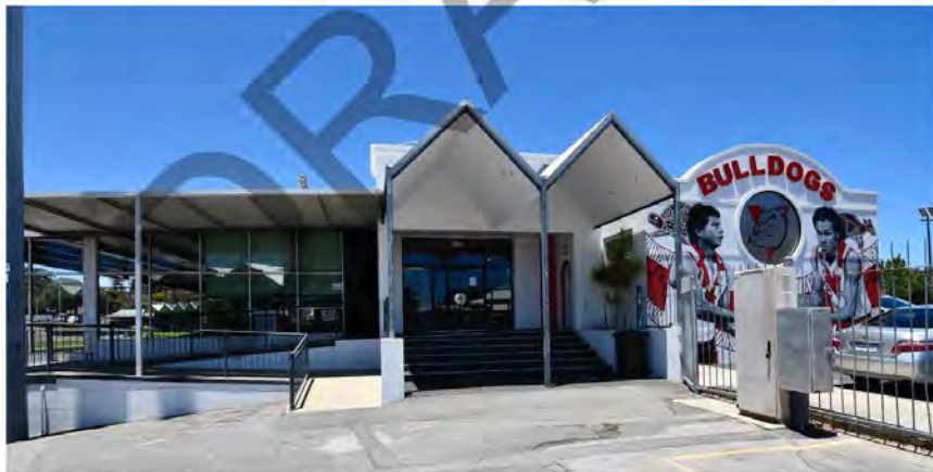
Photograph 38 Griff John Pavilion from the west. Griffiths Architects December 2021.
