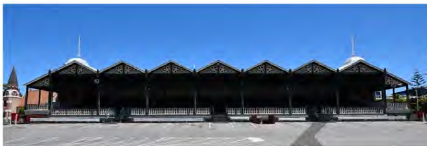
Photograph 33 Victoria Pavilion east elevation. Griffiths Architects December 2021 . The embankment and paving detract from the presentation of the place.
