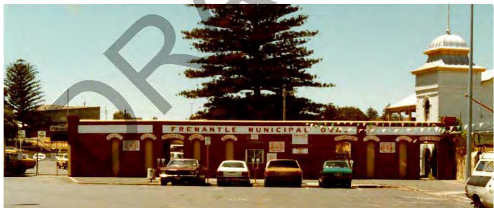
Photograph 14: A photograph showing the original turnstile gates from William Street c. 1984. The Victoria Pavilion is painted at this stage.
