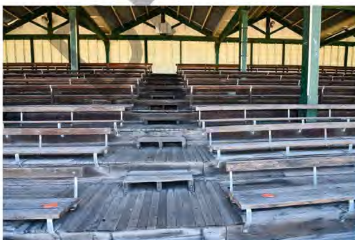
Photograph 34 Victoria Pavilion bleachers and seats. Griffiths Architects December 2021 . There is a mixture of new and replacement material.
