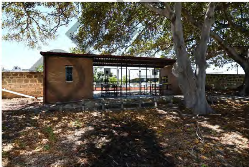
Photograph 40 Fothergill Street entry gates from the west. Griffiths Architects December 2021.
