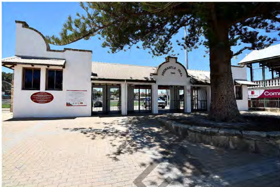
Photograph 43 William Street gates. Griffiths Architects December 2021.
