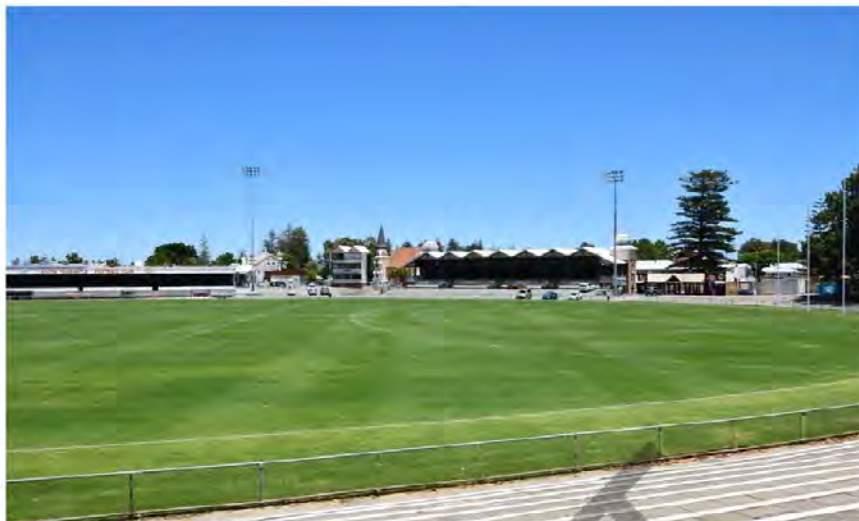
Photograph 28 The eastern oval from the eastern terraces. Griffiths Architects December 2021 Bulldogs Clubrooms, Broadcast Box, Victoria Pavilion and William Street gates.
