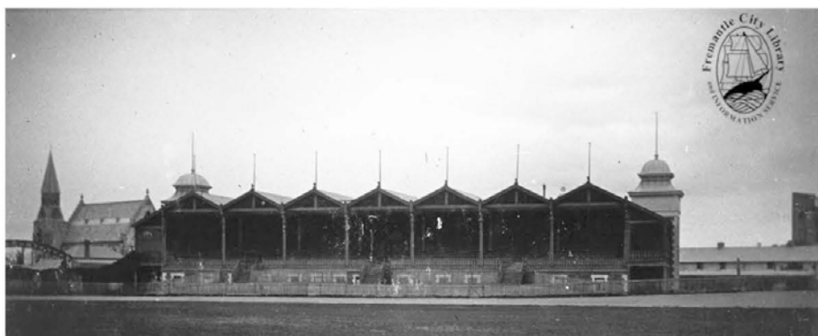
Photograph 06: Victoria Pavilion c. 1920s. Image courtesy Fremantle City Library, Ref no. 1865. Arched entry to the ground and Scots Presbyterian Church to the left and Warders Cottages to the right.
