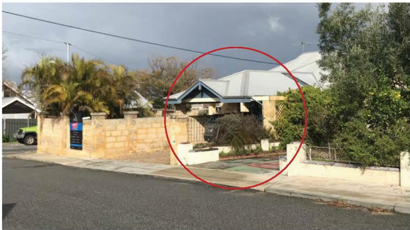
08. 21 TRAFFORD ST (SUBJECT SITE) - EXISTING CARPORT WITH LATTICE SCREEN TO NORTH BOUNDARY (CIRCLED IN RED) IN LOCATION OF PROPOSED TIMBER SCREEN. EXISTING HIGH LIMESTONE FENCE OBSCURING VIEWS TO MARTHA ST
