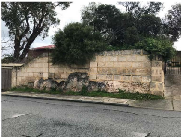
07. 148 MARTHA ST - HIGH LIMESTONE BOUNDARY FENCE WITH EXPOSED REMNANT LIMESTONE CAP ROCK
