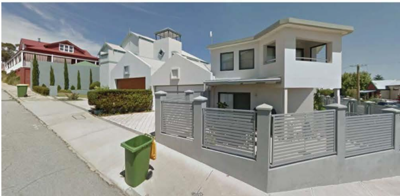
05. 28 & 30 MARTHA ST - CONTEMPORARY BUILDINGS IN STREET WITH REDUCED STREET SETBACK TO PRIMARY STREET
