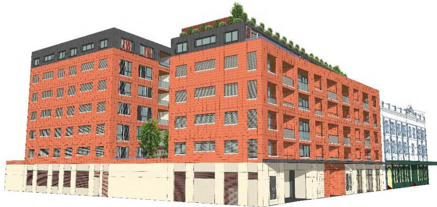
VIEW LOOKING FROM NORTH
