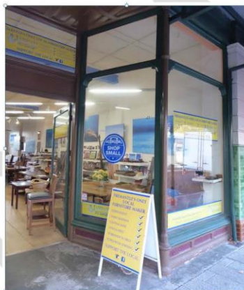
Gold rush era timber shopfront. Note steel structural column to corner, panelled soffit, dado tiling to piers and cast iron vents.
