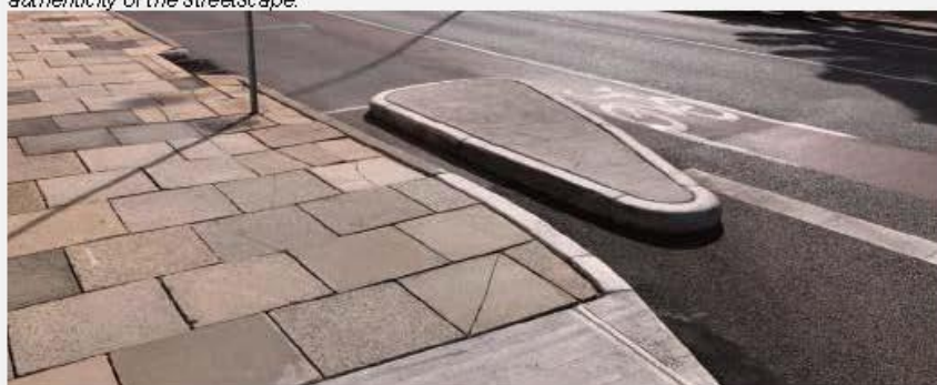
Important details: historic slabs should be kept and maintained. Blobs of concrete as added in the street here and covered in graffiti undermine the traditional linearity of the historic streets.
