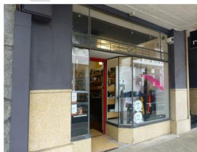
Inter-War Era shopfront. Note fine timber frame with metal cladding and timber door in timber frame. Also note terrazzo dado to piers, terrazzo threshold, highlight windows and pressed metal lining to awning soffit.
