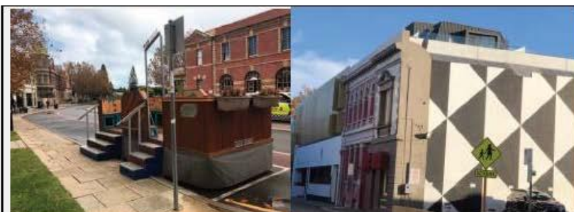
Pop Ups" like this unattractive structure with dead plants, and disrespectful public art on the right have no place in a high quality heritage environment. Note the recent modern grey rooftop additions which further reduce the authenticity of the streetscape.
