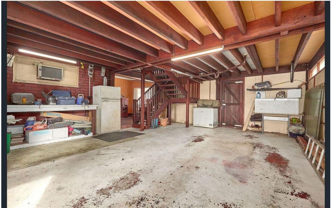
Figure 1: Interior of dwelling showing removed side wall.
