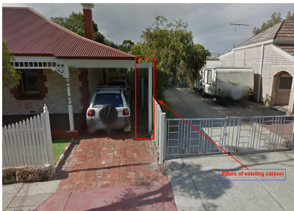
Image 3: Carport including posts located on the boundary of adjoining property at 4 Commercial Street.
