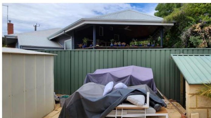
View Illustrating patio deck rail over existing 2100 fence height.
