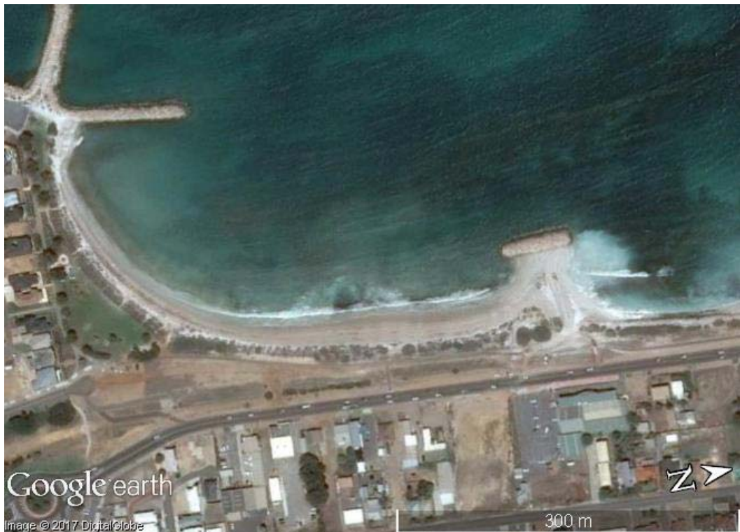
Figure 4-4 Detached breakwater (bottom right) forming a tombolo in Geraldton, Western Australia, as part of a coastal protection and harbour configuration (Source: Google Earth Pro)
