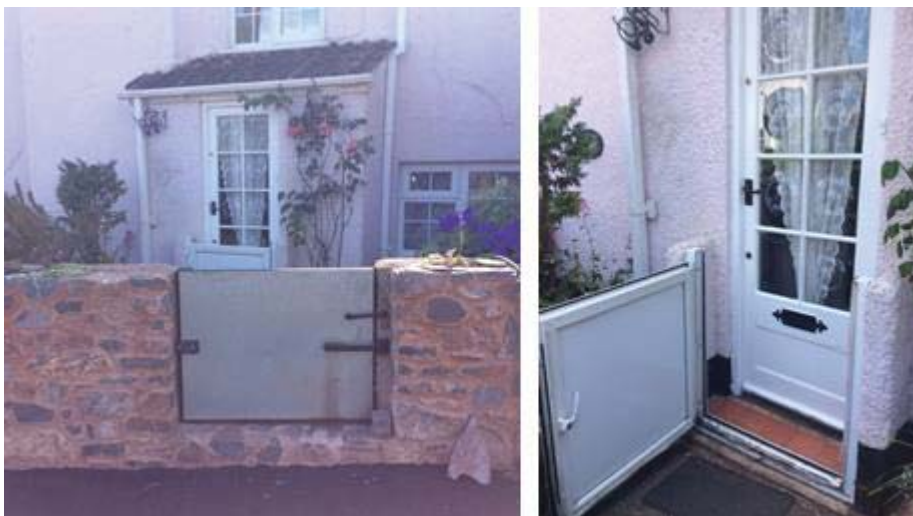
Figure 4-10 An example of retrospective design requirements: flood wall/gates and doors added to a dwelling to protect existing property from storm related flooding in United Kingdom
