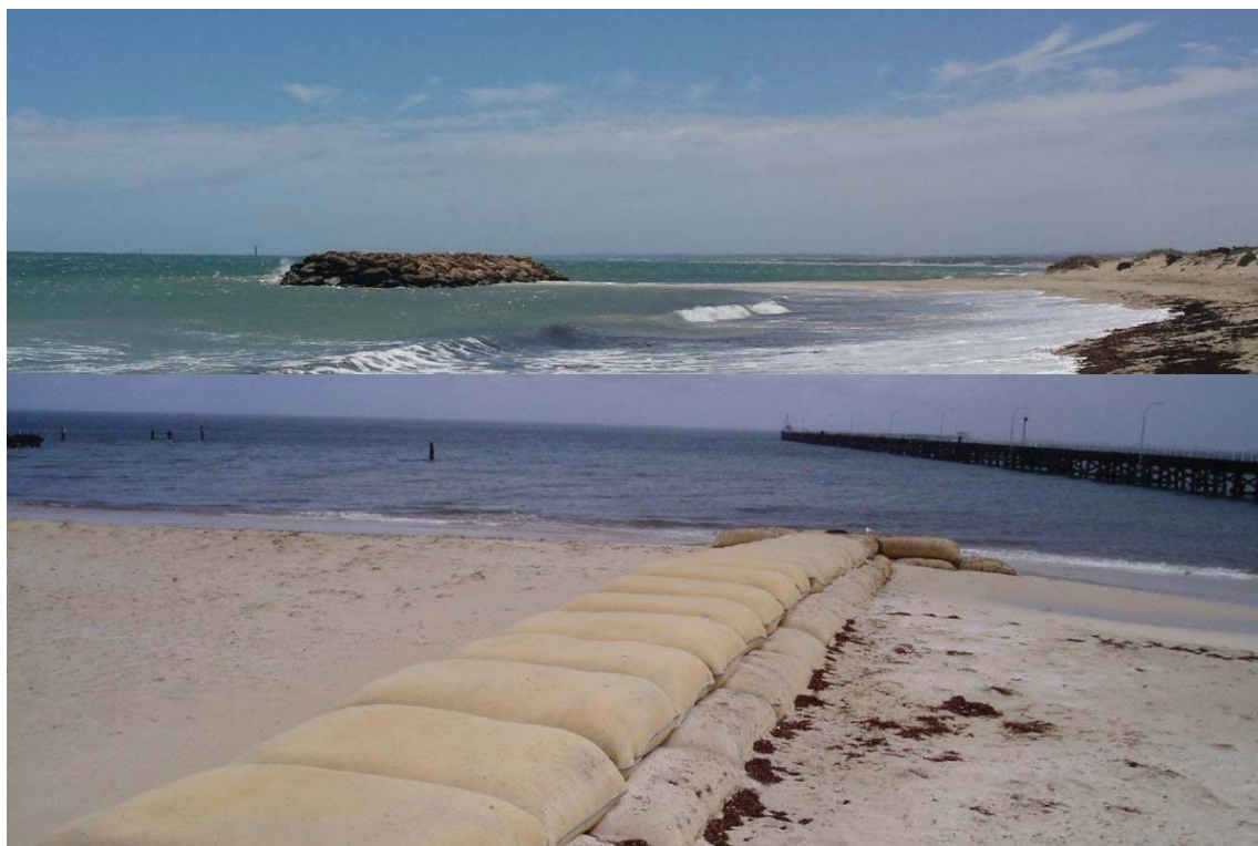
Figure 2-2 Top: offshore breakwater. Bottom: geotextile sand container groyne.
