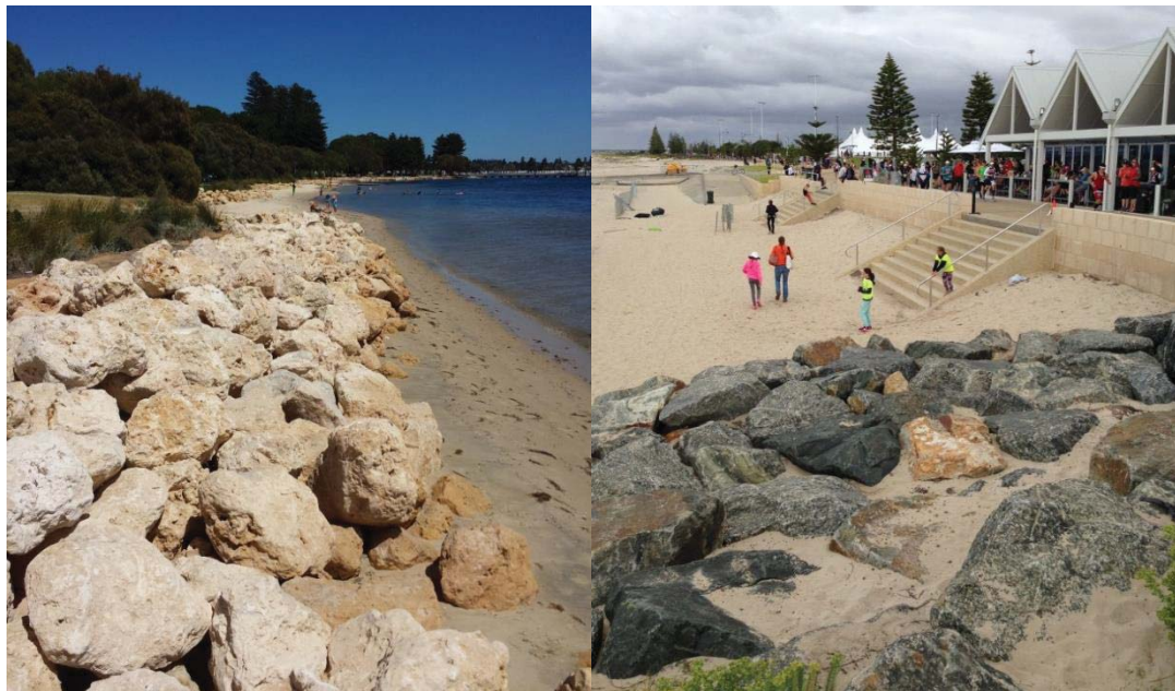
Figure 2-3 Limestone rock seawall left and block work retaining seawall right.
